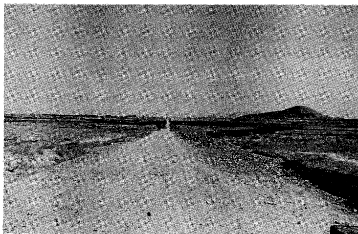
Kilometer 12.8 west of Rezaiyeh. Selected material is dumped in piles on one side of roadbed and gradually spread by hand. Virtually one-way traffic is required for months by this operation.
