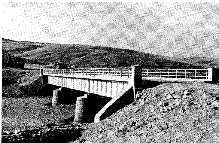
Kilometer 81.3 north of Bijar Junction. Newly constructed steel plate girder bridge with concrete deck. Three 22-meter spans, 5.5-meter roadway with two 0.75-meter sidewalks.
