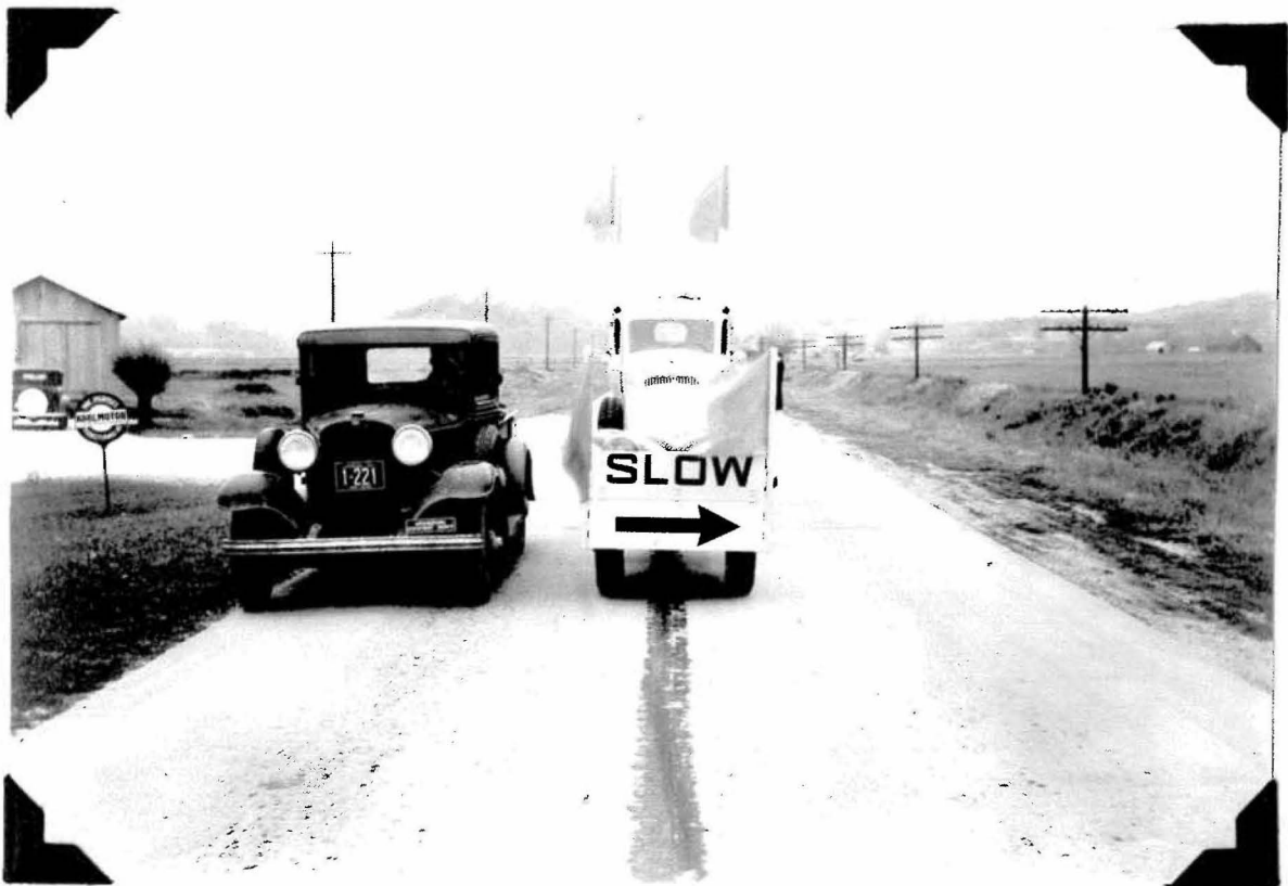
Front view of center line striping machine showing narrow gauge. Note flags and signs for safety.
