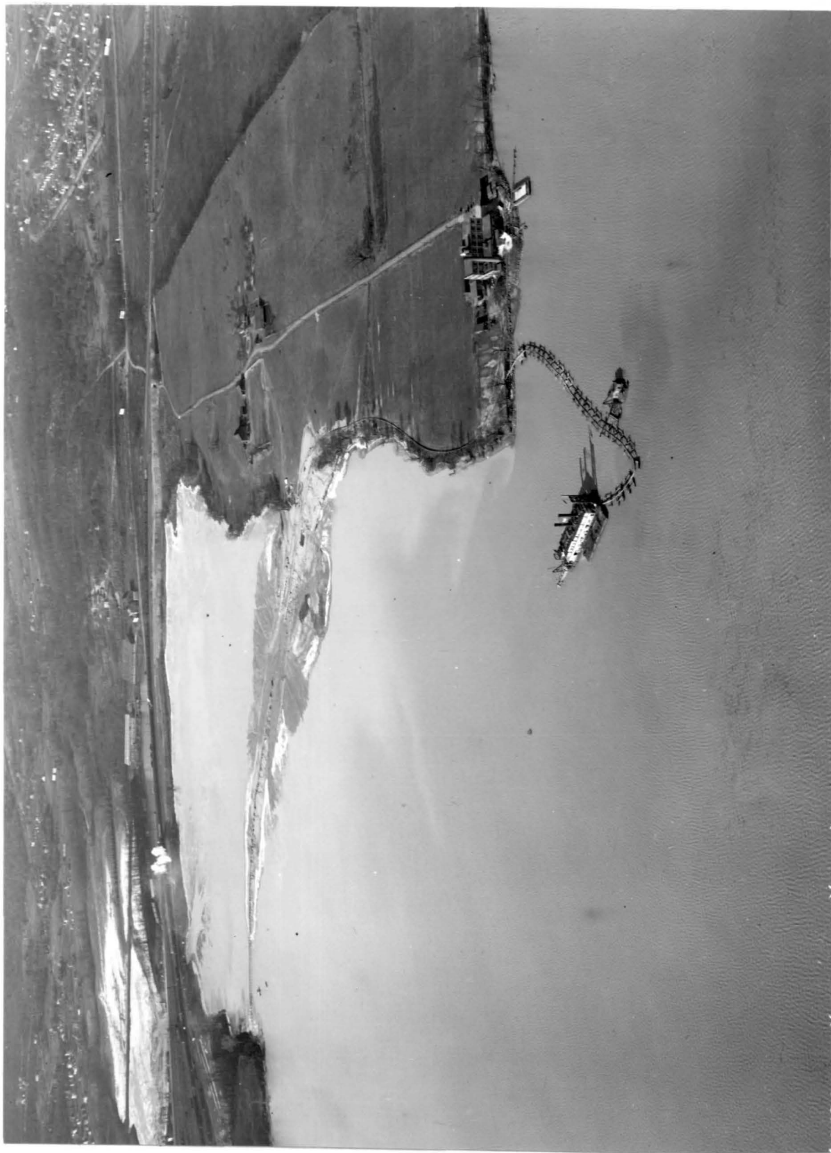
Hydraulic Fill - Four Mile Run.
