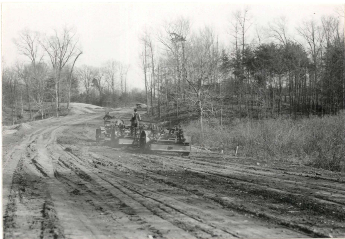
No. 528. Finishing Earth Graded Road
