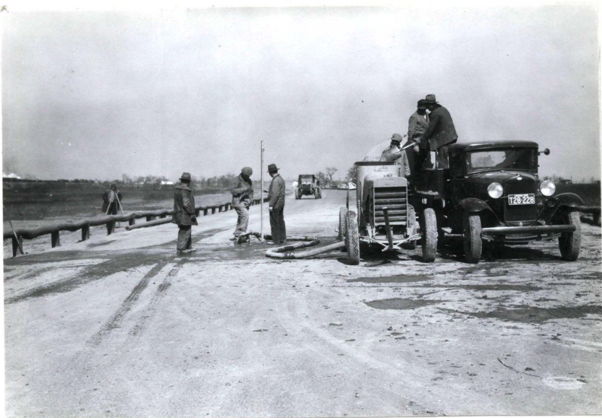
No.715. Checking Grade with Mud Jack in Operation
