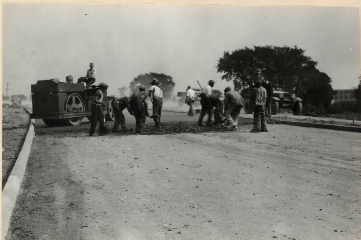
No. 20. Spreading Asphaltic Concrete Surface Course about Station 174.
