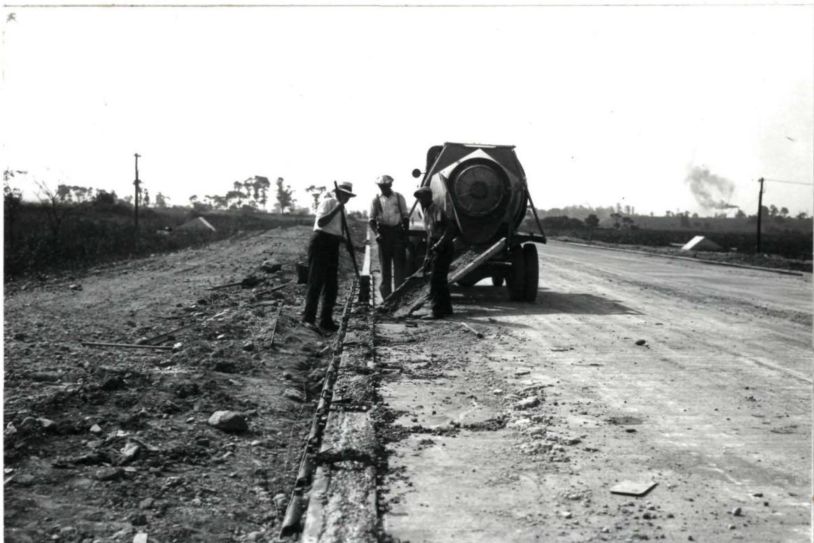
Building Concrete Curb About Station 250
