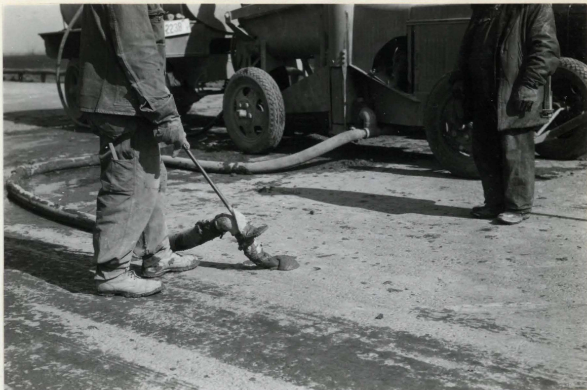
No. 653. Raising Pavement, using Mud-Jack.
