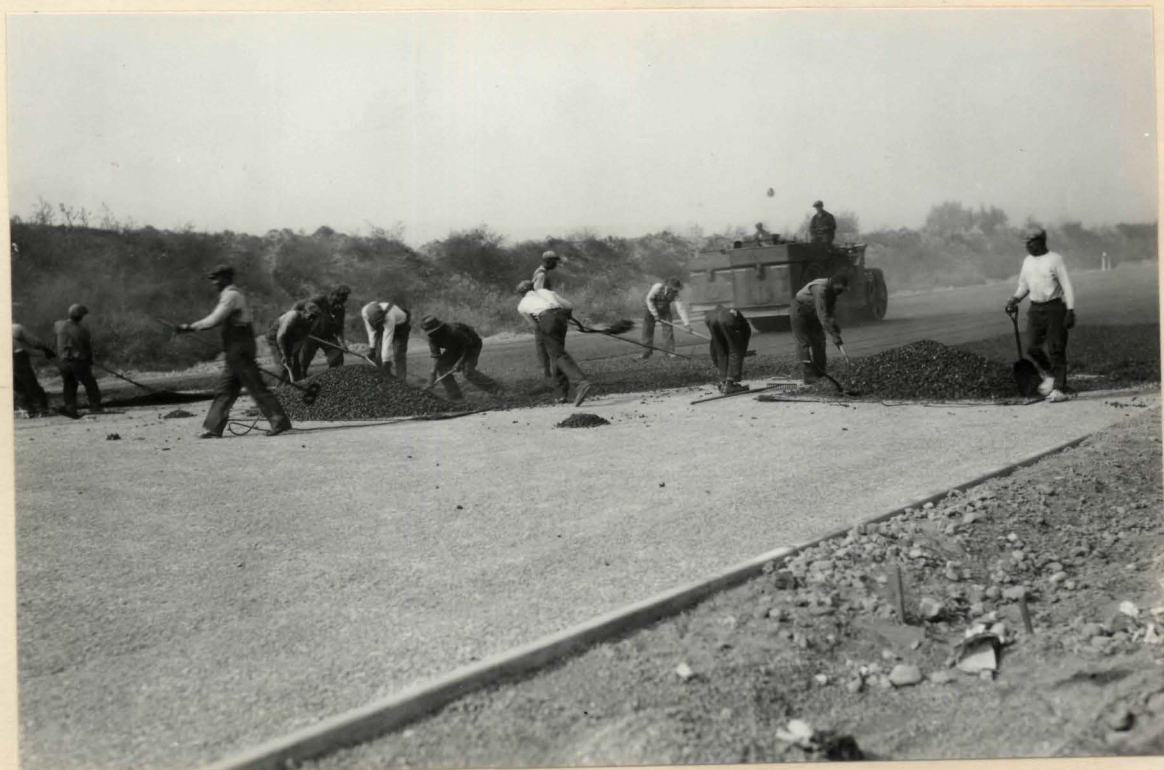
No. 1. Spreading Asphaltic Concrete Surface Course about Station 41 - Columbia Island.
