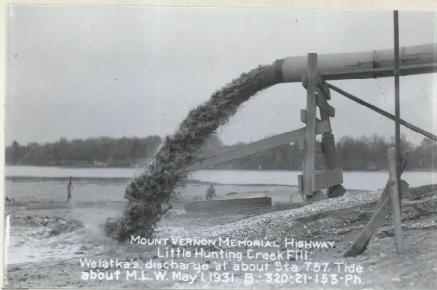
Hydraulic Fill, End of Discharge Pipe
