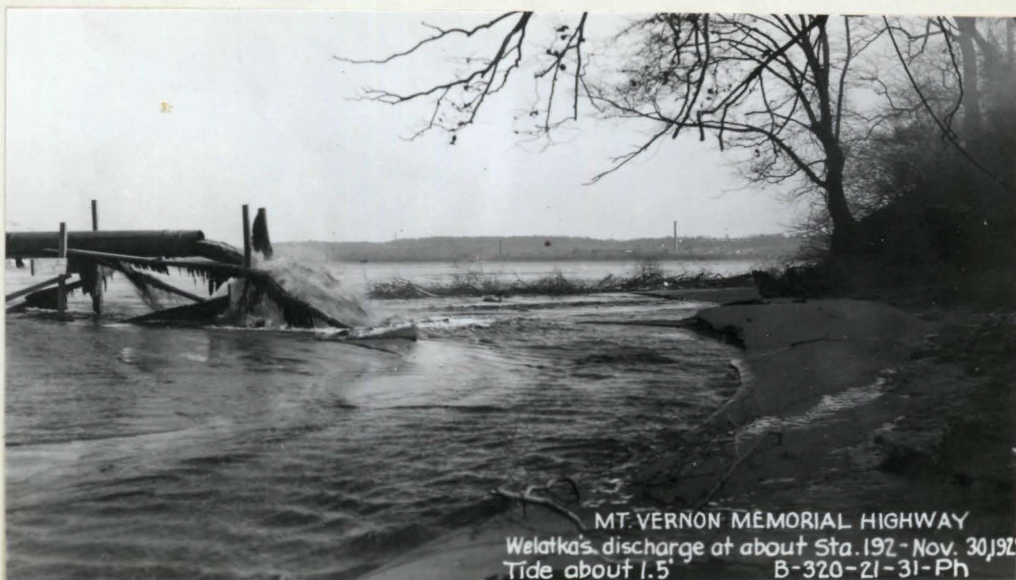
Four Mile Run, South Side, End of Discharge Pipe
