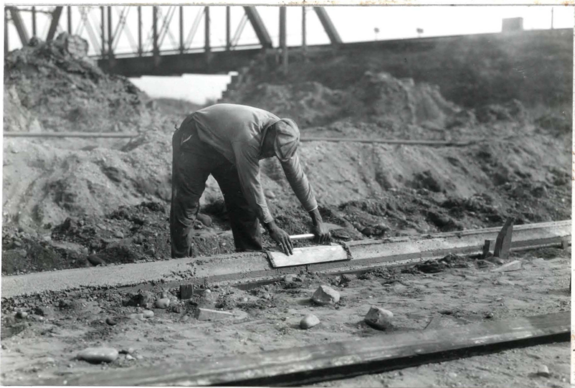
Finishing Concrete Curb About Station 71
