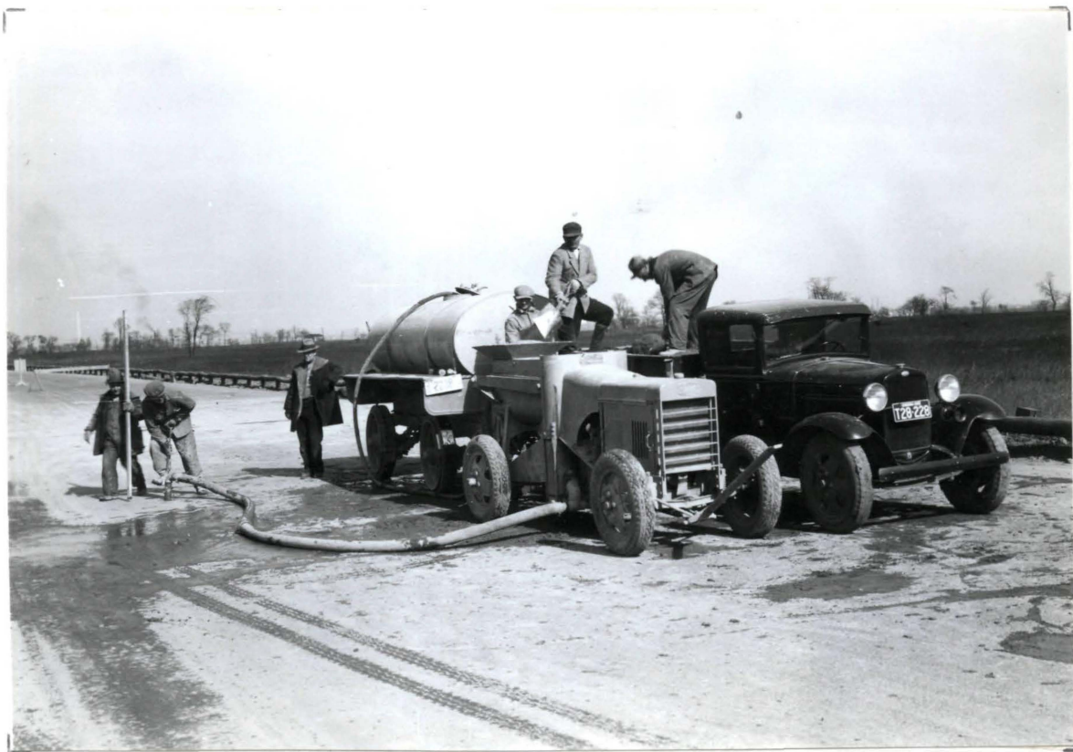
No.651. Checking Grade with Mud Jack in Operation
