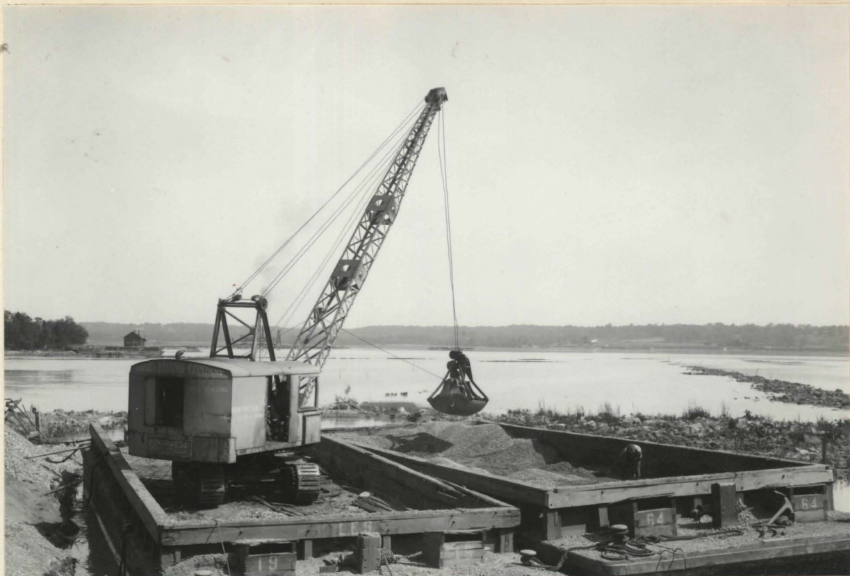
No. 134. Unloading Barges to Batching Plant, Little Hunting Creek
