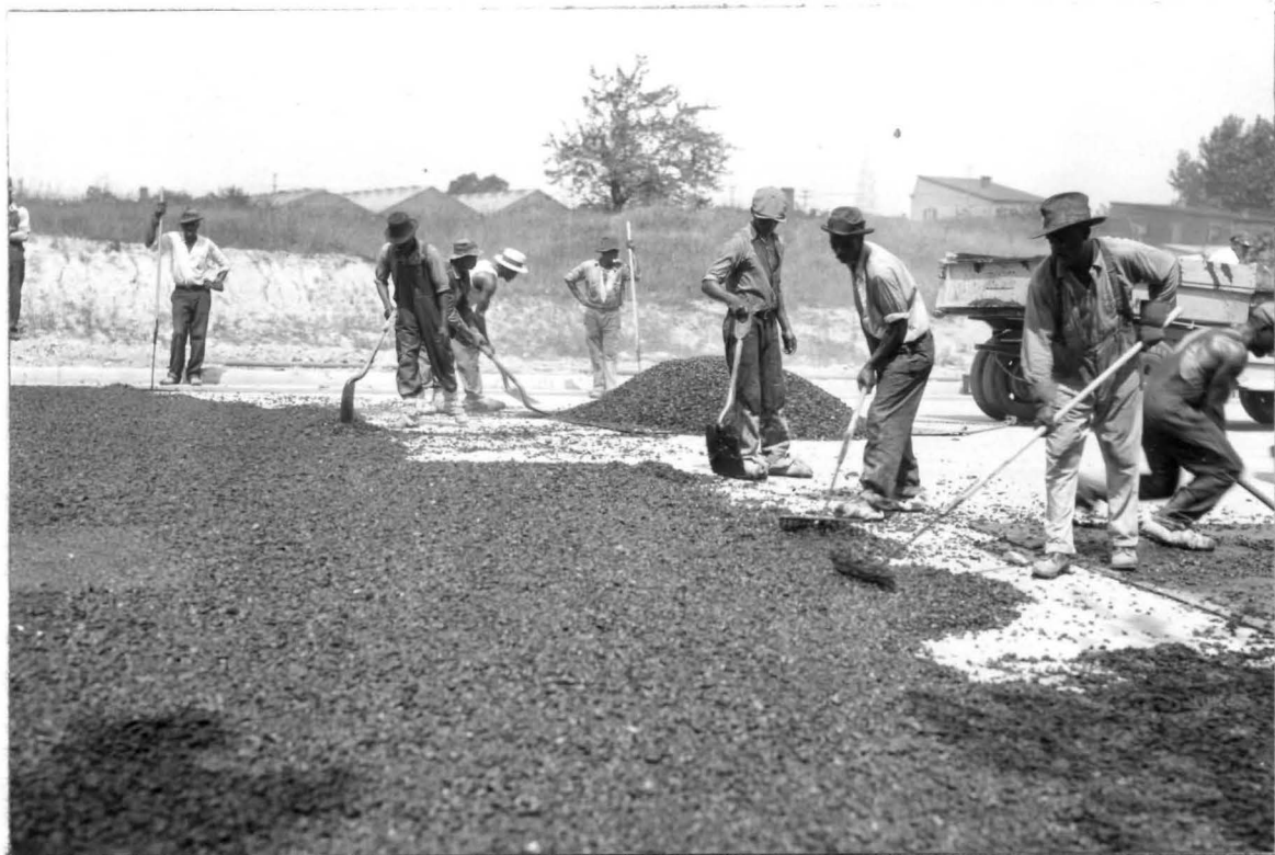
Spreading Asphalt Binder
