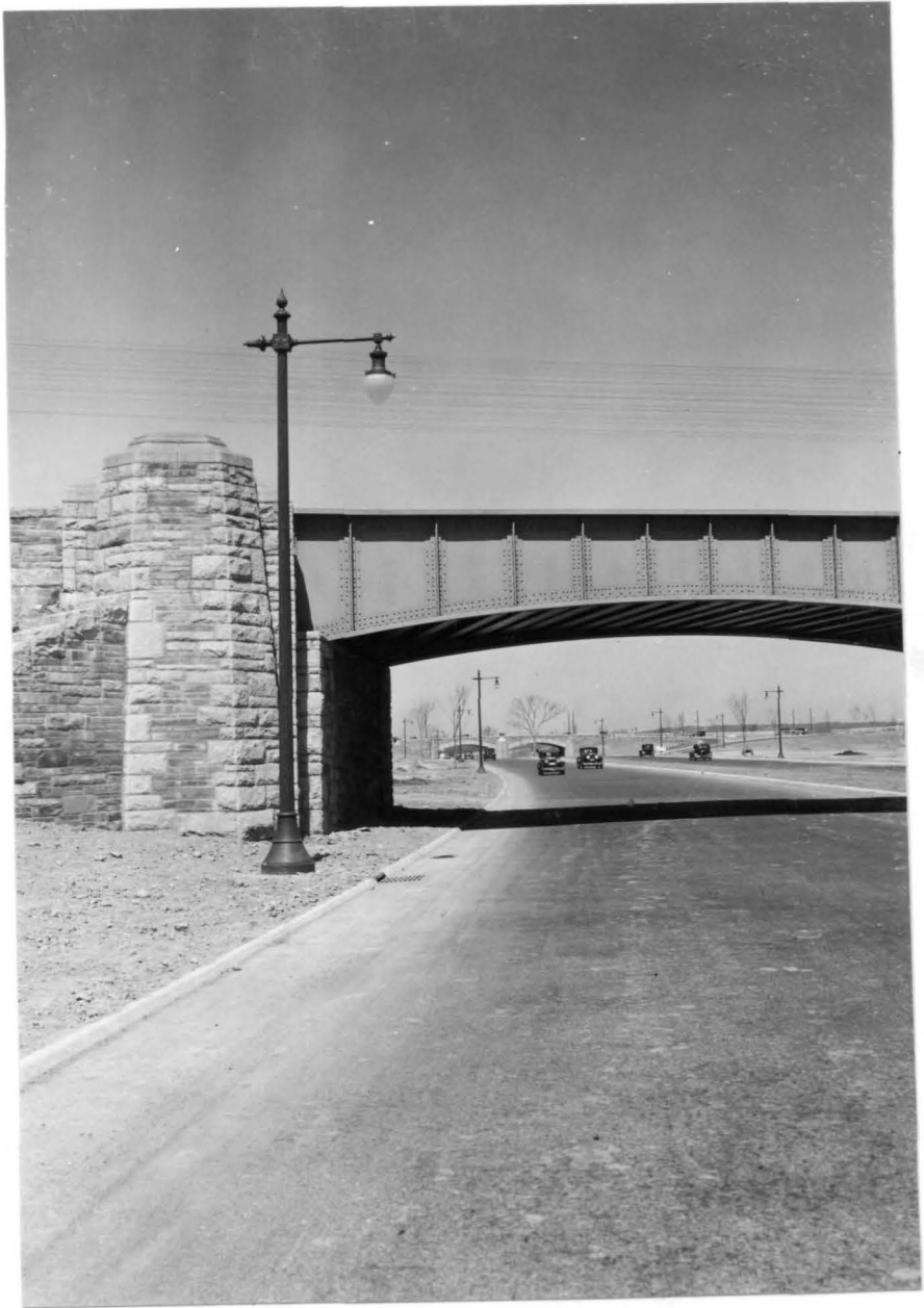
No. 1088 Single Metal Standard near R. F. & P. R. R. Underpass.
