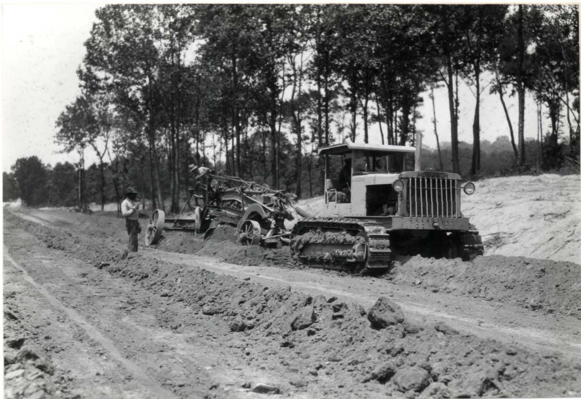
No. 528. Finishing Earth Graded Road
