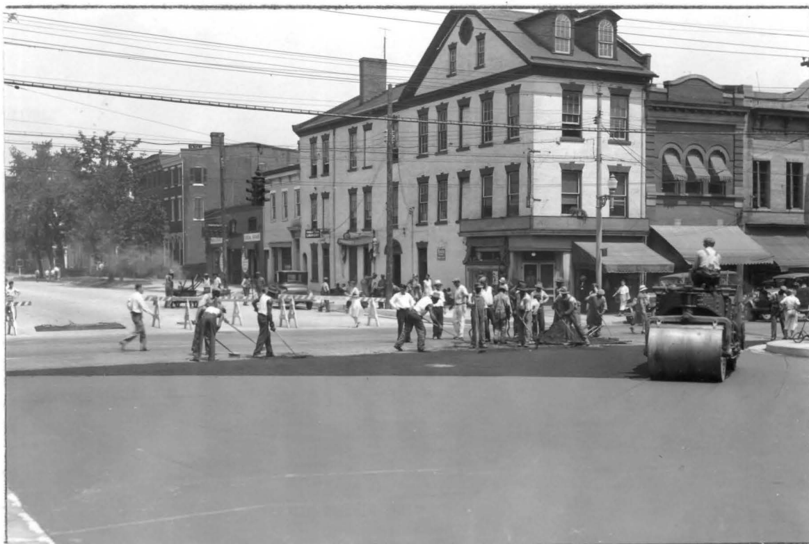
Washington and King Streets Intersection Spreading and Rolling Asphalt
