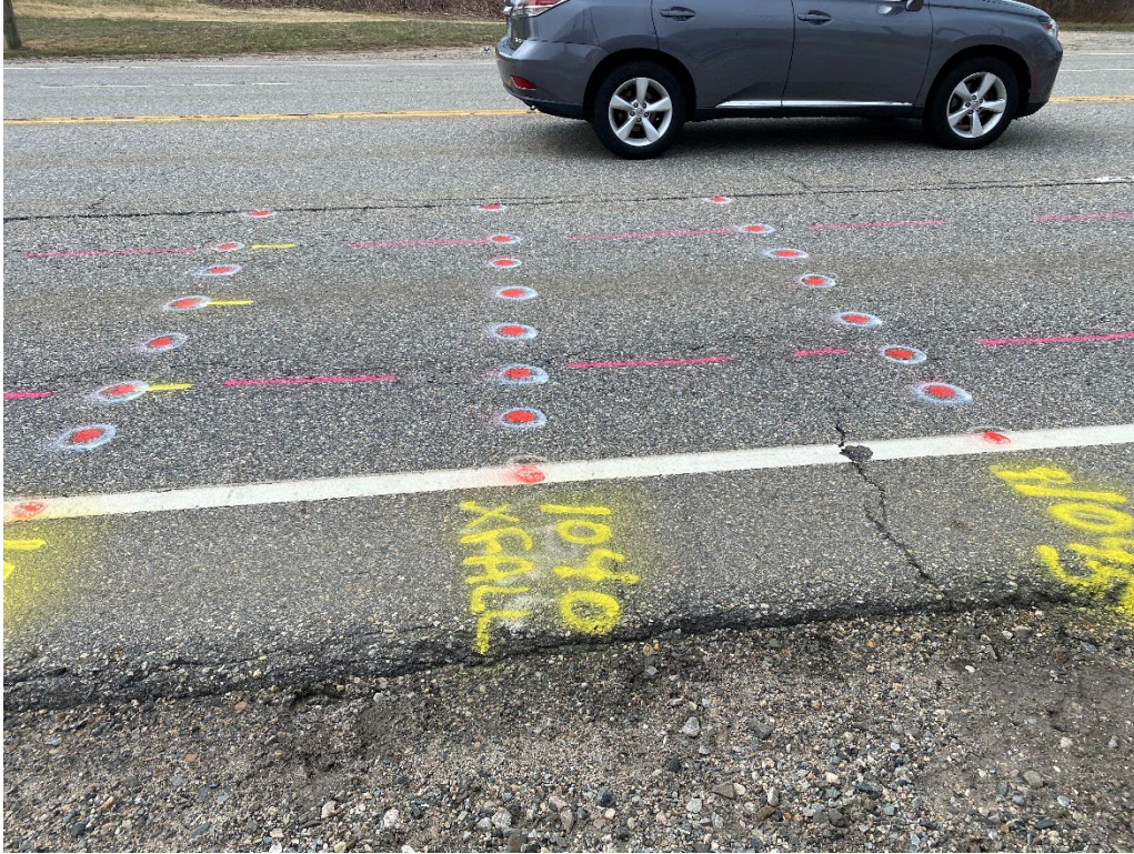
Figure 15. Photo. Marking of CTDOT Site for Transverse Profile Validation
