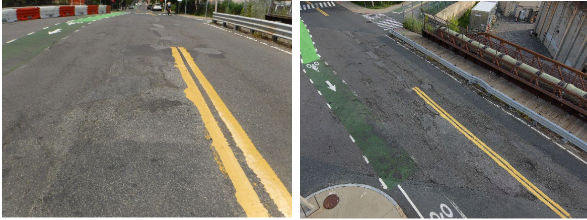
Figure 43 - Terrestrial versus Aerial Image of Wearing Surface
