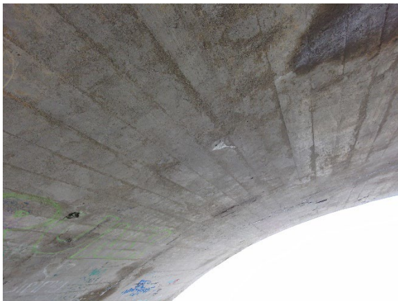
Figure 47 - Underside of Concrete Arch
