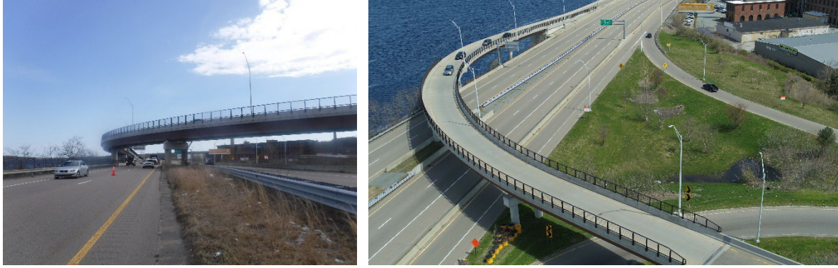
Figure 41 - Terrestrial versus Aerial Elevation of Steel Box Girder Bridge
