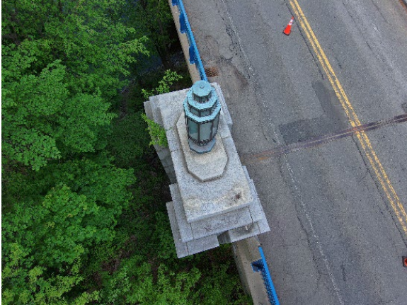
Figure 51 - Top of Pylon
