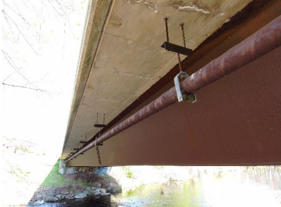
Figure 45 - Underside of Deck Overhang and Girder Web
