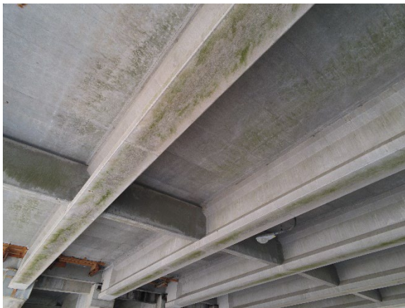
Figure 46 - Underside of Deck
