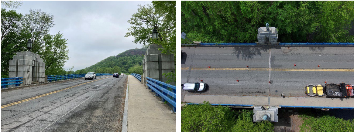
Figure 44 - Terrestrial versus Aerial Image of Wearing Surface
