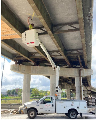
Figure 4 - Inspector Hammer Sounding Deck
