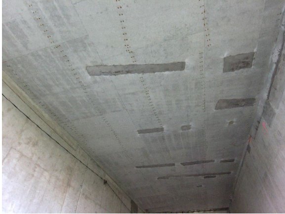
Figure 48 - Underside of Concrete Slab
