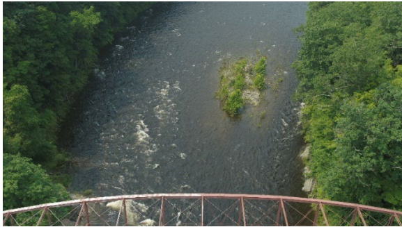
Figure 54 - Aggradation with Vegetation Growth along Channel Upstream of Bridge
