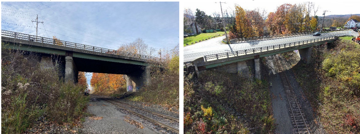
Figure 40 - Terrestrial versus Aerial Elevation of Girder Bridge
