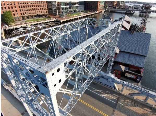
Figure 50 - Counterweight Truss
