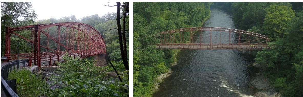
Figure 42 - Terrestrial versus Aerial Elevation of Truss Bridge
