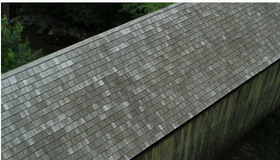
Figure 53 - Roof of Covered Bridge
