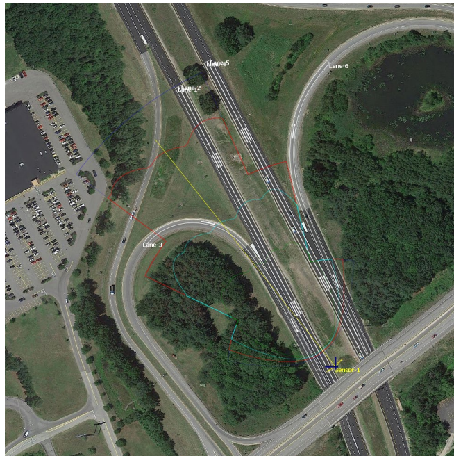
Figure 4-2. Overview of the Tilton North Site
