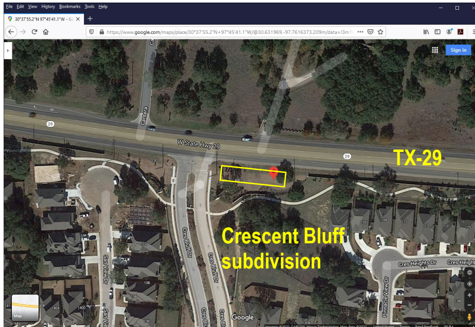
Figure 4.1: Aerial view of the Georgetown (GTWN) field experiment site; the yellow rectangle is the ground surface trace of the probed volume.
