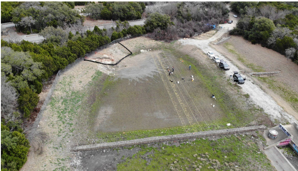
Figure 4.43: Drone view of deployed ERT lines A-D.
