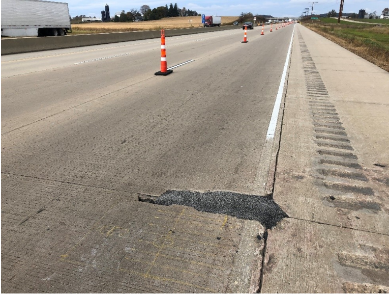
Figure 7.2 Photo. Small corner break fully patched with asphalt observed on I-39 NB in Dane County, Wisconsin.
