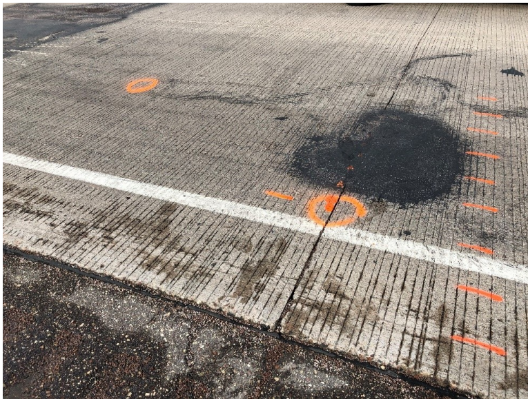
Figure 7.19 Photo. Large spall with asphalt patch and on US 53 in Eau Claire County, WI.
