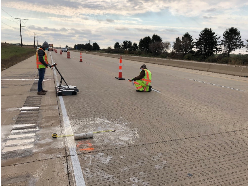
Figure 12.1 Photo. Collecting dowel alignment data using pulse induction on I-39 NB in Dane County, Wisconsin.
