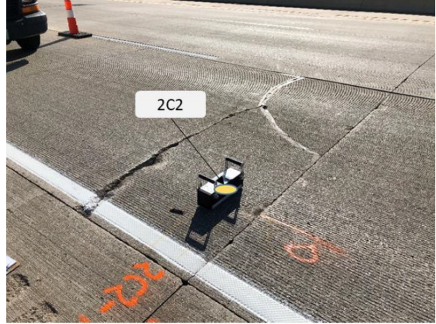
Figure 10.20 Photo and Illustration. Location of core on I-39 NB in Columbia County, Wisconsin, near a cracked slab exhibiting a transverse crack and a corner break.
