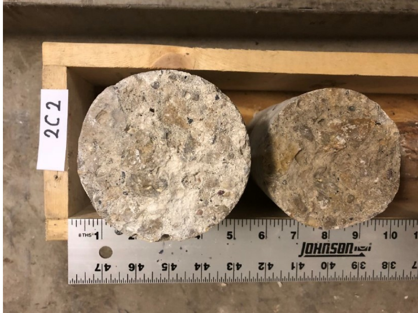
Figure 10.22 Photo. Cross section of 2C2 core from I-39 NB in Columbia County, WI.
