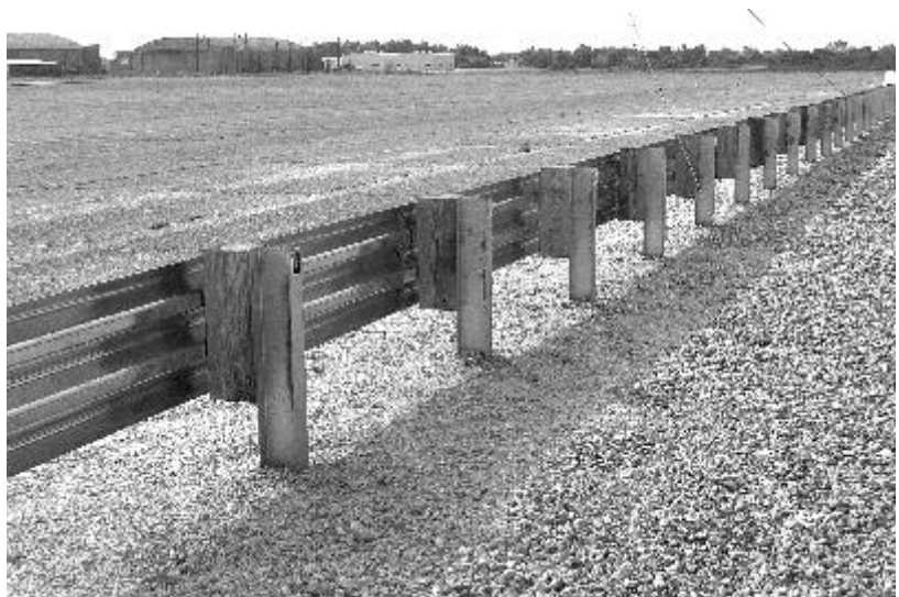
Figure 62. Thrie beam guardrail installation prior to test 404211-10.
