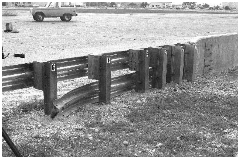
Figure 25. Vertical wall transition prior to test 404211-12.
