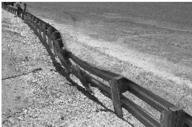
Figure 10. Installation after test 404211-13.
