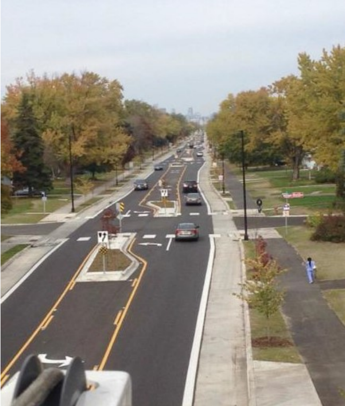
Figure 2 After Conversion in Richfield, Minnesota (Source: Minnesota Department of Transportation)
