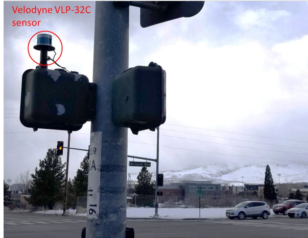
Figure 3-4. The roadside LiDAR sensor for data acquisition.
