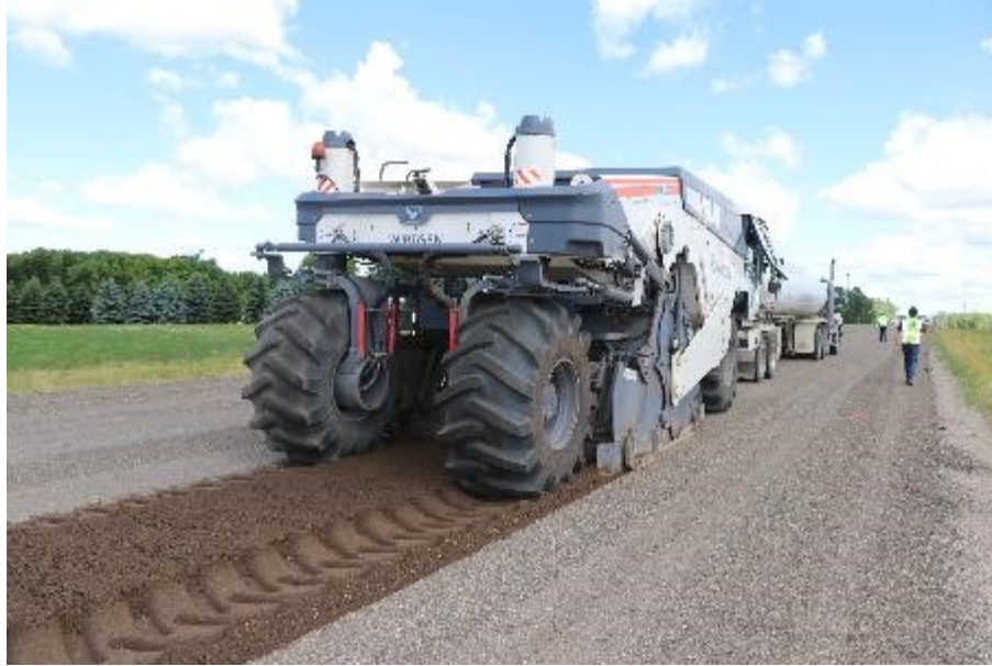
Figure 42. Milling top 8-inch RAP base aggregates using a reclaimer
