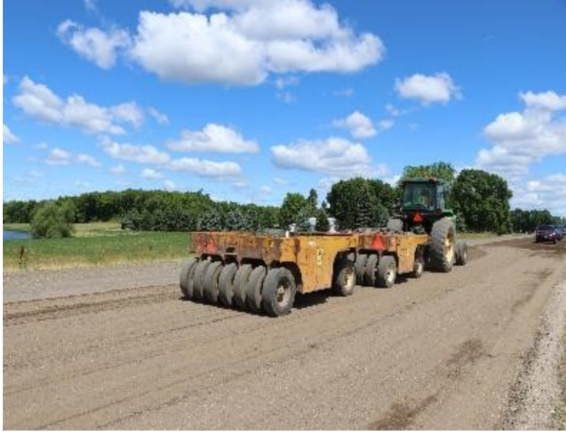
Figure 47. Rubber-tire rolling compaction by using customized weighted vehicle
