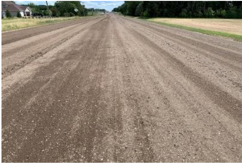
Figure 48. FDR base right after compaction
