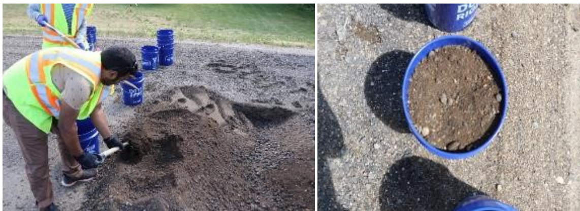
Figure 77. Collecting FDR base material from field demonstration site CSAH-14 highway
