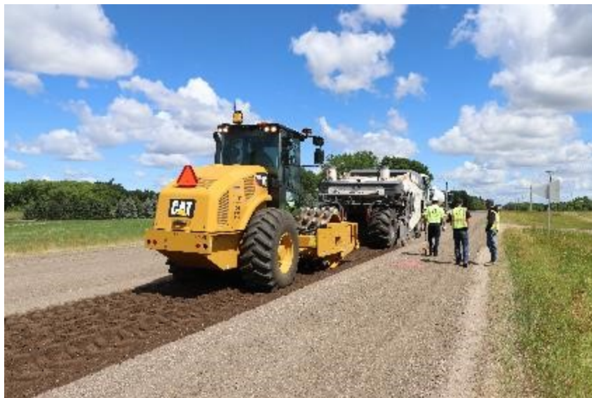
Figure 45. Sheep-foot rolling right after mixing stabilizer with FDR material
