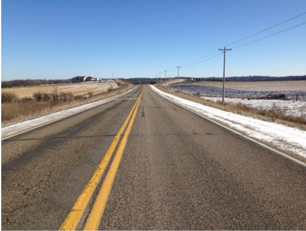
Figure 2.5 Olmsted County Road 117 (Station 105+00) 11/25/2014
