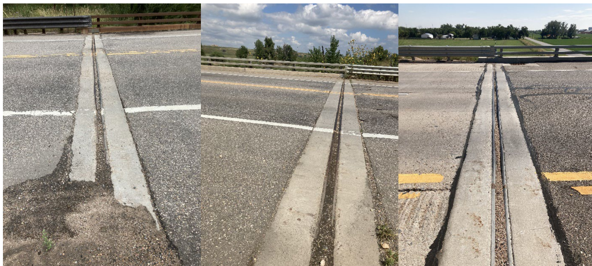
Figure 5-6 Clogged joints observed on multiple bridges within this study
