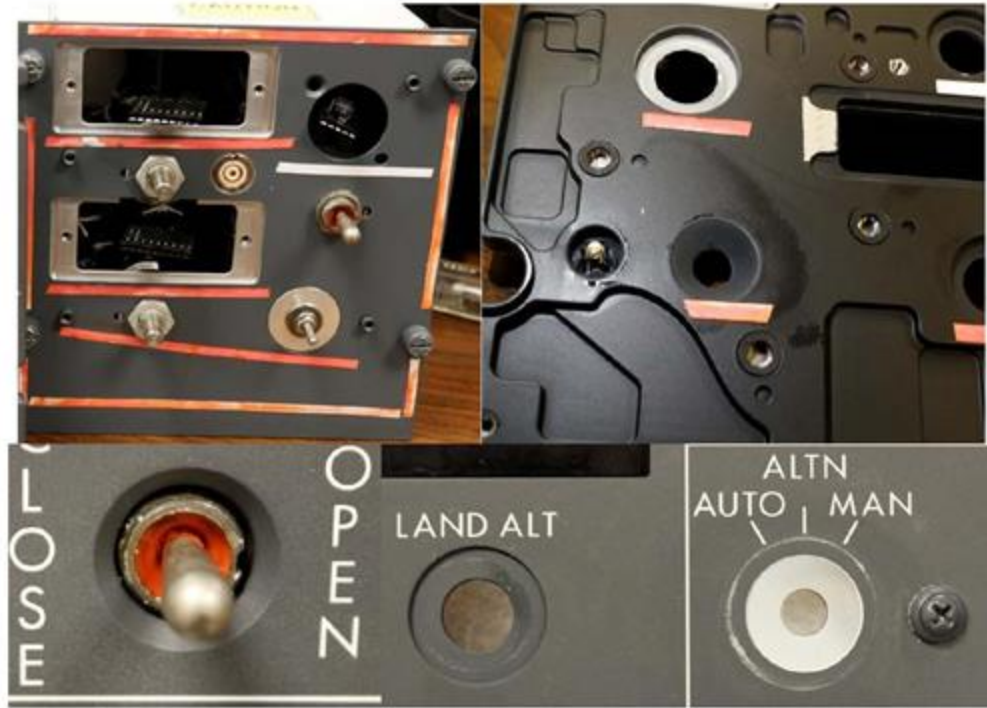
Figure 24: Indications of ingress and residue build up on cabin pressure selector panel
