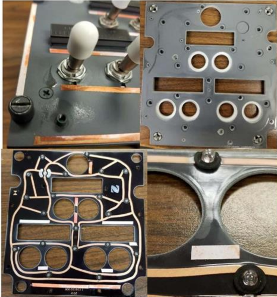
Figure 25: Indications of ingress on fuel control panel and degradation of conformal coating on circuit board
