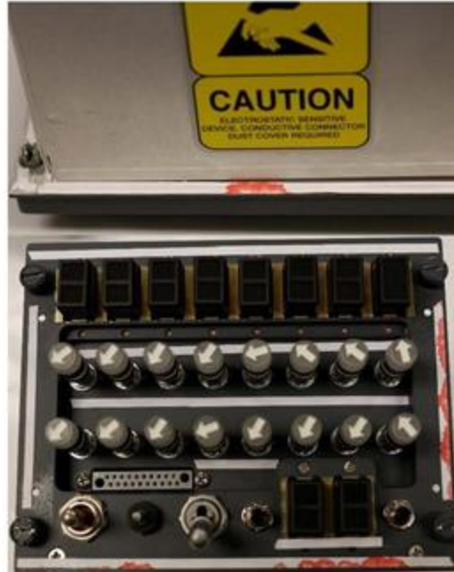
Figure 9: Indications of ingress after set of 2 applications on pressure selector panel (top) and ACP (bottom)
