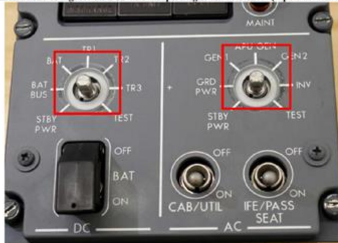
Figure 16: Calla 1452 residue build up behind knobs of P5-13 panel
