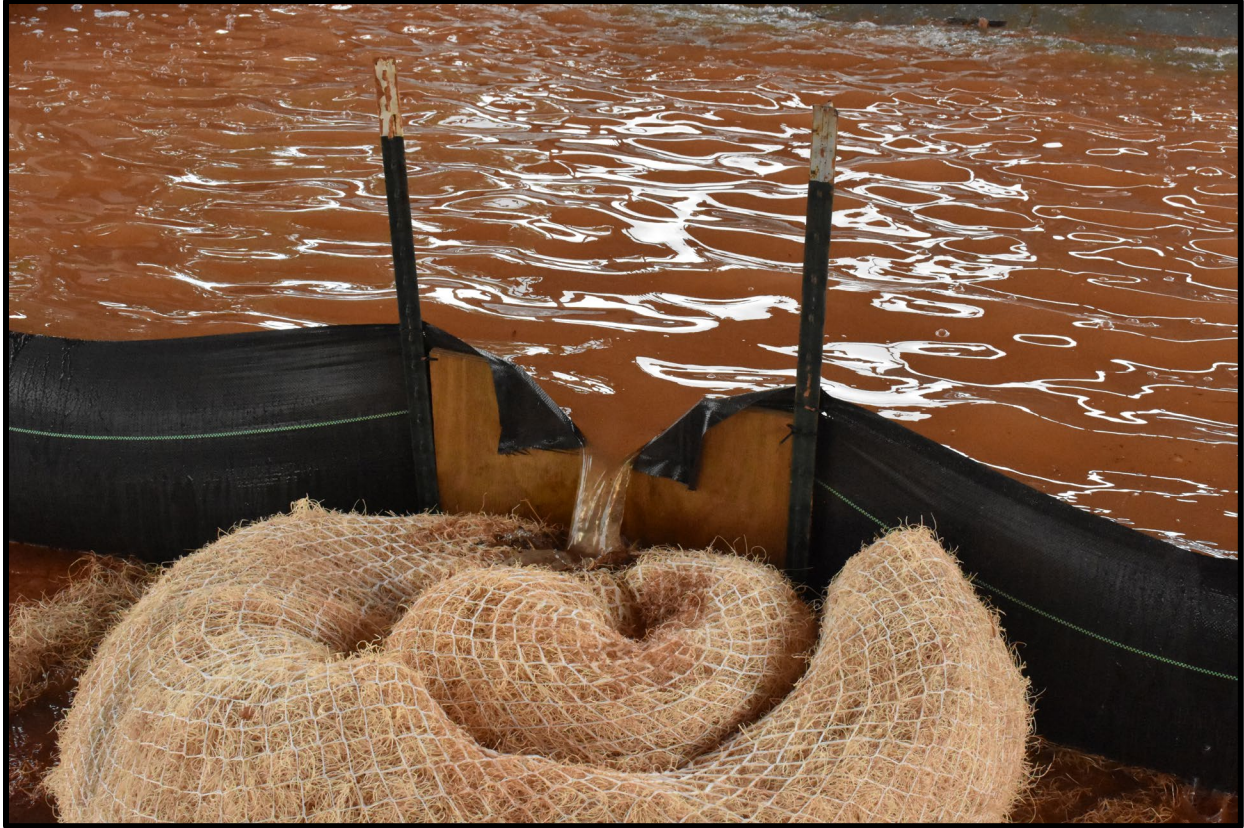
Figure 3.16 Overflow Weir Dewatering
