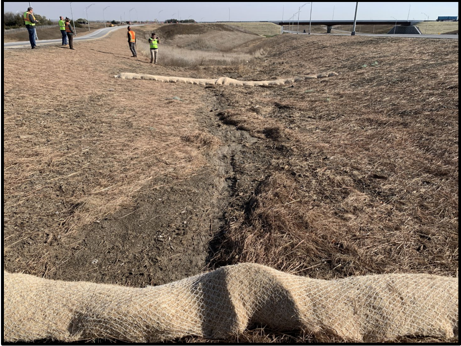
(b) wattle silt check as ditch protection
