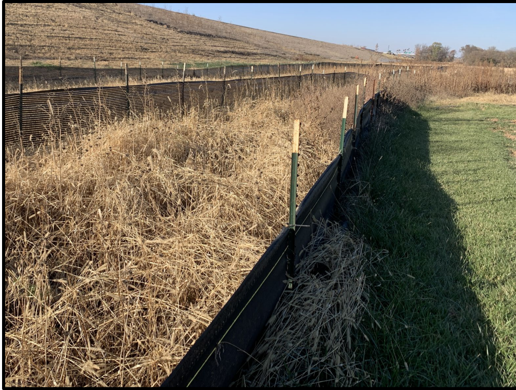
Figure 3.1 Nebraska DOT Silt Fence Installation
