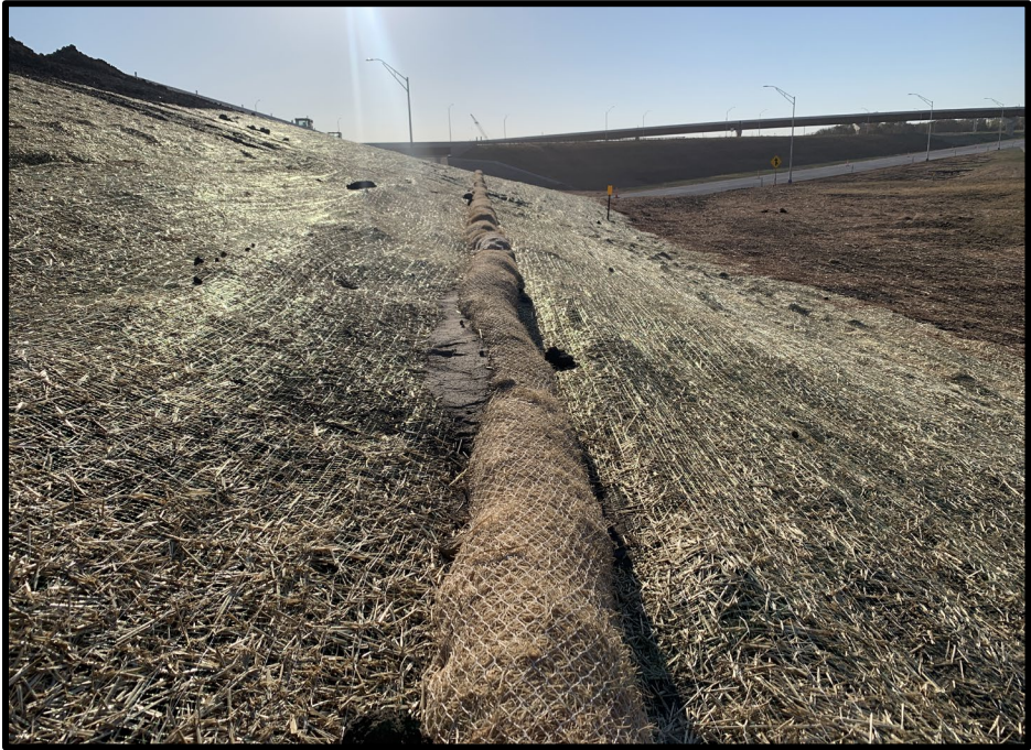
(a) wattle silt check as slope protection
