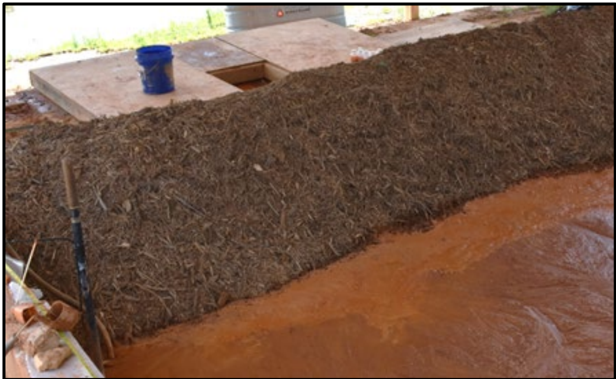
Figure 3.21 Impoundment Formed by Nebraska DOT Slash Mulch Berm Standard
