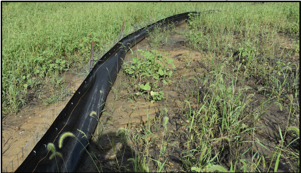
(b) Reinforcement preventing post deflection
