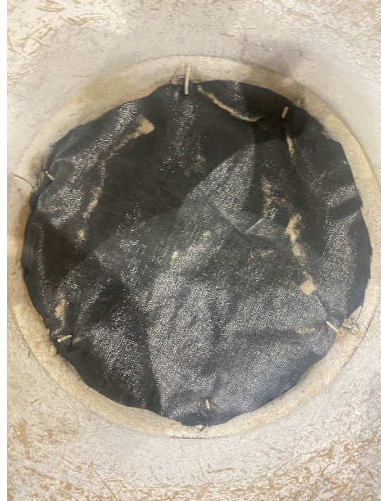
Figure 4.23 500X (GT) geotextile on compacted sand subgrade
