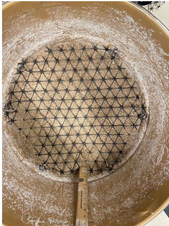
Figure 4.21 TX160 (GG2) geogrid on compacted sand subgrade
