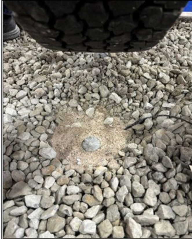
Figure 4.41 Pressure cell installed on top of base course
