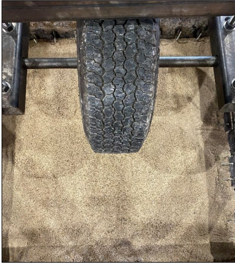
Figure 4.33 Compacted sand subgrade layer
