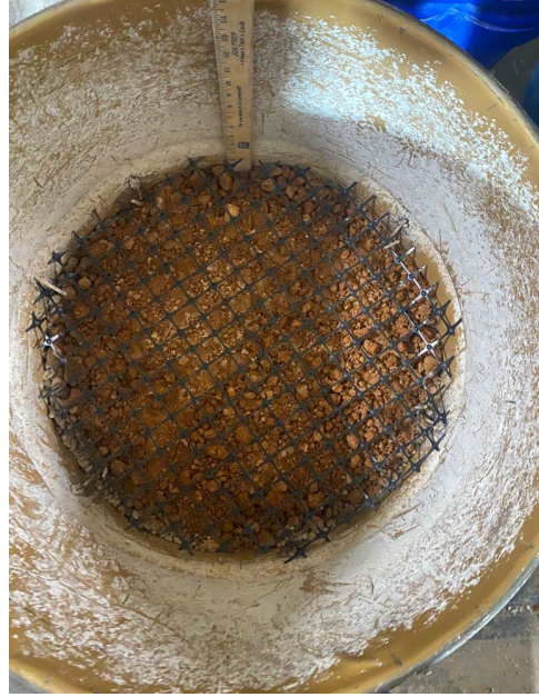
Figure 4.26 Compacted red shale base course layer
