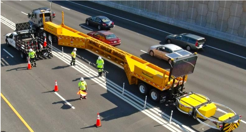
Figure 30. Positive Protection in Work Zones for Protecting Workers
