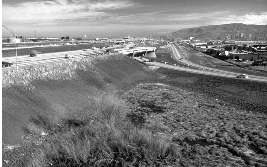
Figure 1-4: Typical highway embankments for improvements and rehabilitation of I-15 Project in Utah. (PB Slide Library)
