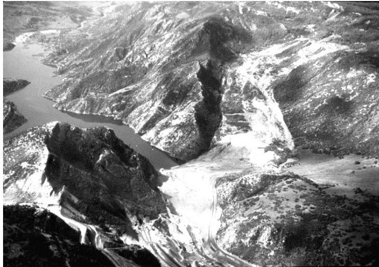
Figure 1-1: Thistle Utah Landslide (U.S. Geological Survey)
