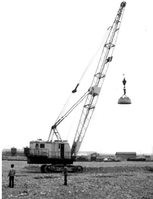
Figure 9-23 Photo Dynamic Compaction at Port of Ningbo, China (Munfakh, 1999)
