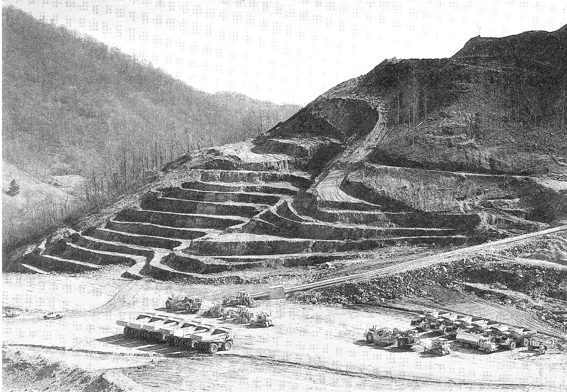
Figure 10-2: Bench Cuts for Interstate 26 Project in North Carolina
