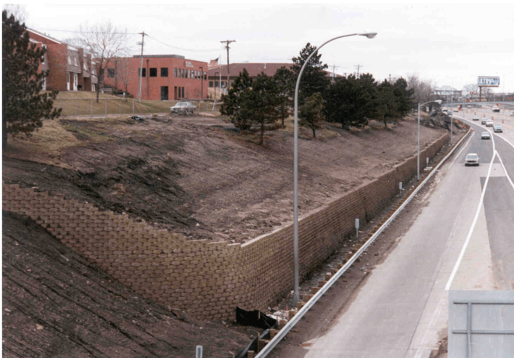
Figure 20. Completed I-94 Wall.
