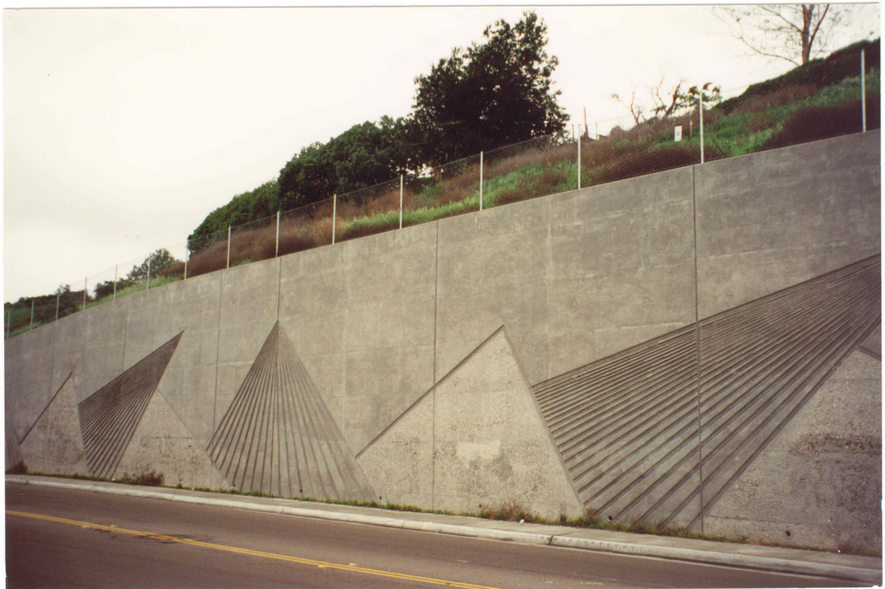
Figure 21. Completed Tonawanda Wall.
