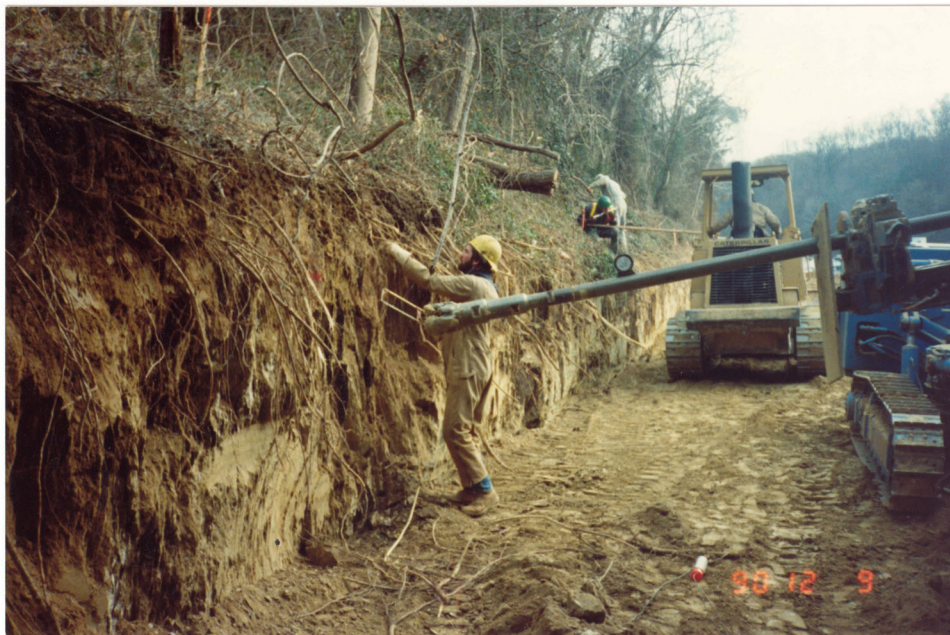
Figure 3. Drilling a Nail Hole.
