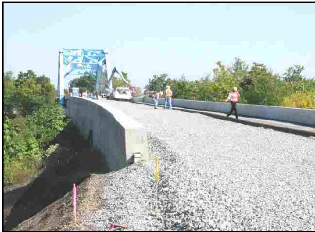
Photograph 4. Completed T-Wall Ramp (Rancocas Bridge in background).
