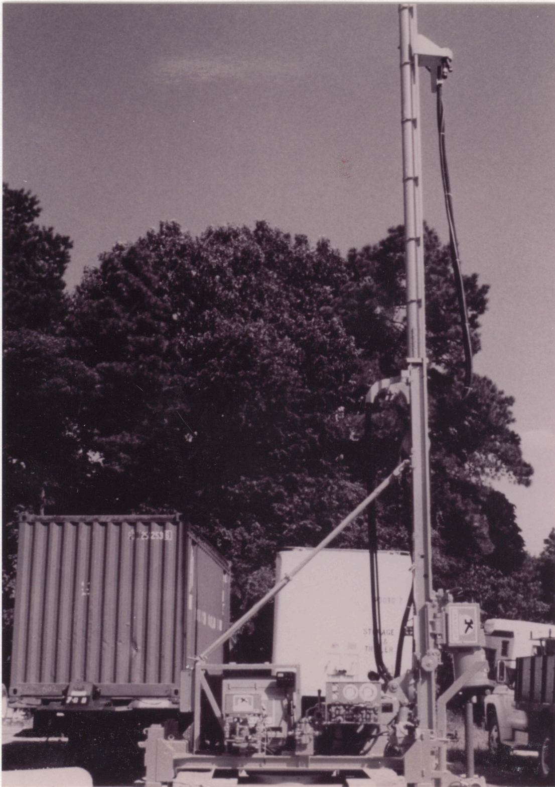
Figure 20. Jet Grouting Rig.
