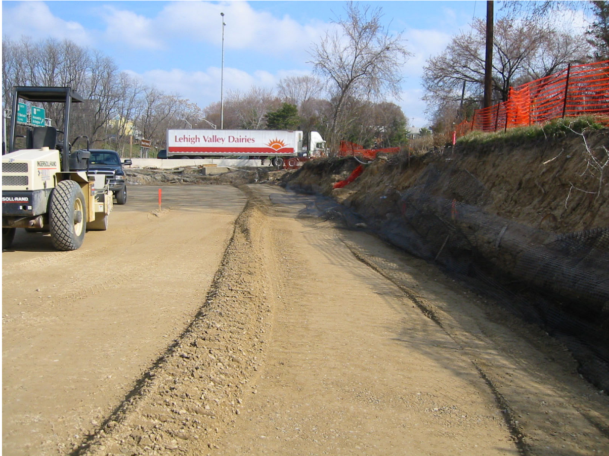
Figure 7. Load Transfer Platform Select Fill Placement.
