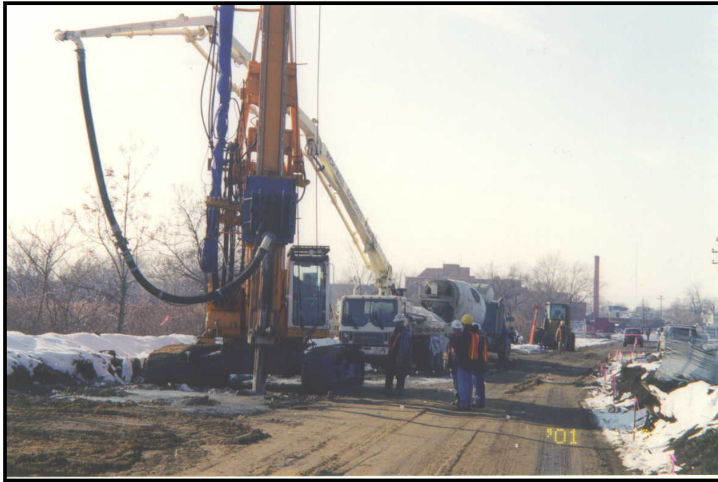
Photograph 1. Vibro-Concrete Column Installation (Vibrator and Concrete Pump).
