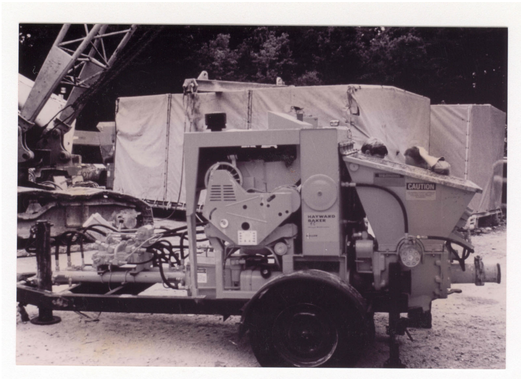
Figure 18. Compaction Grout Pump.
