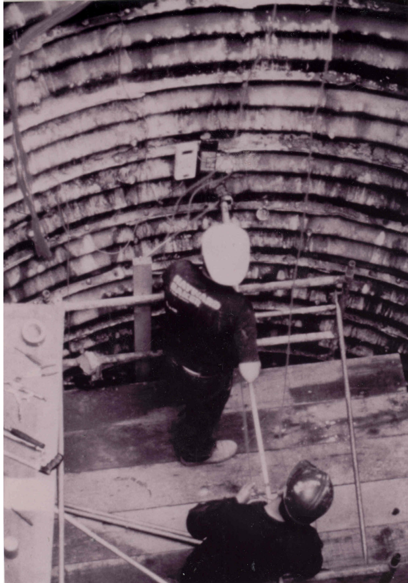
Figure 41. Access Shafts used to Inject Grout.
