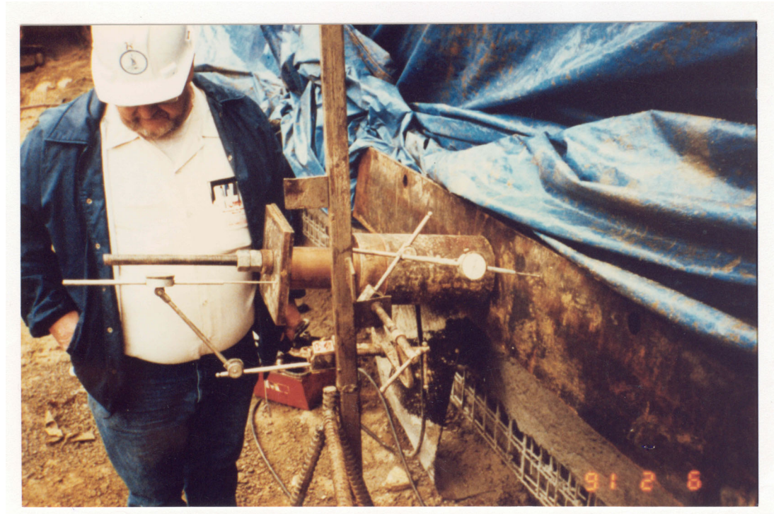
Figure 19. Testing Soil Nails for Capacity.
