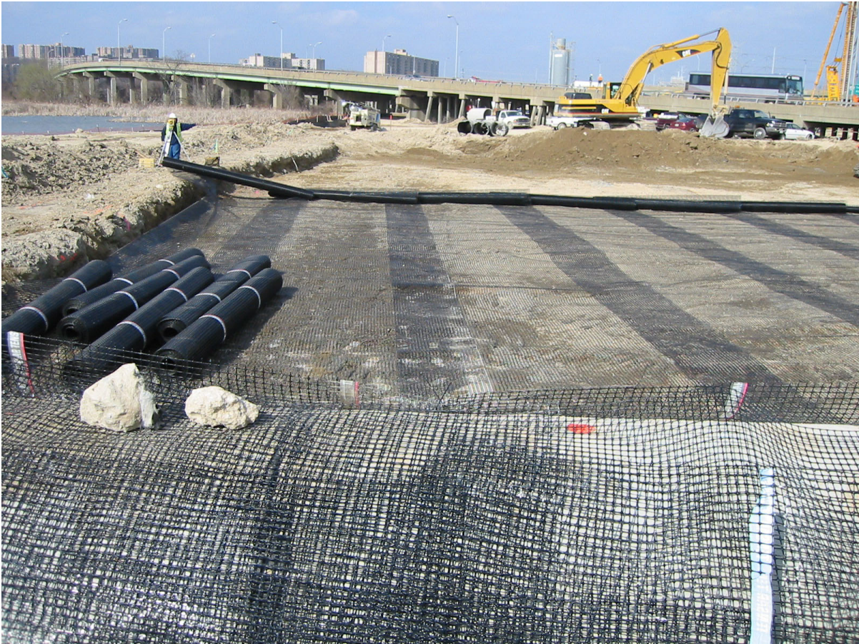
Figure 6. Load Transfer Platform Reinforcement Placement and Compaction.
