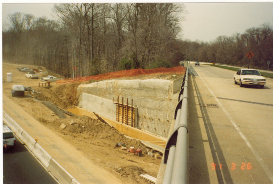
Figure 7. Construction of Cast-in-place Final Facing.
