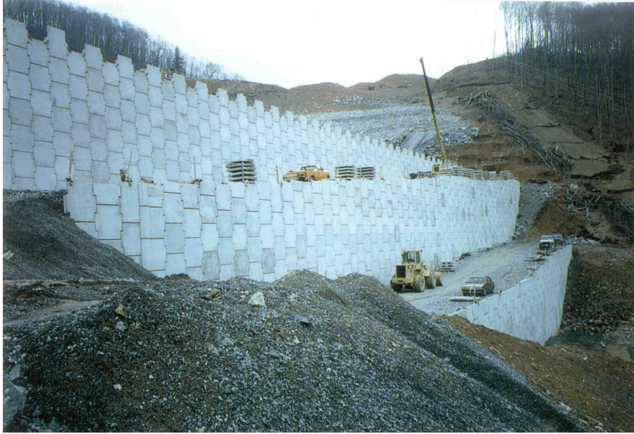
a) During erection
