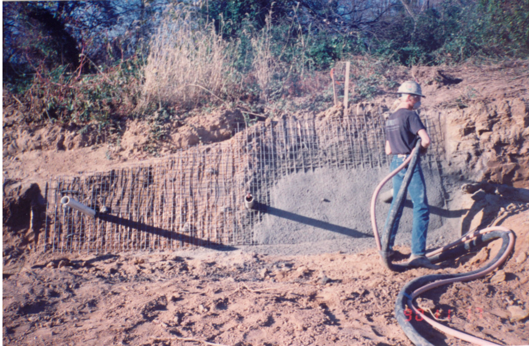
Figure 4. Shotcreting of Face.
