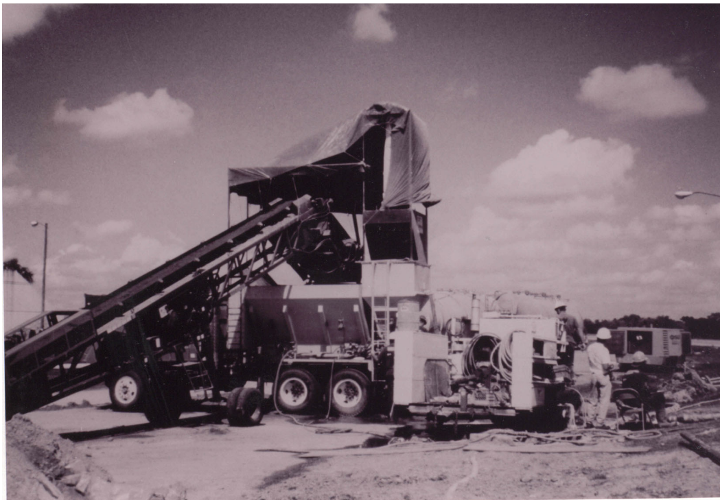
Figure 17. Larger On-Site Grout Batching Plant for Compaction Grouting.
