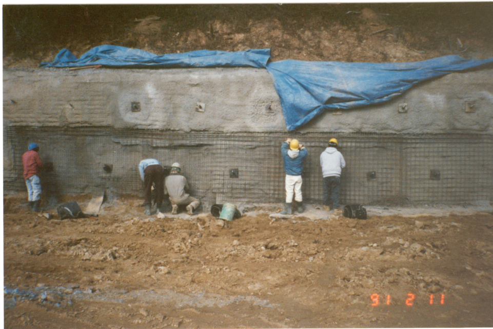
Figure 6. Steel Reinforcement Placement Prior to Second Stage Shotcrete Layer at Facing.
