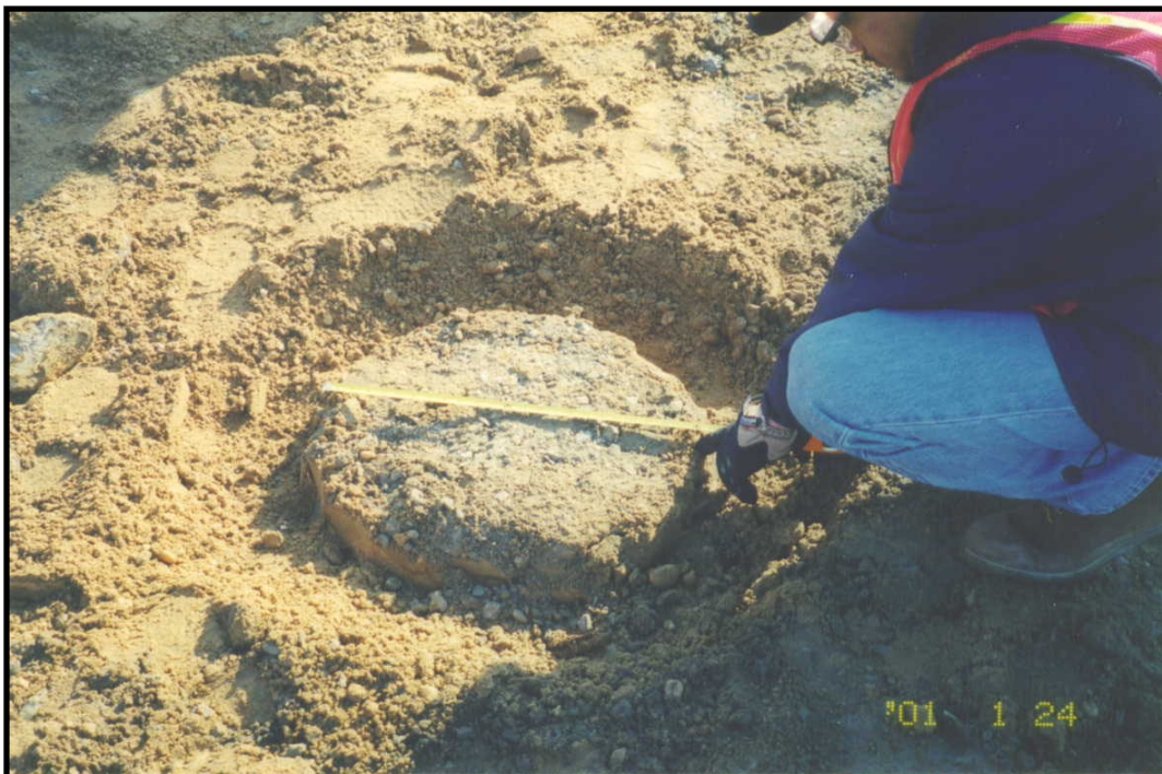
Photograph 2. Top of Finished Vibro-Concrete Column.
