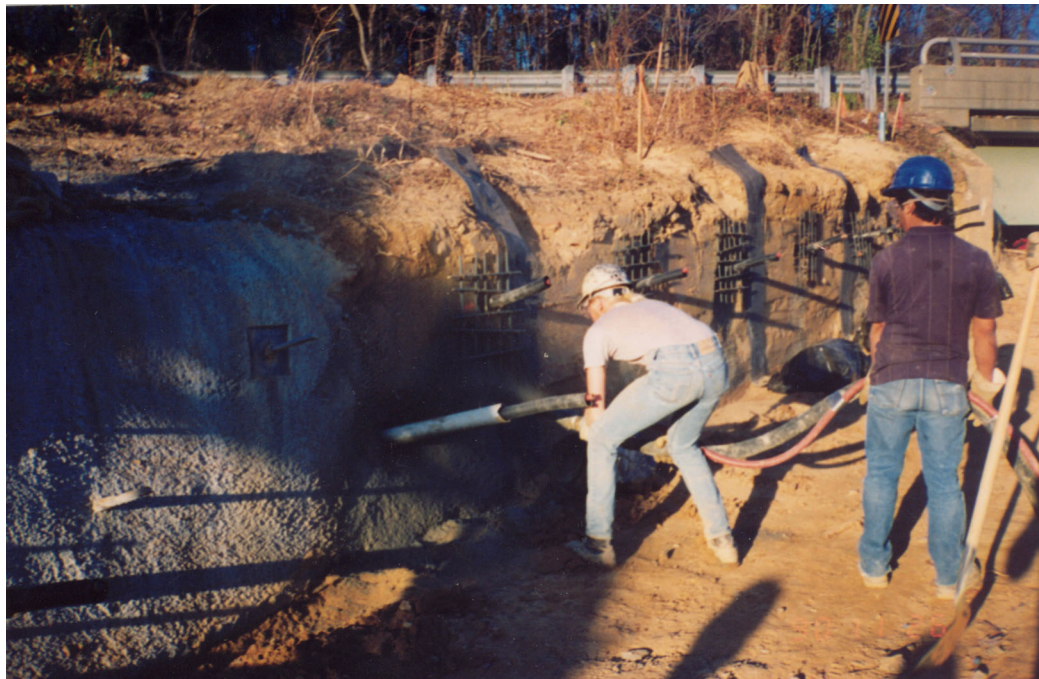
Figure 5. Grouting a Nail Hole.
