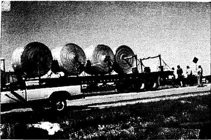
a) Prefabricated Edge Drain for Automated Installation
