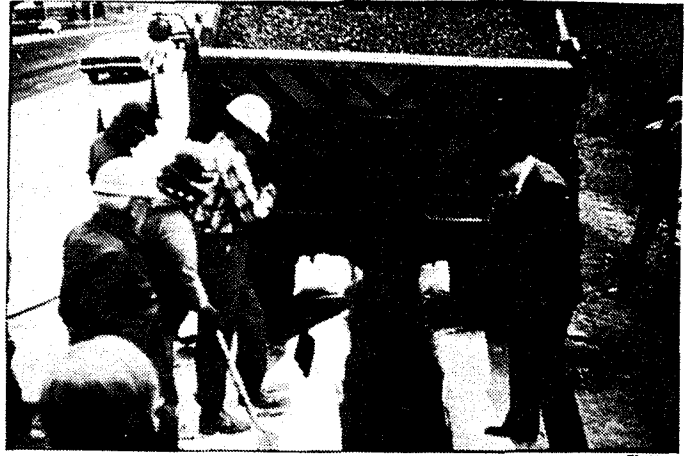
b) Aggregate Placement
