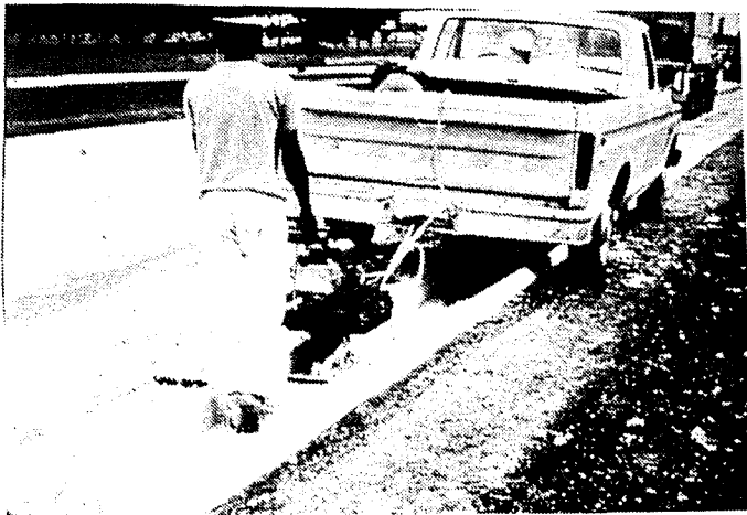
c) Compaction of Aggregate
