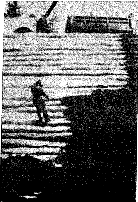
a) Geotextile Wrapped Face Temporary Wall
