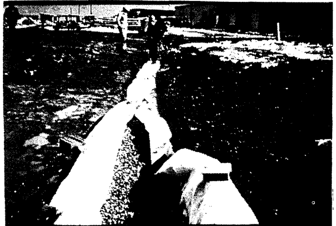
d) Geotextile Overlap prior to Final Cover
