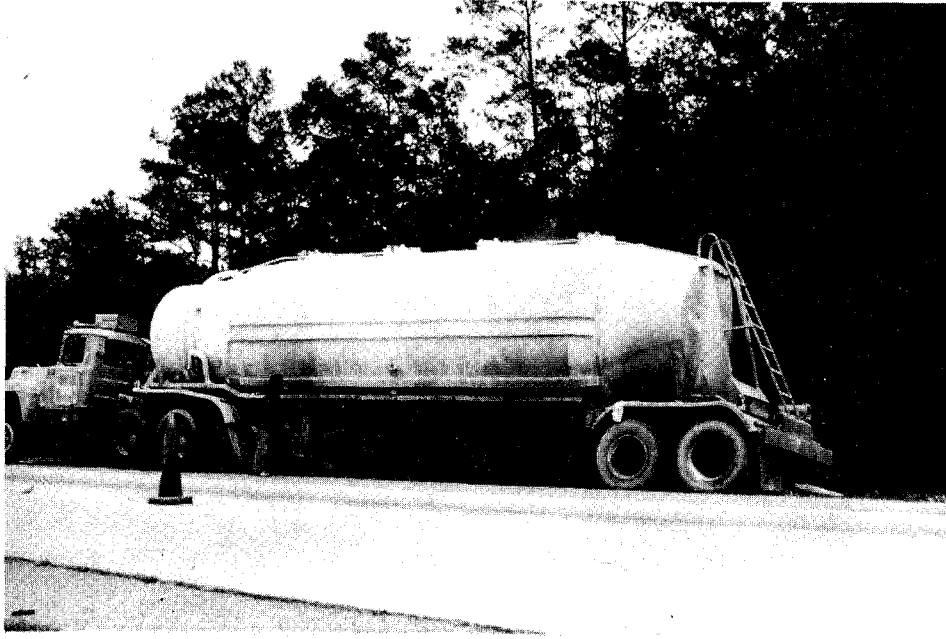
Photo 1 Lime and Fly-Ash hauled to jobsite in bulk and in the same tanker truck.
