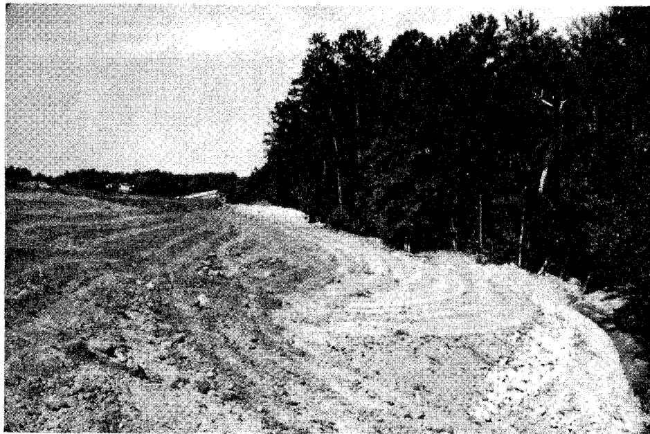
Photo 12 Rock Buttress and slope completely reconstructed except for grassing.
