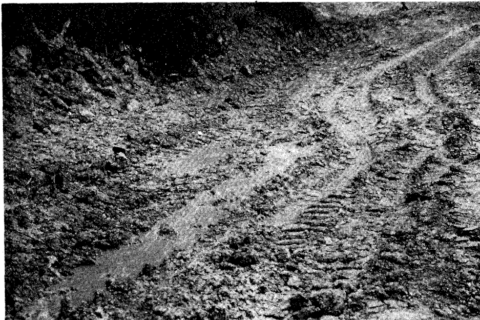
Photo 6 Eruption of slurry from ground approximately 50 feet from point of injection.
