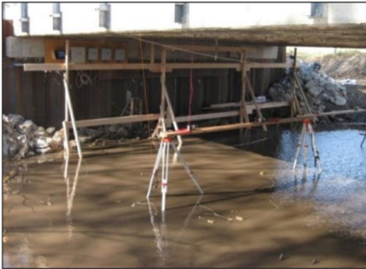
a.) View of west abutment
