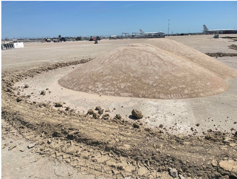
Figure 4.7 The fill sand used for the static pile loading test.
