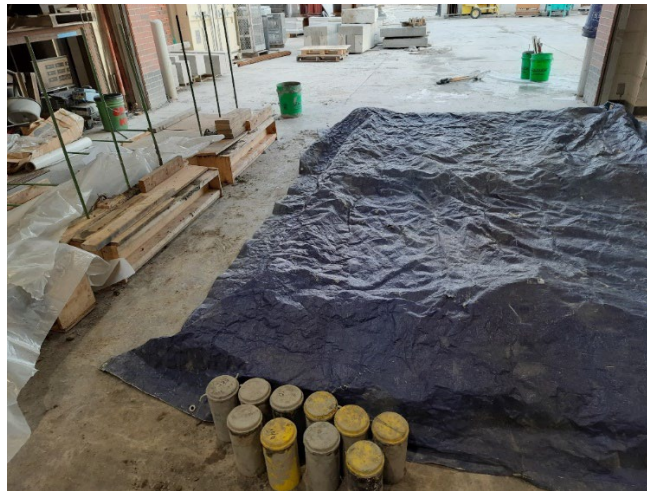
Figure 5.5 Curing of specimen in the mockup
