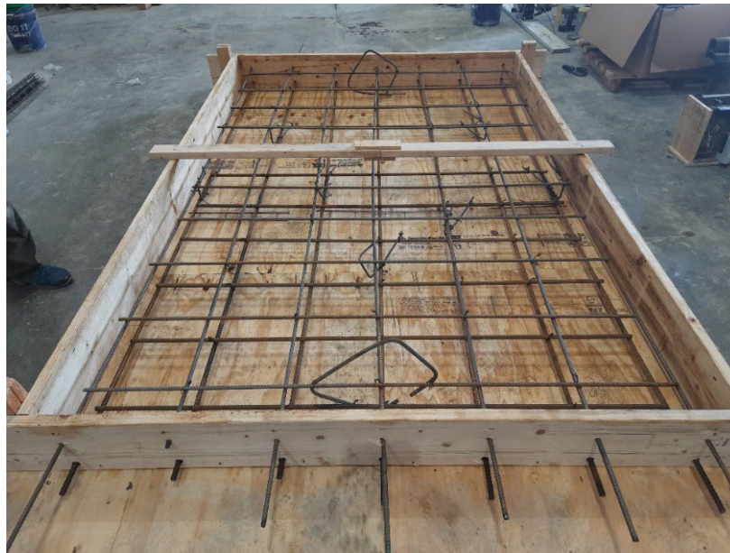
Figure 5.2 Form with rebars of deck slab specimen
