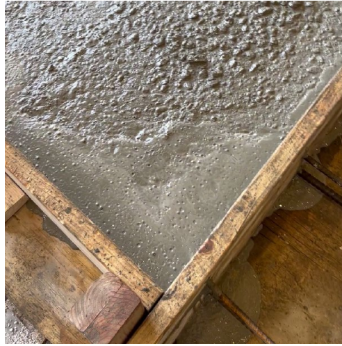
Figure 5.4 Bleeding of O47BD-R150 mix while pouring
