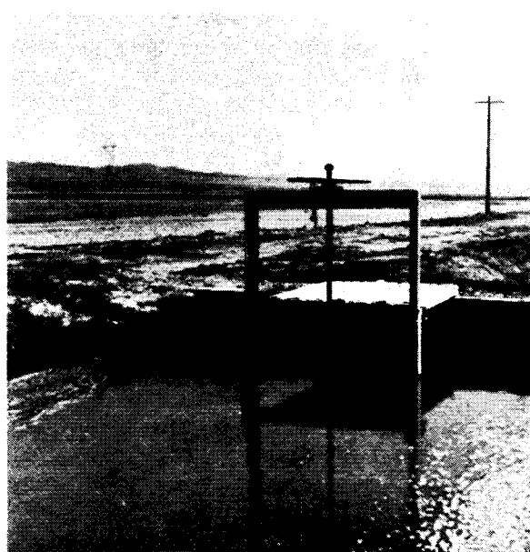
Figure 4-2. Check and pipe inlet in operation. P-222-116-53579D
