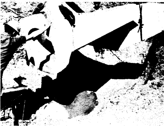
Figure 1-11. Placing precast concrete transition. P-707-729-2134
