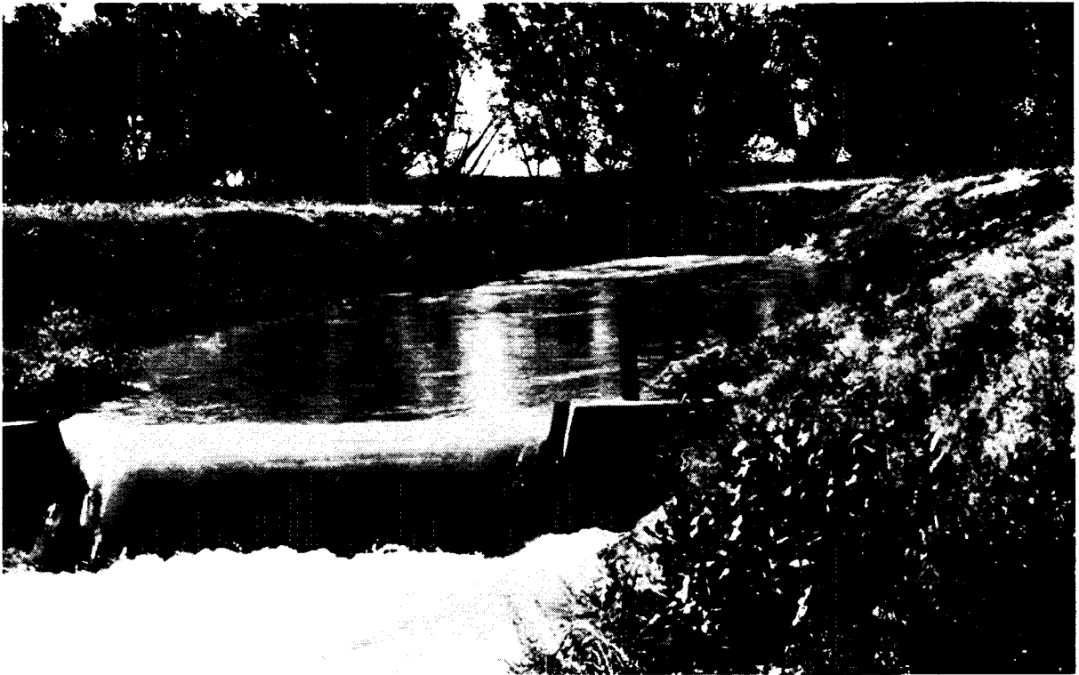
Figure 5-15. Water flowing over a standard Cipolletti weir. P20-D-34861
