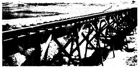
Figure 2-12. Elevated flume crossing natural drainage. PX-D-4592
