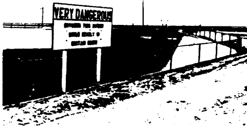
Figure 9-6. Warning sign, safety cable, and safety fence at siphon inlet. 805-236-14106
