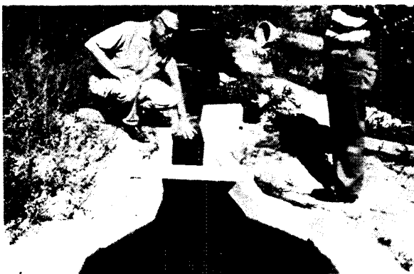
Figure 5-1. Flow through a 9-inch Parshall flume. P 20-D-29299-520
