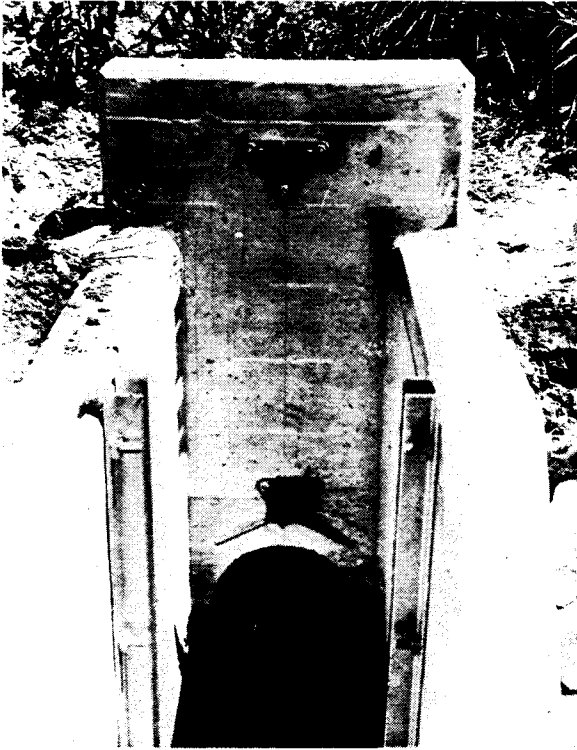
Figure 3-23. Farm turnout outlet. Brackets on headwall hold open-flow meter. Angles in foreground hold stoplogs to force conduit to flow full. P 499-700-383.
