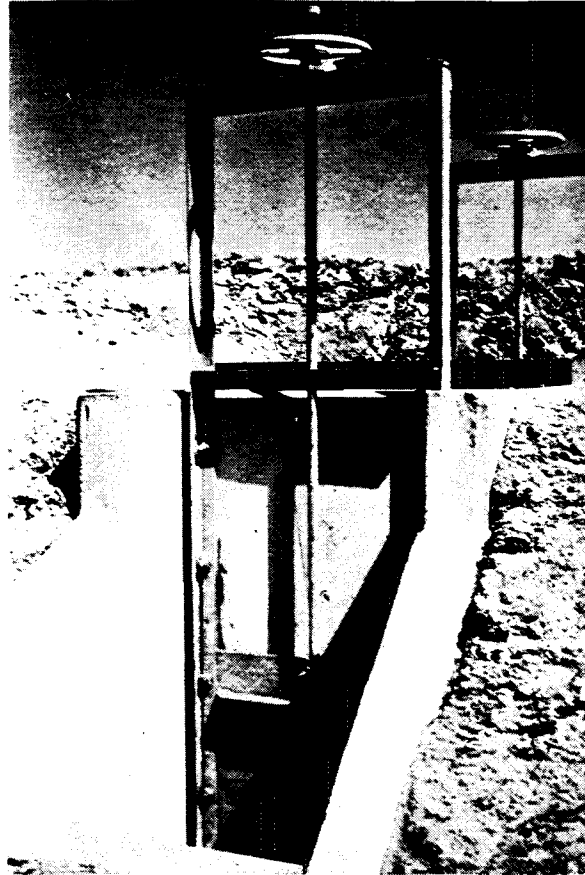
Figure 3-25. Constant-head orifice turnout inlet. PX-D-72618 D
