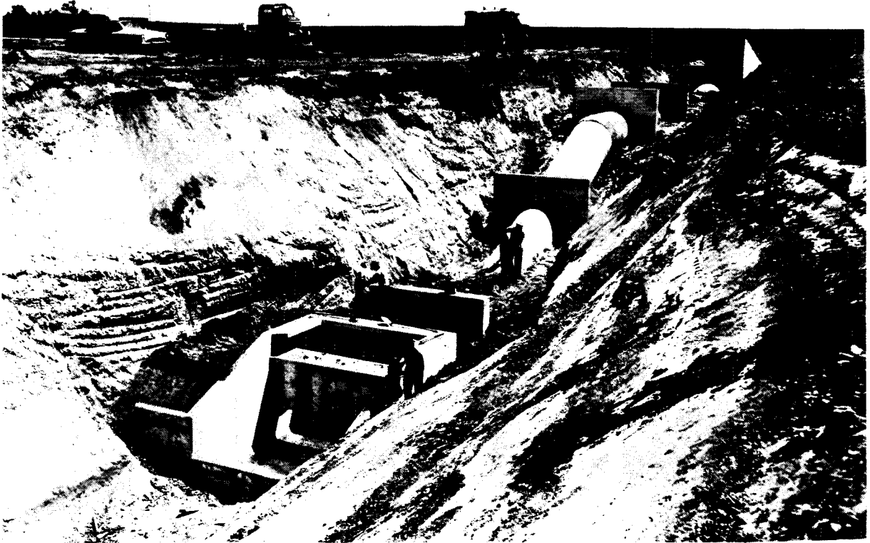
Figure 2-23. Pipe drop with baffled outlet and pipe collars. P 328-701-8417
