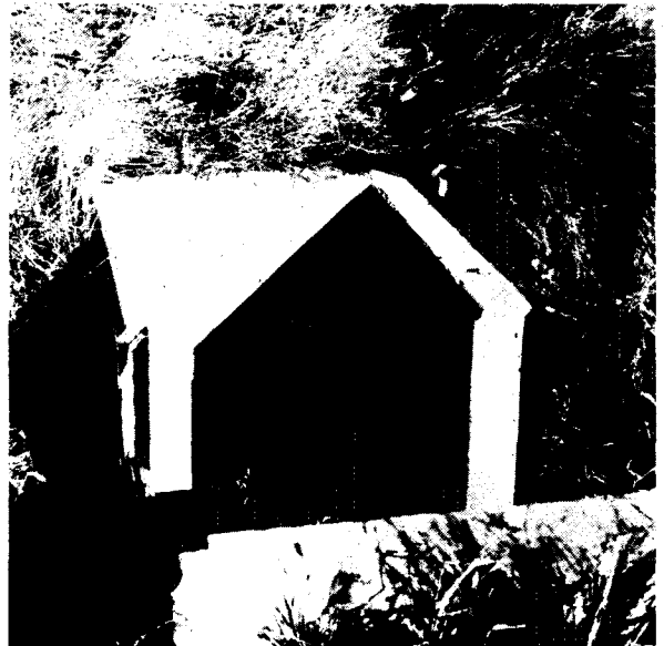
Figure 3-34. Division structure used as outlet to turnout. P 328-701-7166
