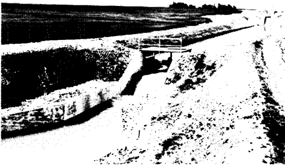
Figure 2-18. Series of rectangular inclined drops. P-328-701-7738
