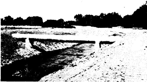
Figure 4-31. Steel pipe overchute on the Colorado-Big Thompson Project. P-245-713-300
