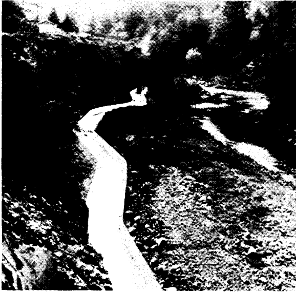
Figure 2-10. Concrete bench flume.
