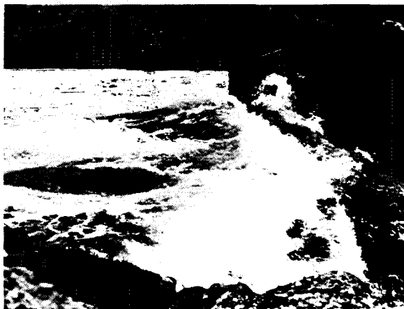
Figure 2-48. Wave sweeping through the outlet transition of a stilling pool. Flow is 140 cfs. P222-117-36227
