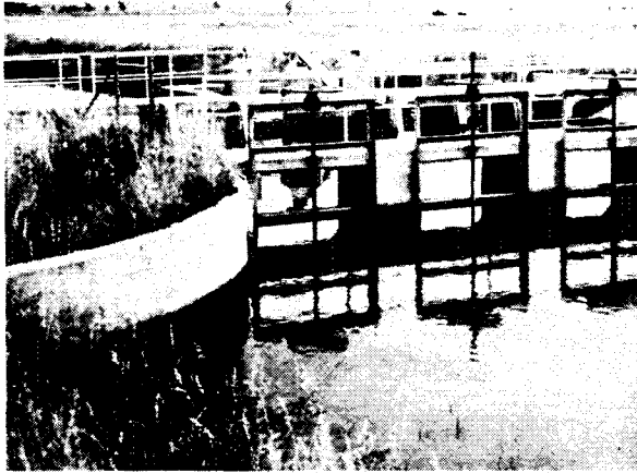
Figure 3-28. Constant-head orifice structure used as a check. Structure maintains upstream water surface and measures flow in the canal. PX-D-72605
