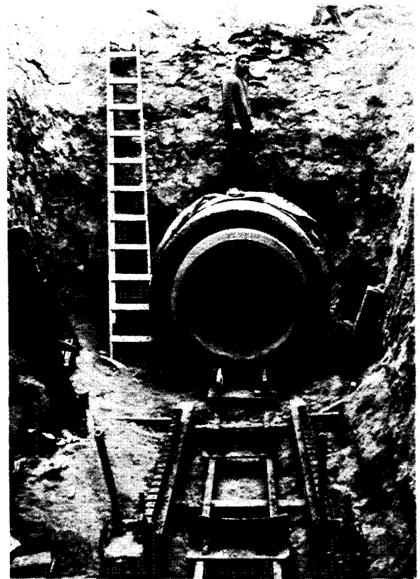
Figure 2-3. Jacking and threading pipe under roadway. P-707-729-2007.
