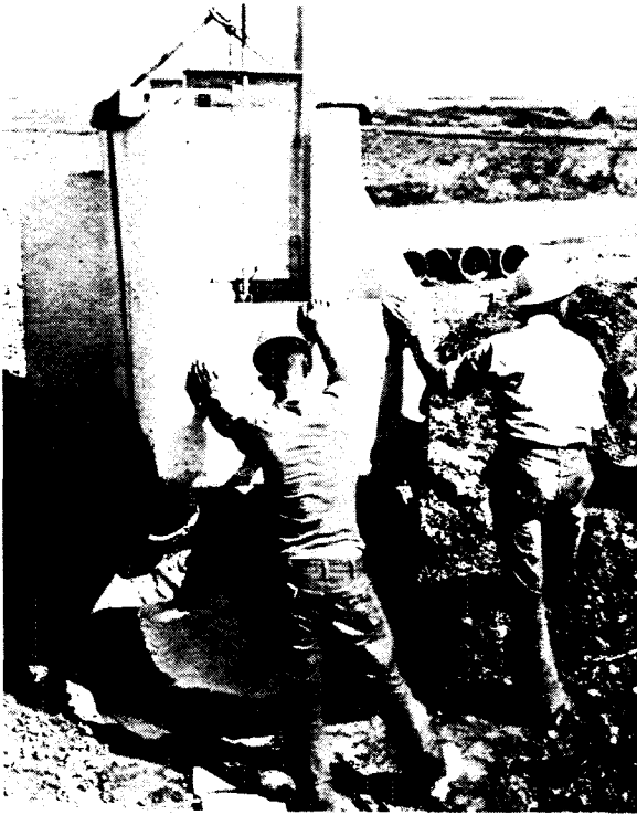
Figure 1-13. Precast concrete turnout inlet being lowered into position on mortar pad. P-707-729-1769
