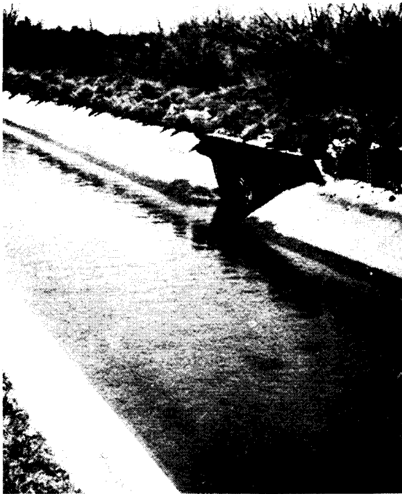
Figure 4-40. Drain inlet with flap gate to prevent reverse flow. PX-D-73101
