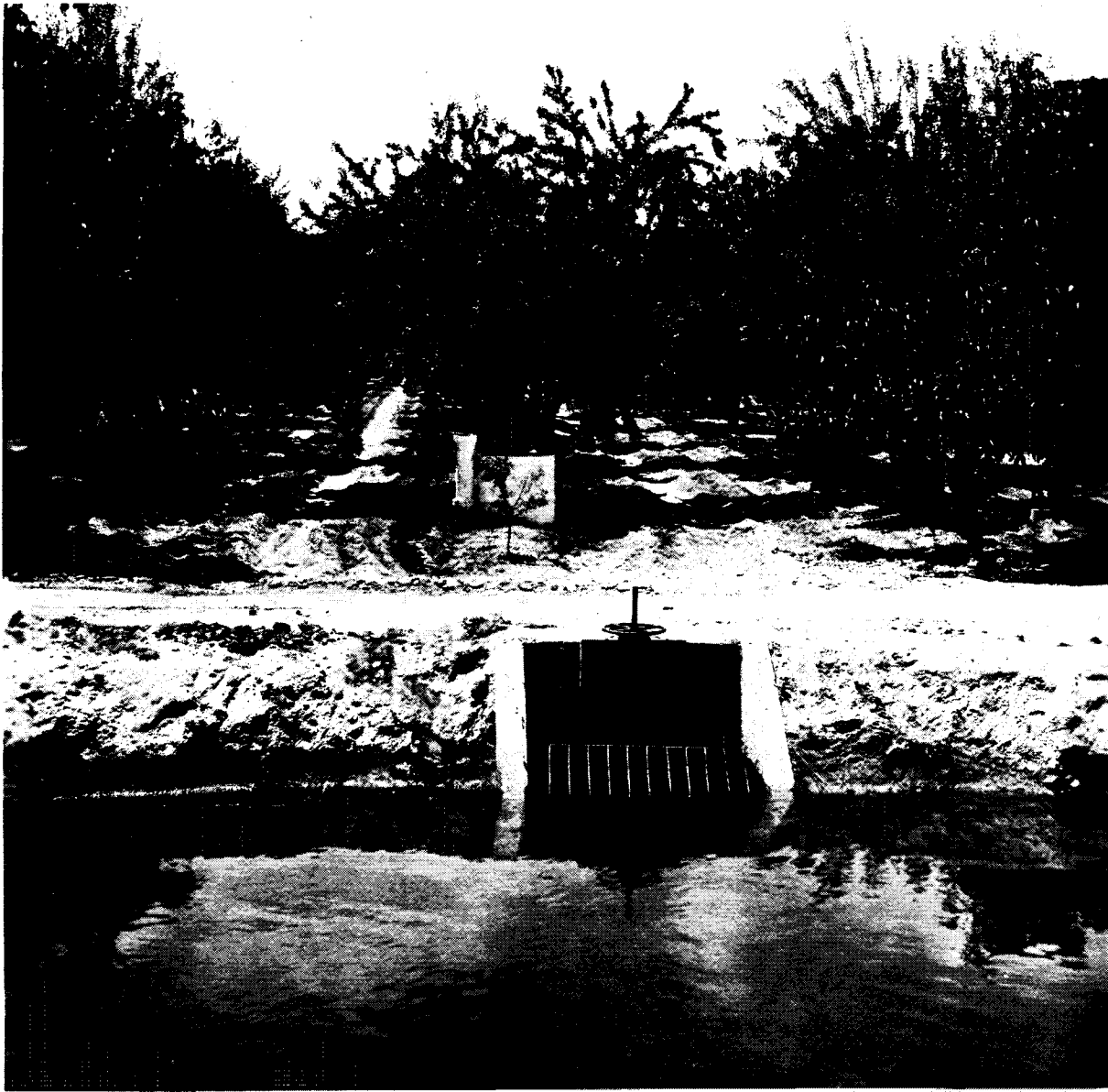
Figure 3-19. Turnout structure in earth channel. P214-D-73783
