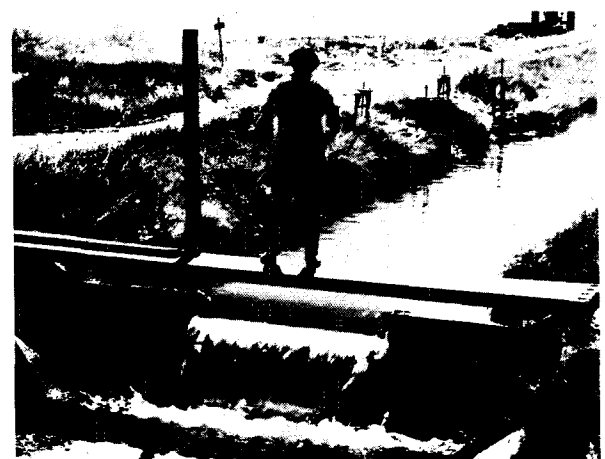
Figure 3-7. Operator removing stoplogs from a check-drop structure. Constant-head orifice turnouts in background. P-606-600-66A
