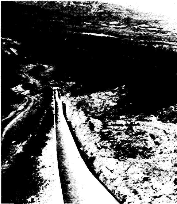
Figure 2-34. Rectangular concrete chute on a steep slope. P 482-417-908
