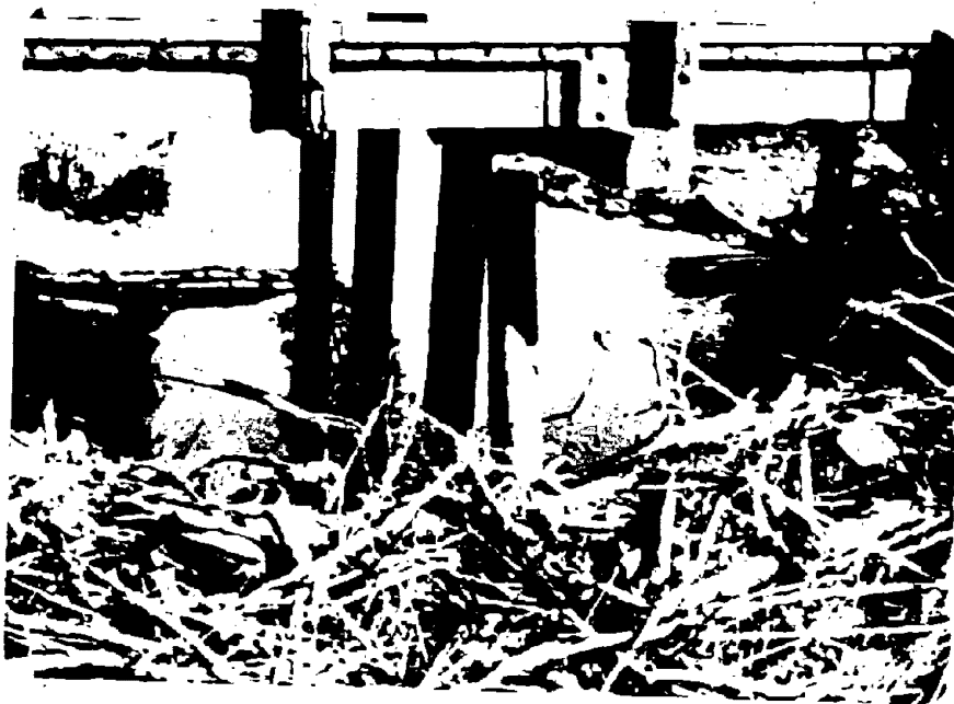
Figure 3 A Bridge on the Bayou Plaquemine, Acadia County, Louisiana
