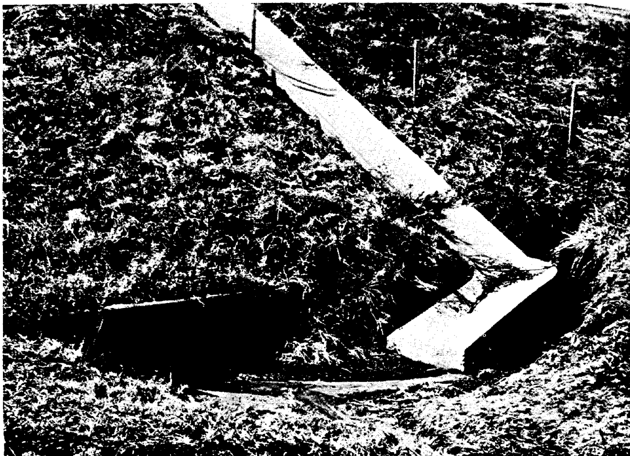
Figure 22.—Chute with sharp change in alignment. Note erosion due to sharp curvature.
