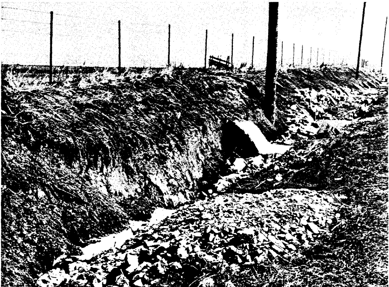
Figure 4.—Poorly designed ditch checks.
