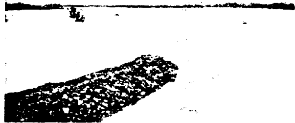
Figure 32.—Spur dike on 45^\circ skewed bridge over Susquehanna River at Nanticoke, Pa.
