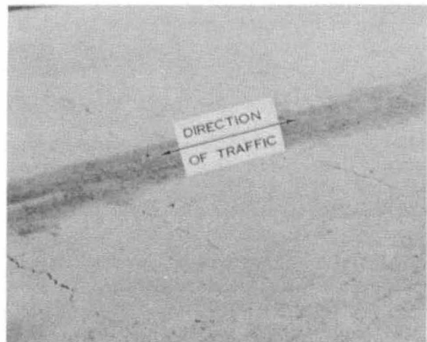
Figure 5-6. Transverse cracking.
