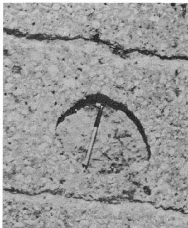
Figure 5-12. Small surface spall.
