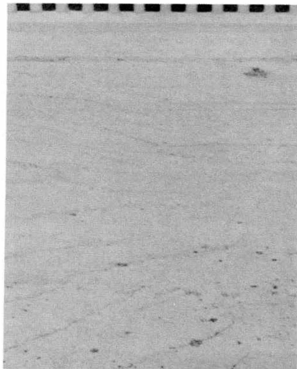
Figure 5-8. Diagonal cracking.
