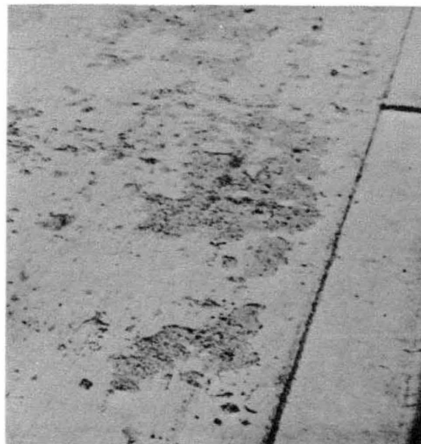
Figure 5-2 Light scale. Scale depth is less than \frac{1}{4} ".
