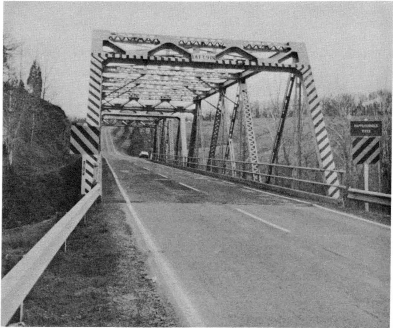
Figure 5-124. Approach to narrow bridge. Note paddle boards and striping of endposts and portal chord.
