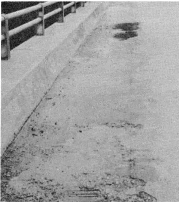
Figure 5-5. Severe scale. Scale depth is greater than 1". Note dislodgement of coarse aggregate and exposure of reinforcing bars.
