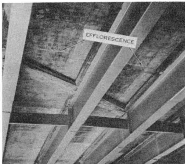
Figure 5-85. Transverse cracks. Note cracks are near inflection point, and are transverse even though deck is skewed. Note efflorescence.
