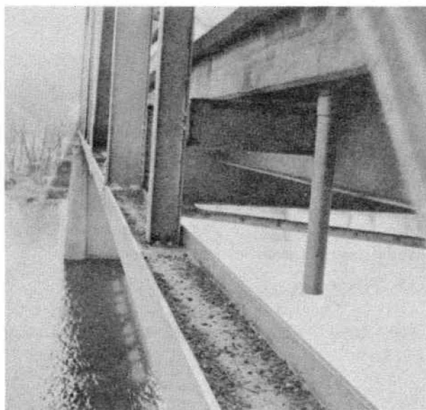
Figure 5-65. Panel point connections along lower chord. Note the collection of debris along the horizontal surface of the bottom chord.
