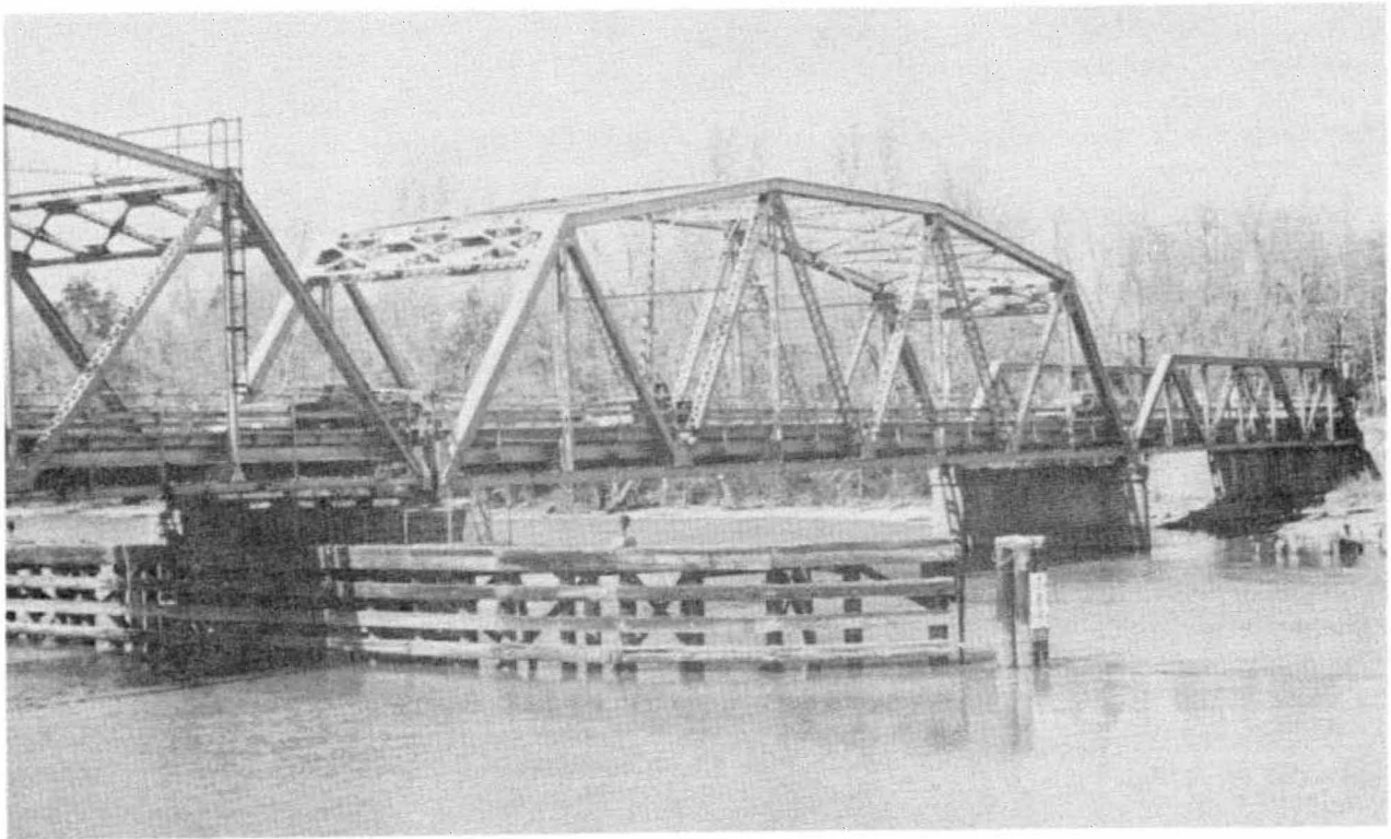
Figure 5-100. Timber bent fenders.
