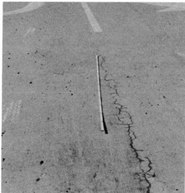
Figure 5-83. Longitudinal deck crack.
