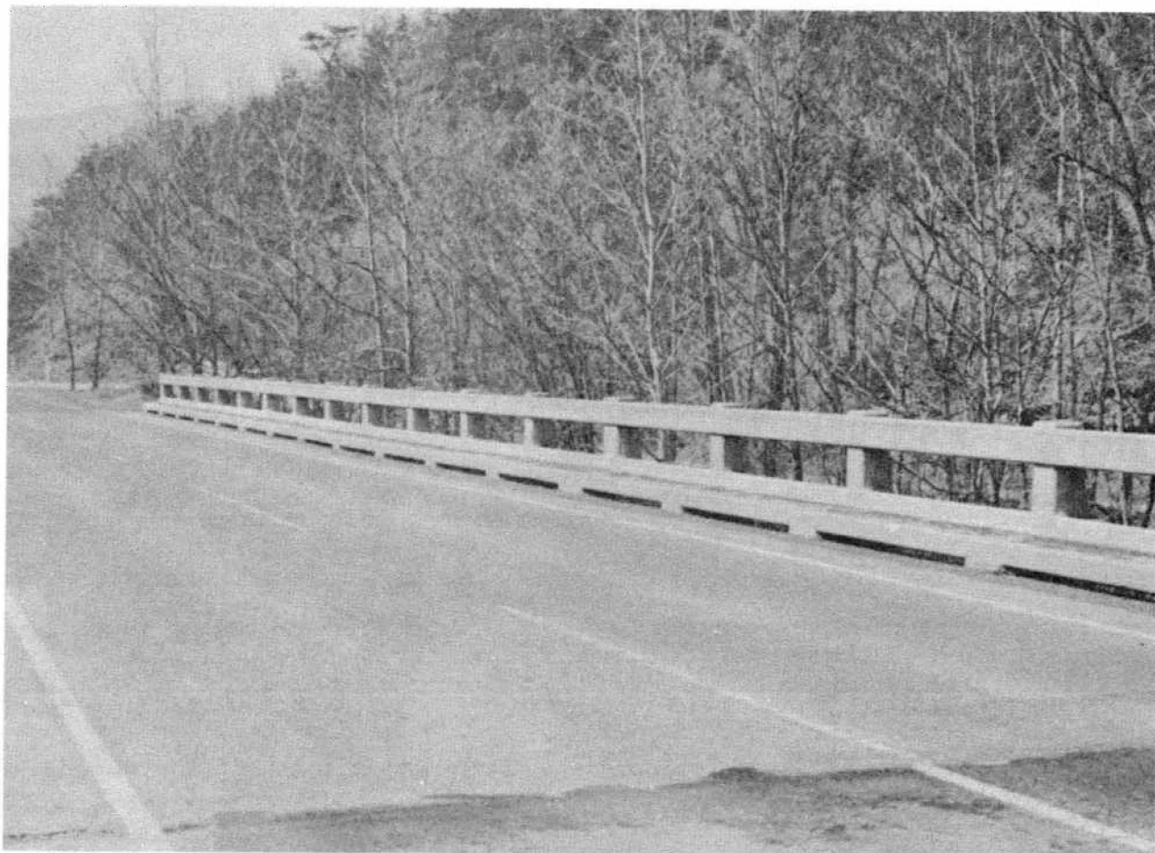
Figure 5-91. Concrete railing and curb.
