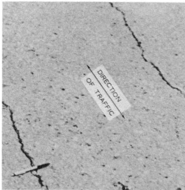
Figure 5-7. Longitudinal cracking.
