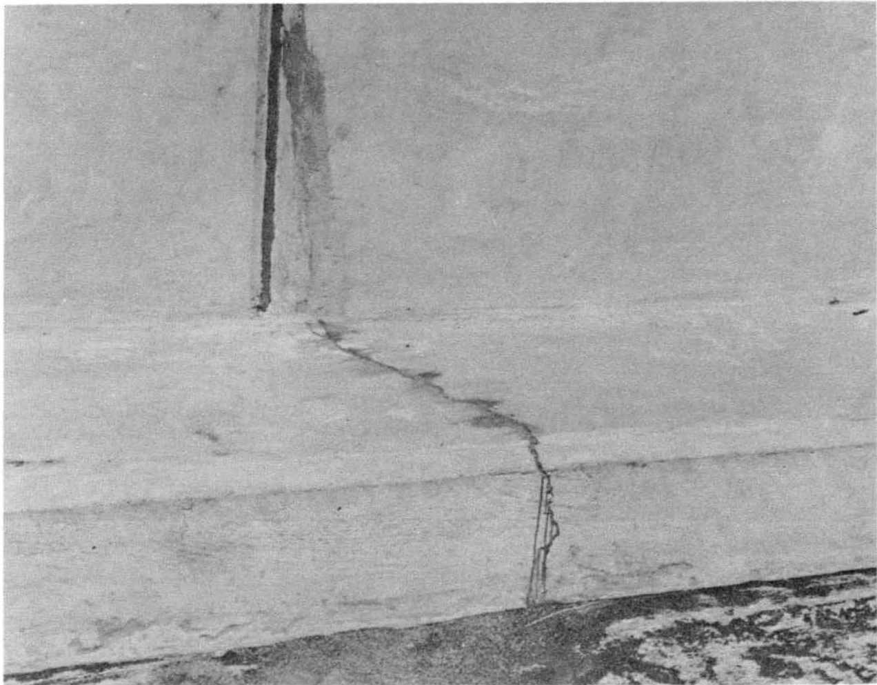
Figure 5-94. Crack through safety curb. Crack started at parapet joint and continued across curb and deck. See also figure 5-84.
