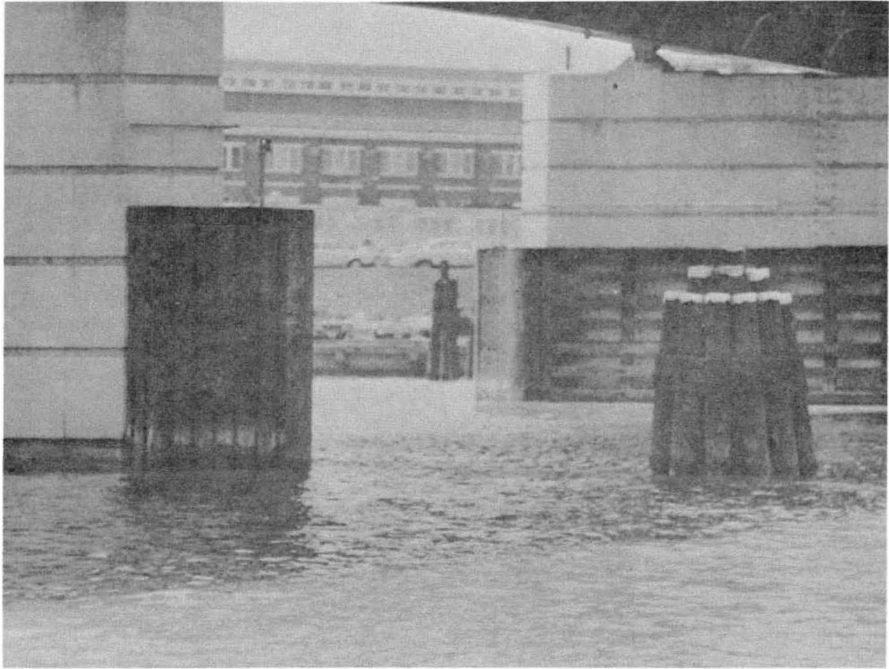
Figure 5-99. Timber pile cluster dolphins and timber fender system on pier.
