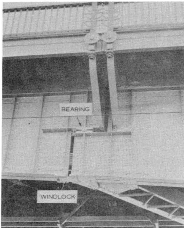
Figure 5-79. Cantilever girder with direct bearing. Note windlock.
