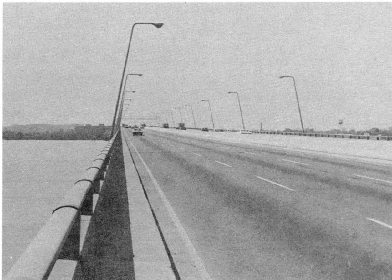
Figure 5-90. Concrete parapet and sidewalk with steel tubular rail (left) and concrete median barrier (right).
