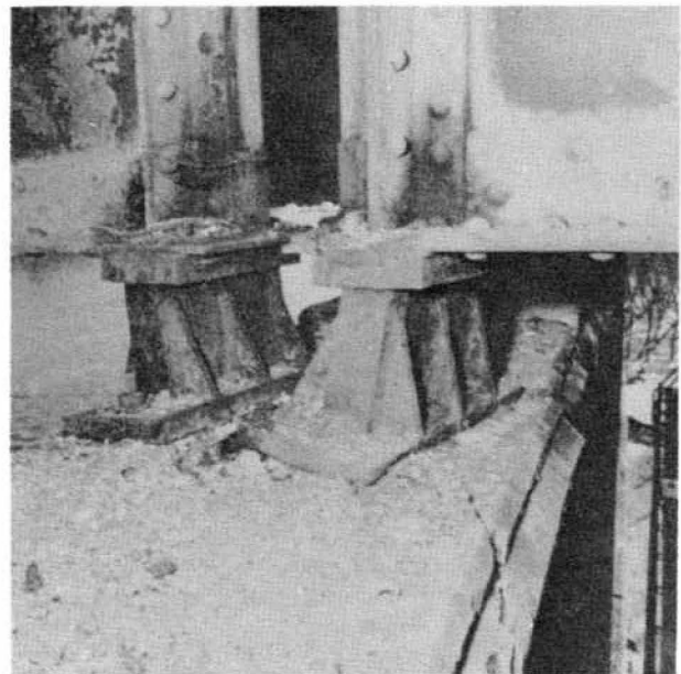
Figure 5-1. Concrete damaged by intense heat. Note the cracking and spalling of the reinforced concrete pier cap.
