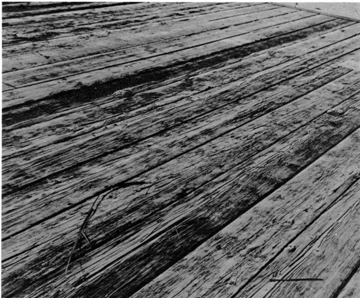
Figure 5-28. Weathering and wear of untreated timber deck.
