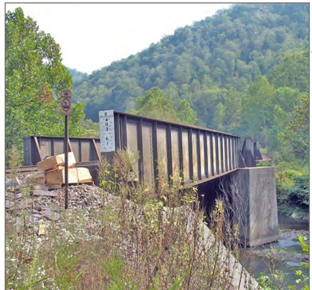
Half-Through Girder Bridge at Mile Post 403.61 Adjacent to the East Portal of Antler Tunnel #1, near Mohegan, McDowell County, West Virginia.
