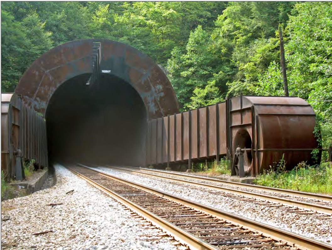
Elkhorn Tunnel West Portal with Ventilating Fans, Mile Post 375.52, Elkhorn, West Virginia. Source: TRC, October 2007.
