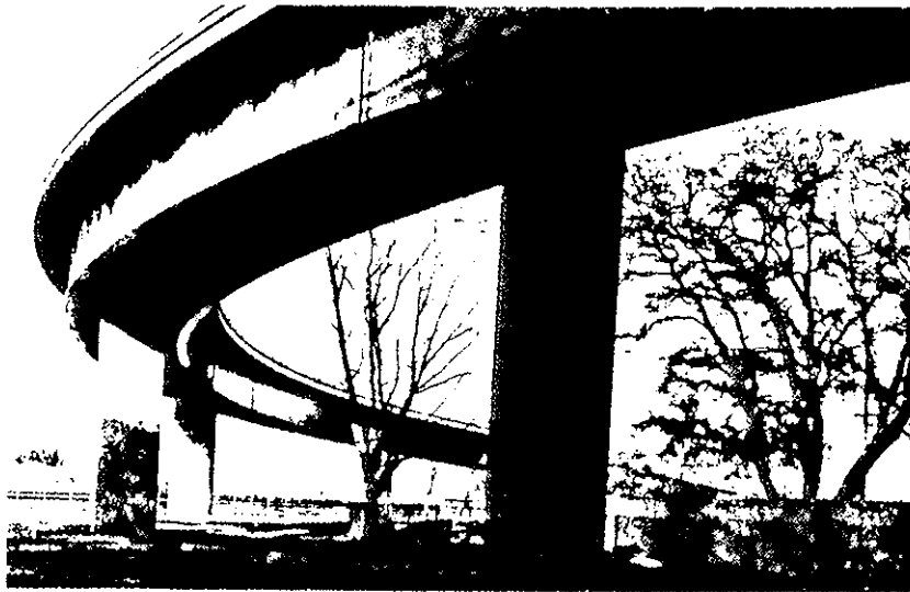
Figure 2.7 Curved Girder Bridge
