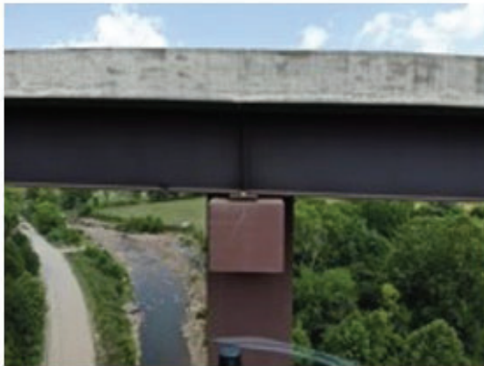
(a) Bridge pier cap (normal view)
