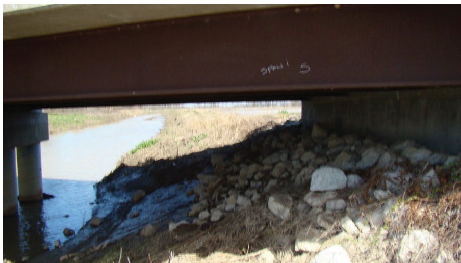
Figure 52. Bridge 07225 Viewing East Abutment from Southside of Bridge
