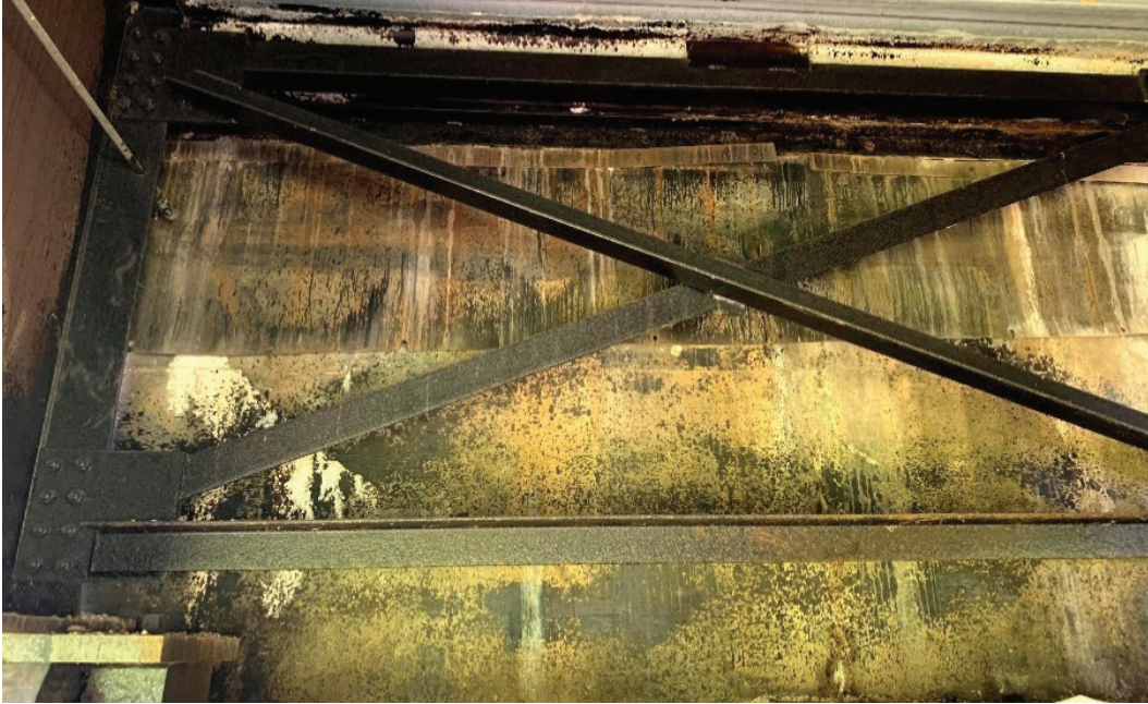
Figure 13. Rust Inhibitor at End Abutment
