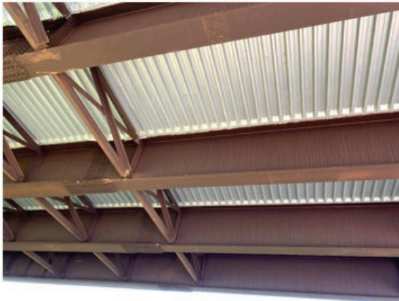
(a) ARDOT Bridge A6284: CS 1
