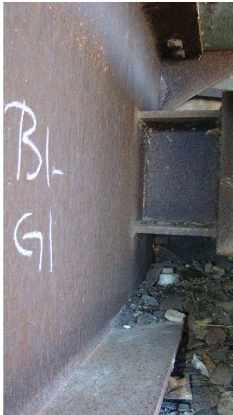
Figure 61. Girder Support at Fascia Girder
