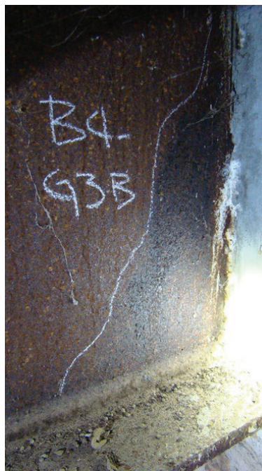
Figure 58. Bridge 07335, Bent 4, Girder 3
