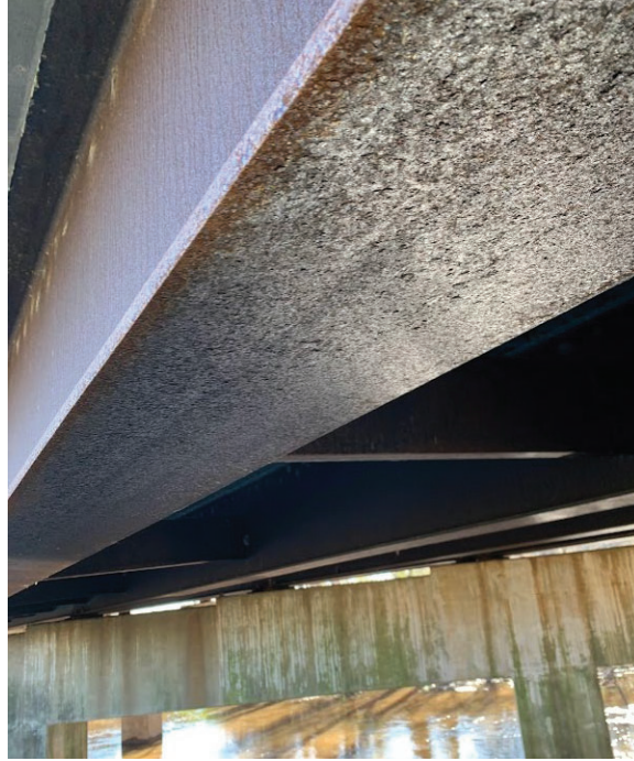
Figure 40. Bridge 02312: CS 2 Under Flange
