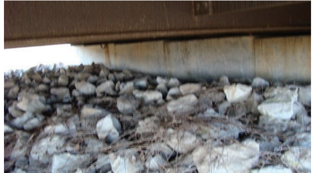
(b) Bridge B6401 at North Abutment
