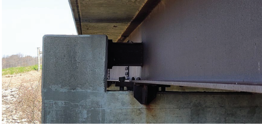
Figure 62. Bridge A6401. Seismic Restrictive Devices Used at Piers
