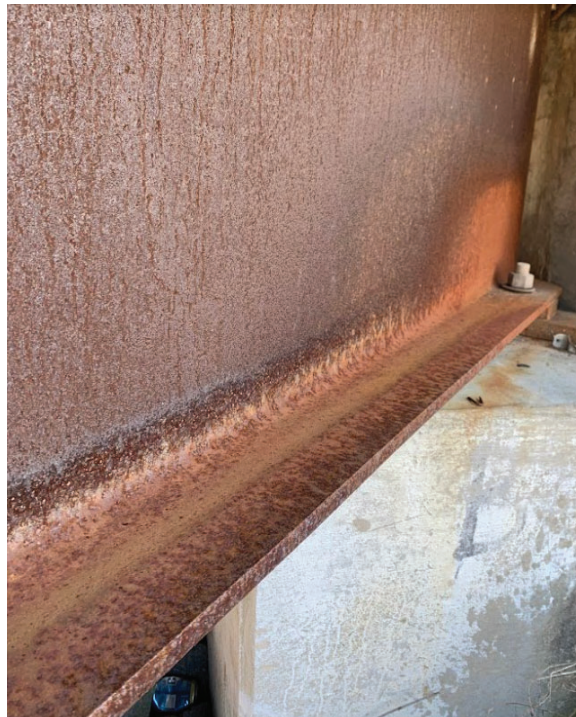
Figure 41. Bridge 02312: CS 1 and CS 2 on the Outside Web and Flange
