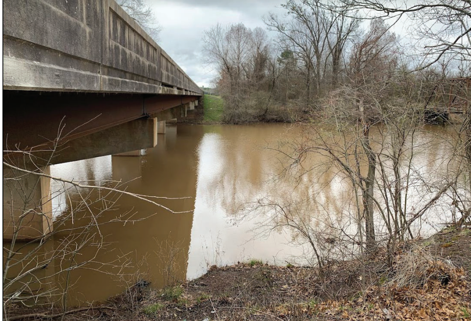
Figure 38. Bridge 05812 over Water
