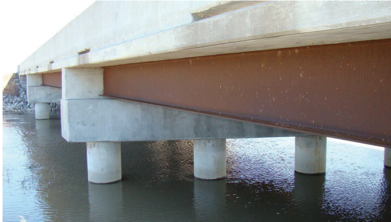
Figure 53. Bridge 07335, North Side of Bridge Looking East
