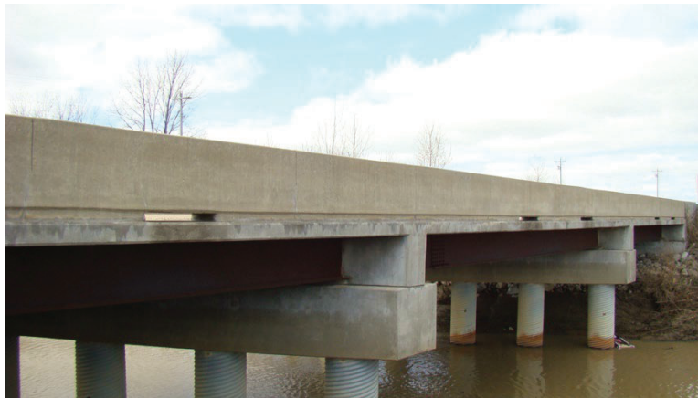
Figure 50. North Side of Bridge 07225
