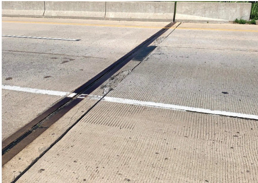
Figure 12. Bridge Deck Expansion Joint
