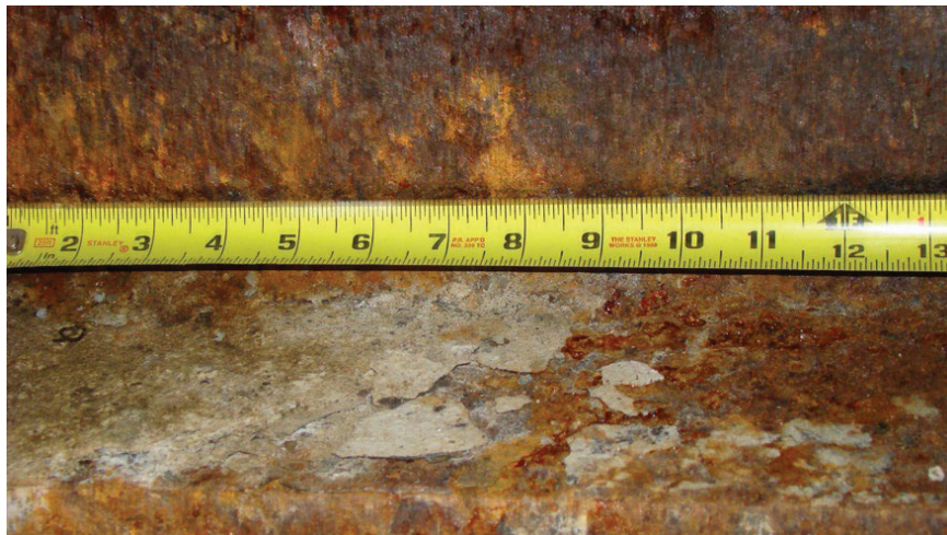
Figure 54. Bridge 07335, Girder 4, Bent 4
