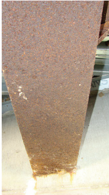
Figure 55. Bridge 07335, Bent 4, Girder 4, Bottom of Girder Flange
