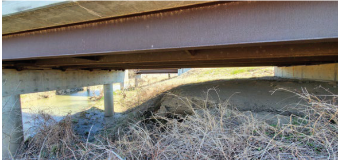
(a) Bridge A6401 at South Abutment
