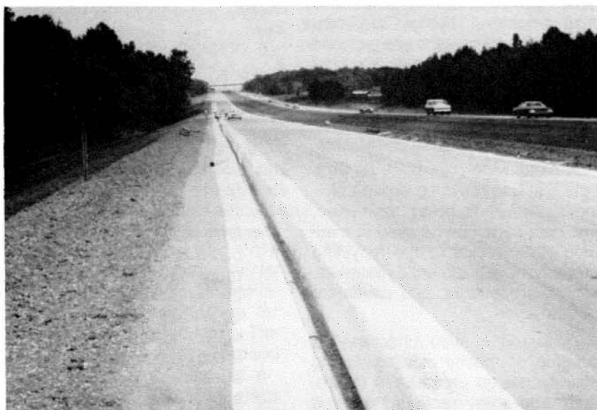
Trench in shoulder area with subsurface drainage pipe in place.
