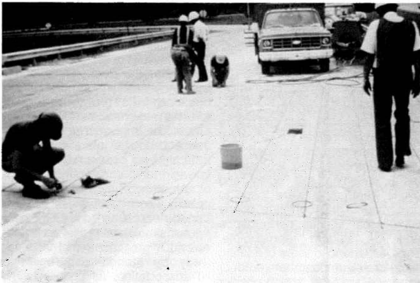
Overall view of bridge deck at New Columbia, Pa. Platinum anodes were laid in precut slots backfilled with conductive polymer concrete.
