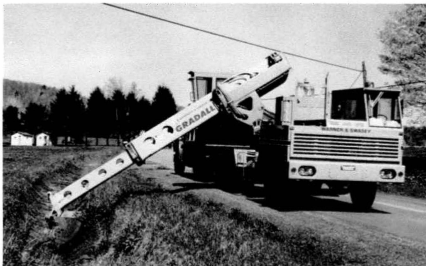
Cleaning a ditch parallel to the roadway.
