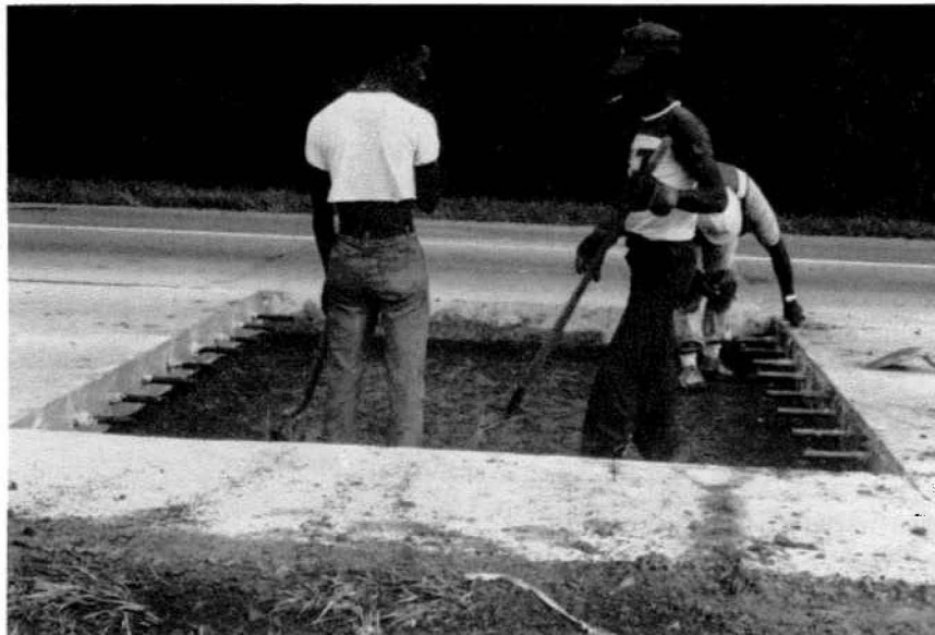
Reestablishing load transfer devices during rigid pavement repair.
