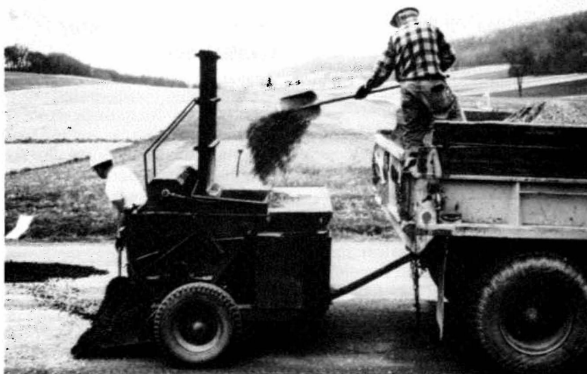
Heater-mixer for supplying hot asphalt for pothole patching.
