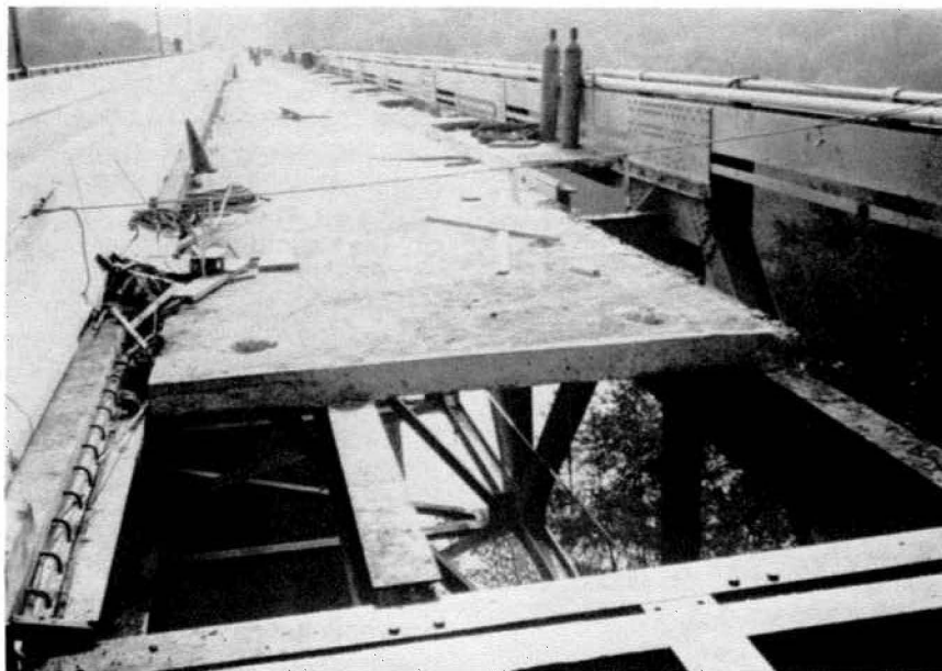
Replacement of the deck on a through-girder bridge with reinforced concrete panels connected to the stringers to provide composite action.
