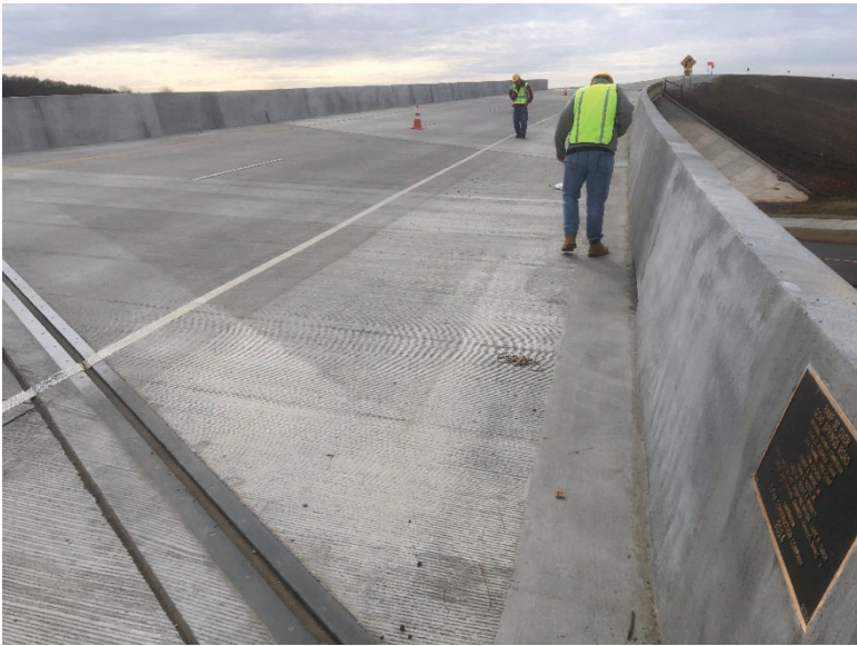
Figure 6. Bridge 07315 Lowell, AR Looking Southwest
