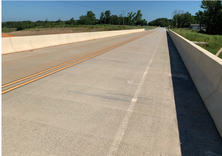
Figure 8. Bridge 07273 Looking Northwest
