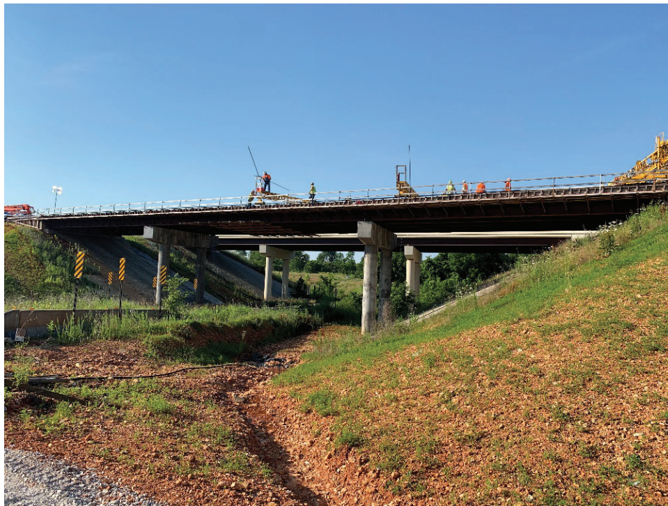
Figure 15. Picture of Bridge No. A7195 Taken from the North
