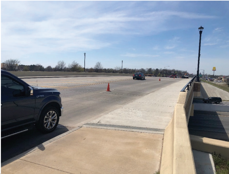
Figure 7. Bridge 05945 in Springdale, AR Looking to the East
