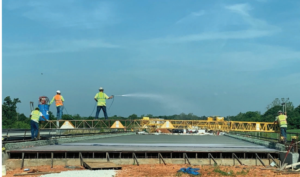
Figure 65. Workers Spraying White Curing Compound on Bridge After 2nd Pour
