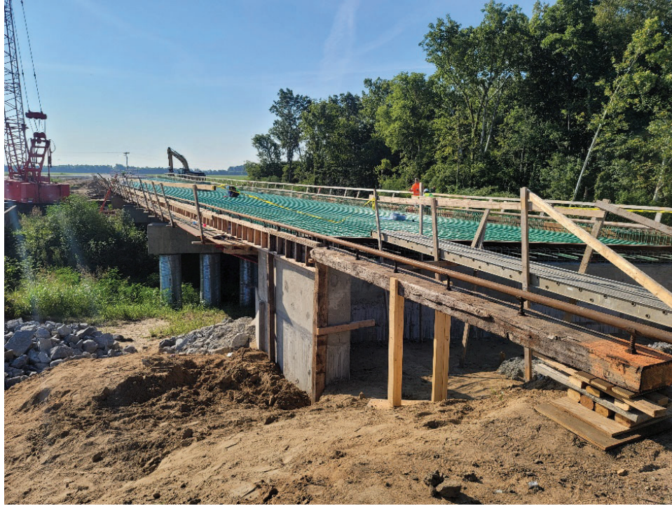
Figure 18. Image of Bridge No. 07473 Taken from Northwest Corner
