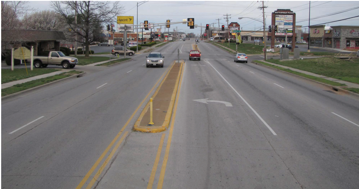
EXHIBIT 5-2 Short median strip to restrict left-turn access
