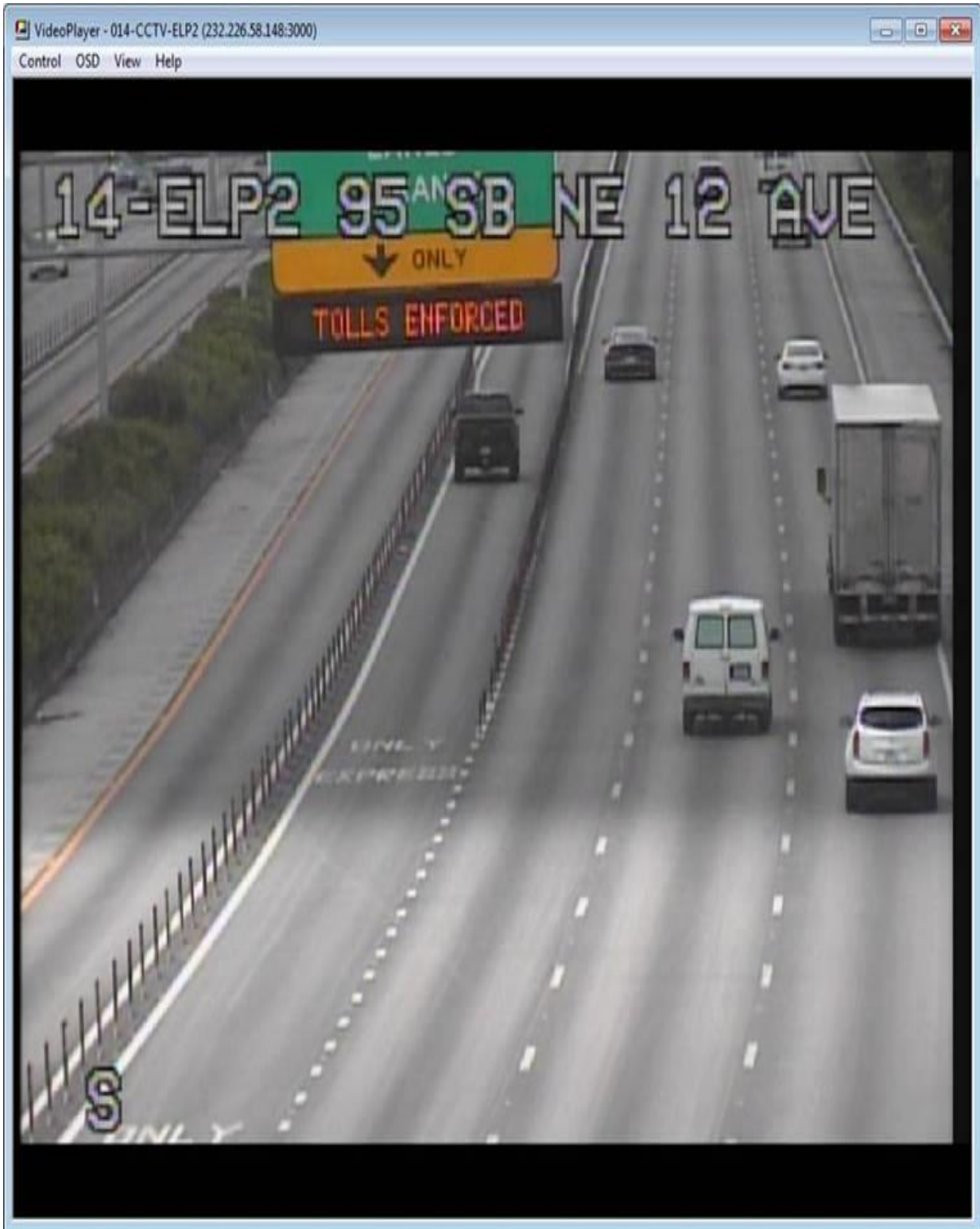
Figure 4: Asphalt Site 1—I-95 Express Lanes Southbound ramp from I-95 Mainline/Ives Dairy Road (CCTV-014 ELP2)
