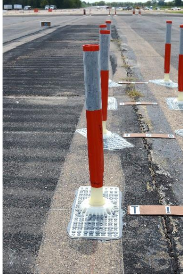
Figure 3.59. 607531-02-9 Sample (Concrete Surface).
