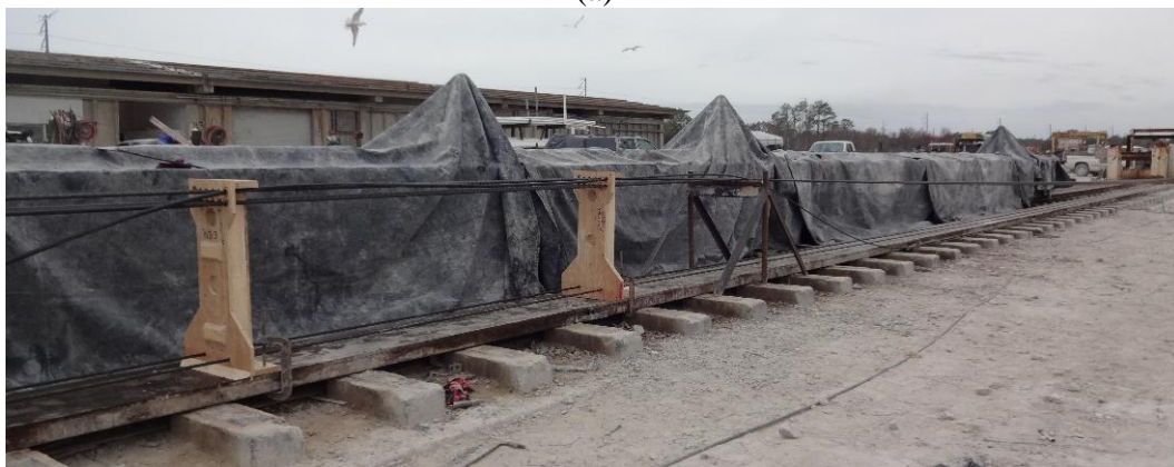
Figure 7.3 Bulkheads and steel deflectors for prestressing strands: NB precast beams
