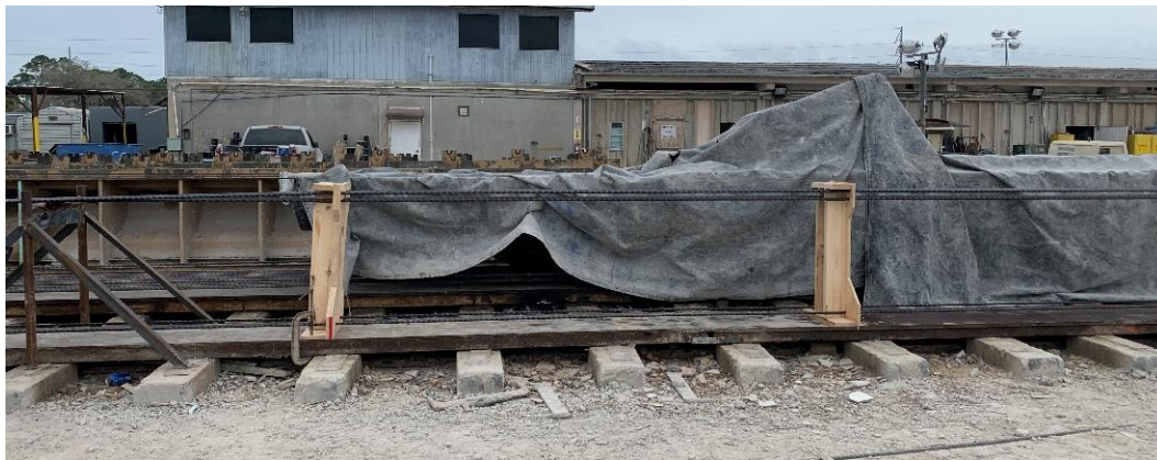
Figure 7.2 Custom plywood bulkheads for NB precast beams
