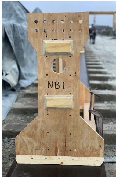
Figure 7.2 Custom plywood bulkheads for NB precast beams
