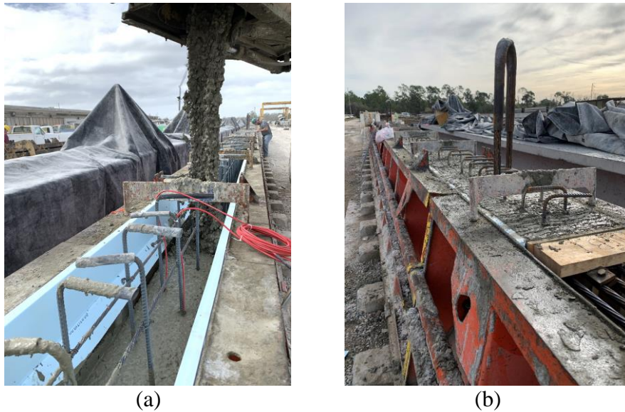
Figure 5.12 (a) Concrete placing and (b) roughened top surface
