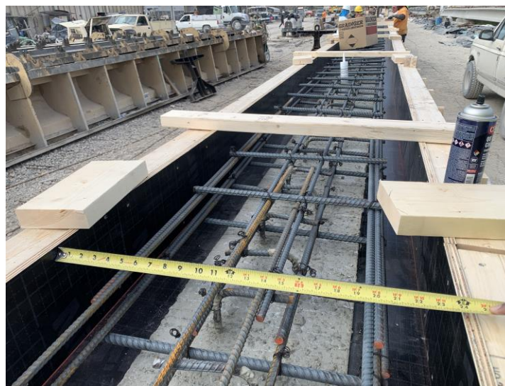
Figure 5.13 Mild steel reinforcement for concrete deck
