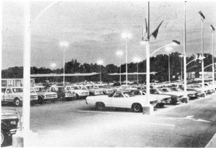
Figure 41. Common twin mast arm support placed along the spine of parking rows in shopping center.
