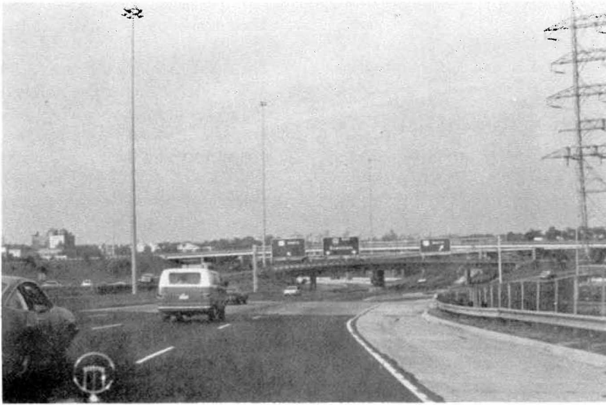
Figure 17. Common high mast configuration.
