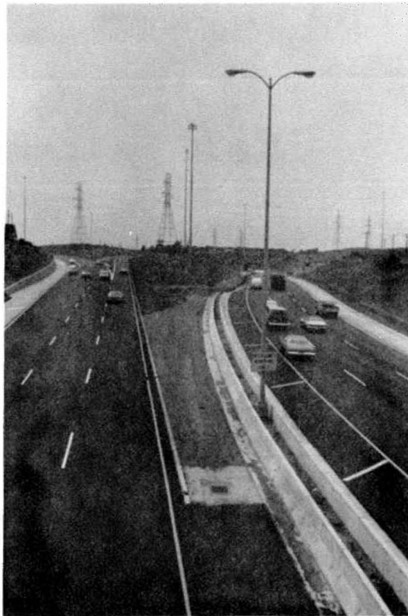
Figure 26. Wisconsin split concrete median barrier.
