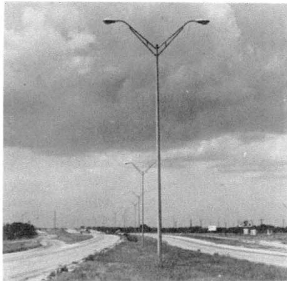
Figure 22. Example of median-mounted lighting in wide median.
