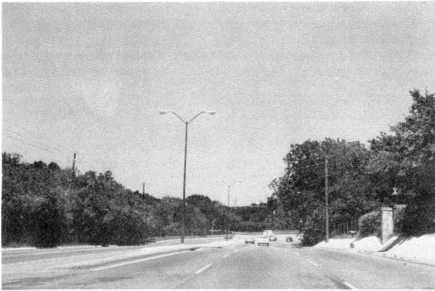
Figure 33. Median-mounted lighting on arterial street.
