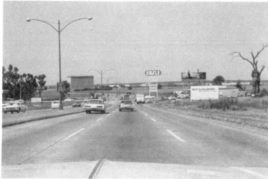
Figure 11. Typical luminaire support with mast, mast arm, base, and foundation.
