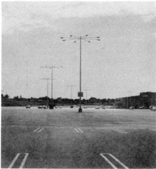
Figure 42. Multi-armed support used for parking lot lighting in shopping center.
