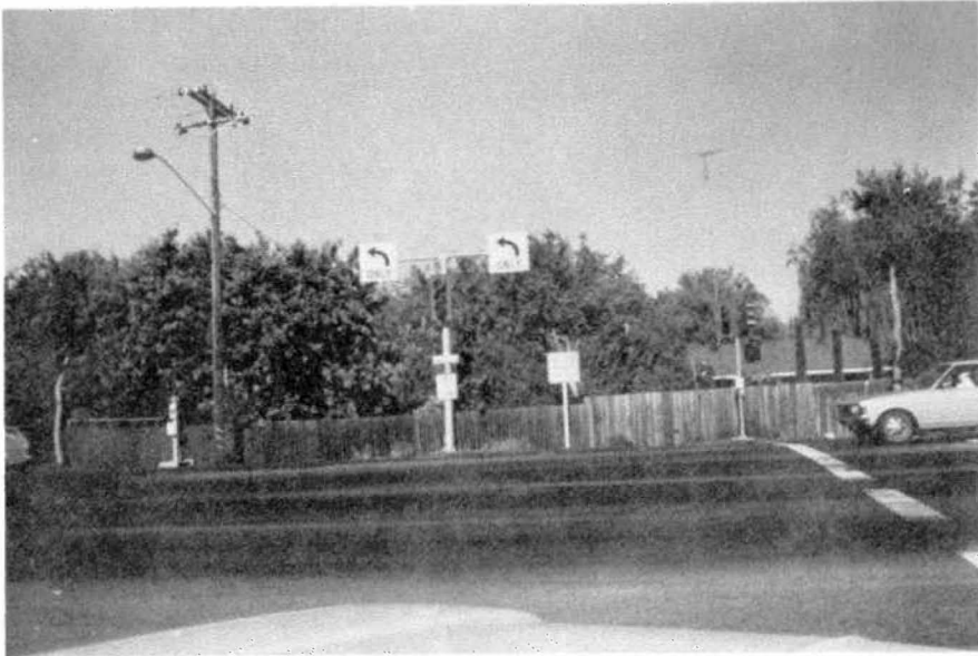
Figure 66. Power pole-mounted luminaire.
