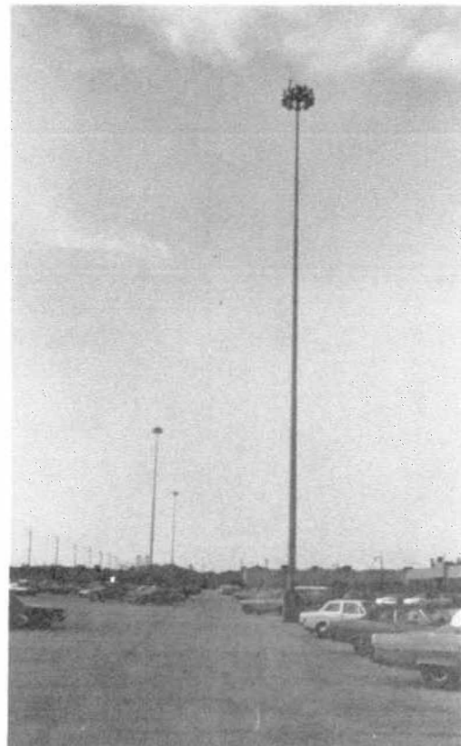
Figure 43. High mast lighting used in shopping center parking lot.
