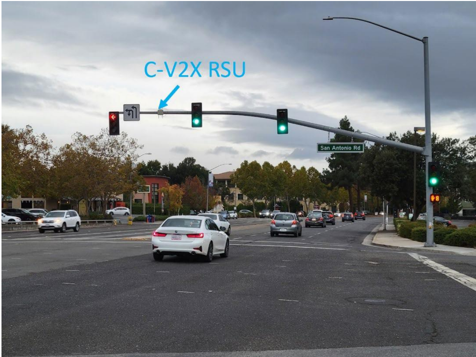
Figure 8 C-V2X RSU Installed at San Antonio Rd @ ECR
