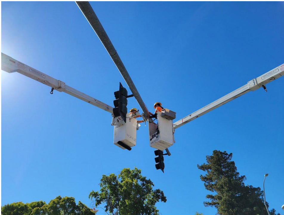
Figure 7 Mounting the RSU on the Mast Arm (From left to right: Daniel Bu and Antonio Lopez)
