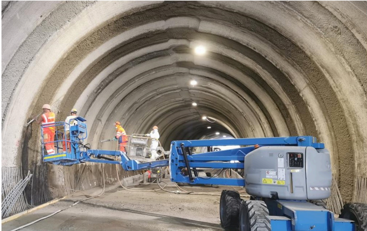
Figure 6. Photo. T5 tunnel rehabilitation construction.
