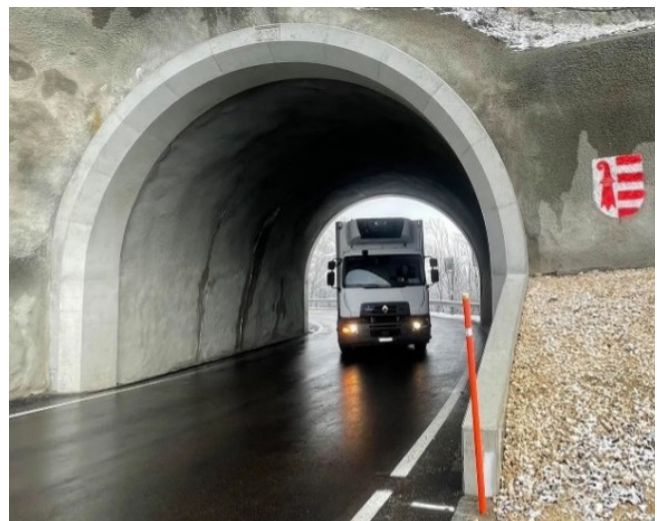
B. After rehabilitation.
