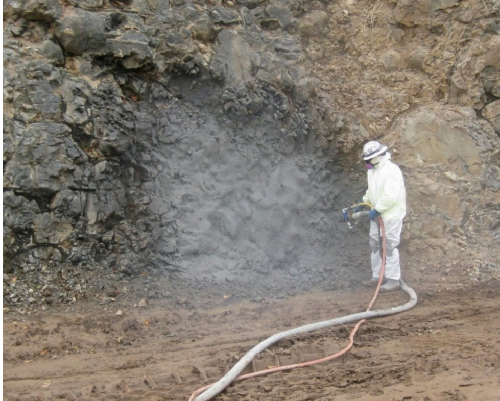
© 2020. Florida Department of Transportation, courtesy of UHPC Solutions North America.
