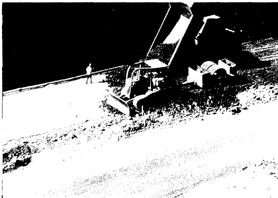
Figure 79. Placement of reinforced backfill.
