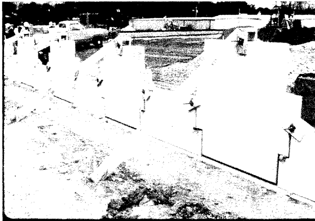
Figure 78. Setting first row of precast facing elements.
