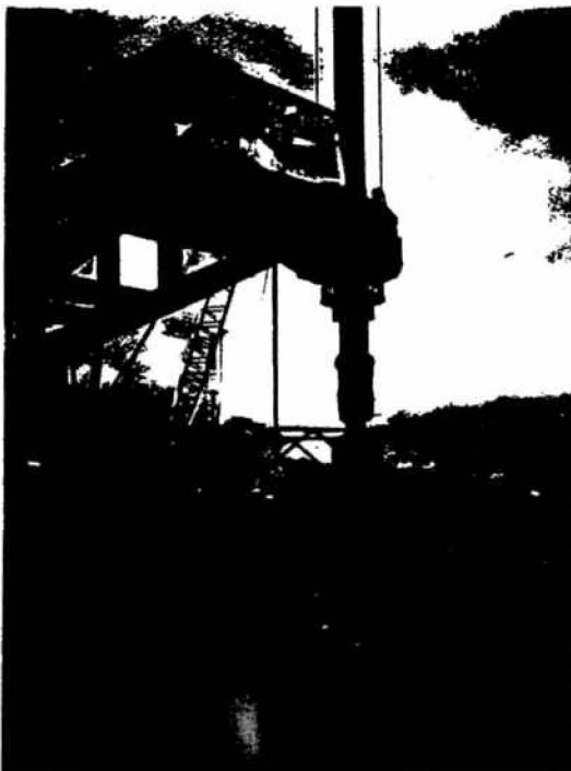
Left: Soil Mixing in progress at Ham Marine Facility in Pascagoula, MS.
