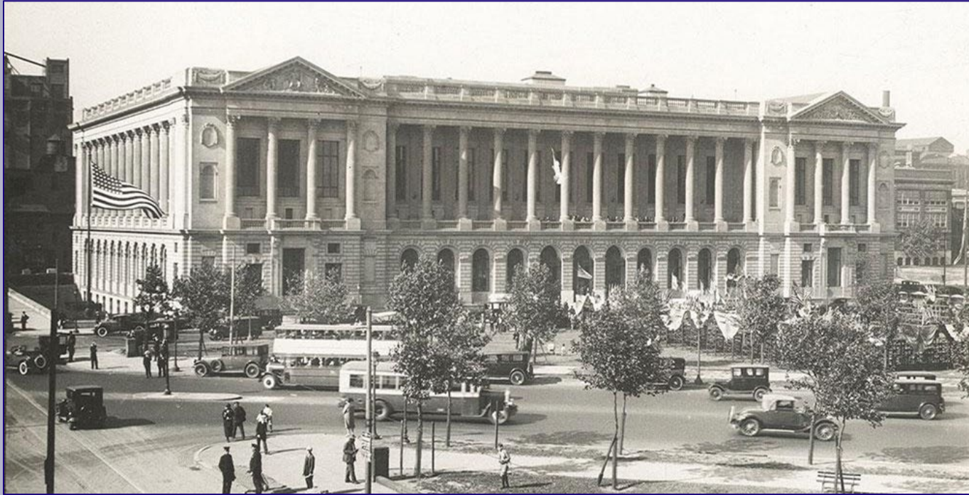
Parkway Central Library on Opening Day June 2, 1927
