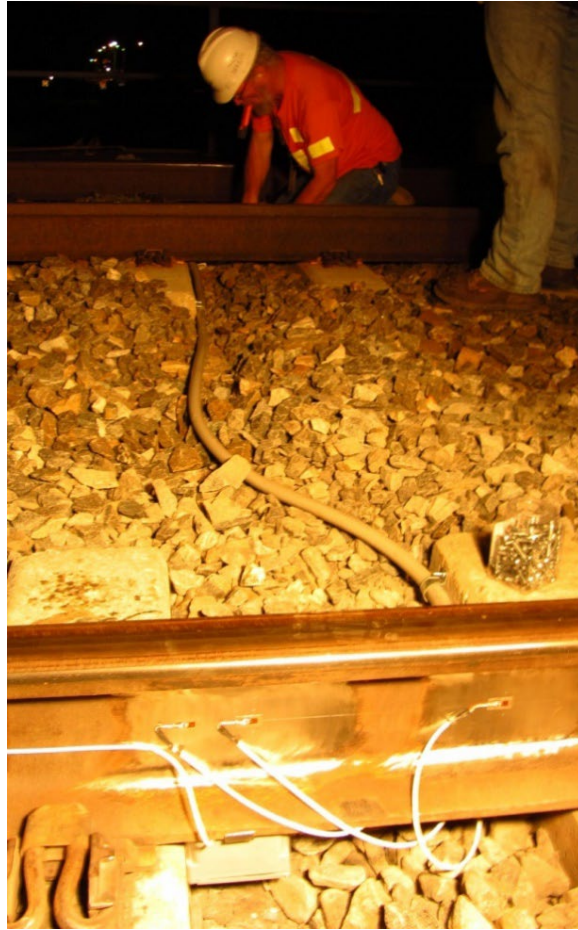
Figure 3.27: Installing Cable Duct Underneath Adjacent Tracks
