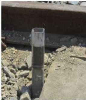
Figure 6.23: Different Steps Involved in the Stone-blowing Process
