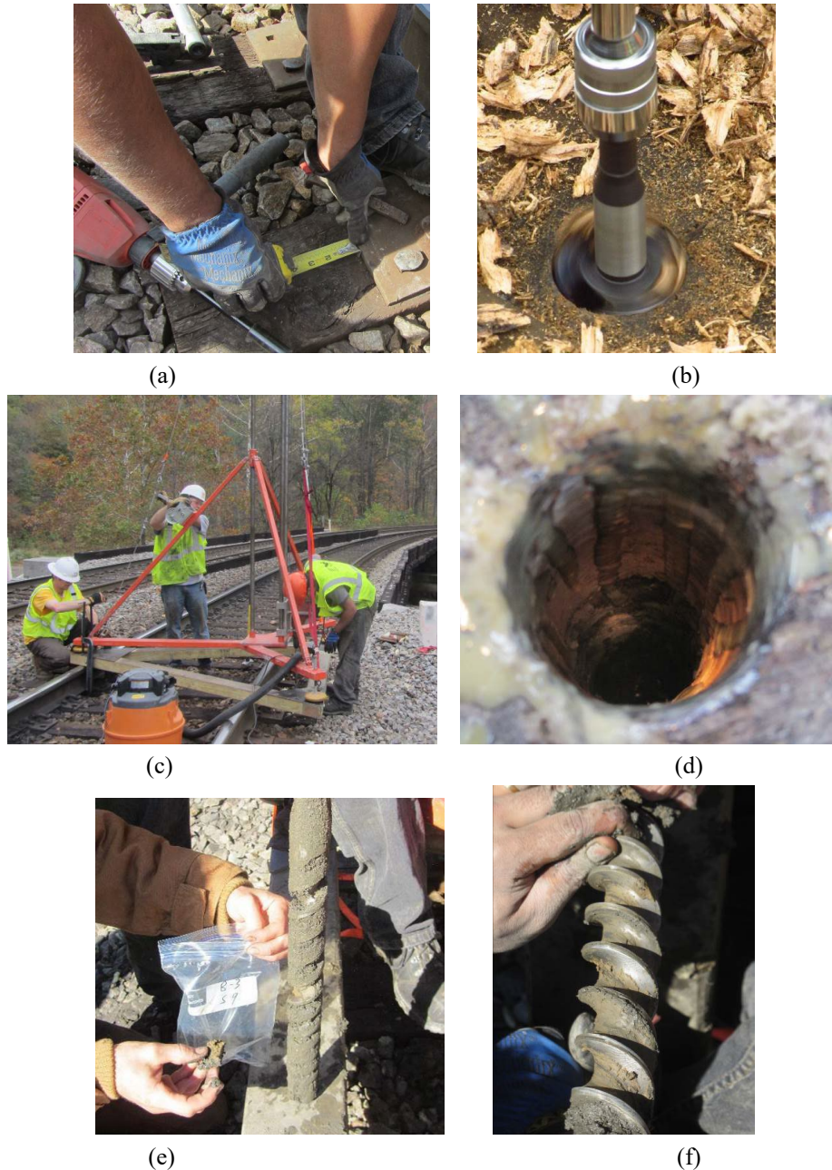
Figure 3.17: Photographs Showing Different Stages of Drilling for MDD Installation
