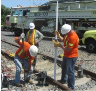
Surveying of Track to Establish Top-of-Rail Profile
