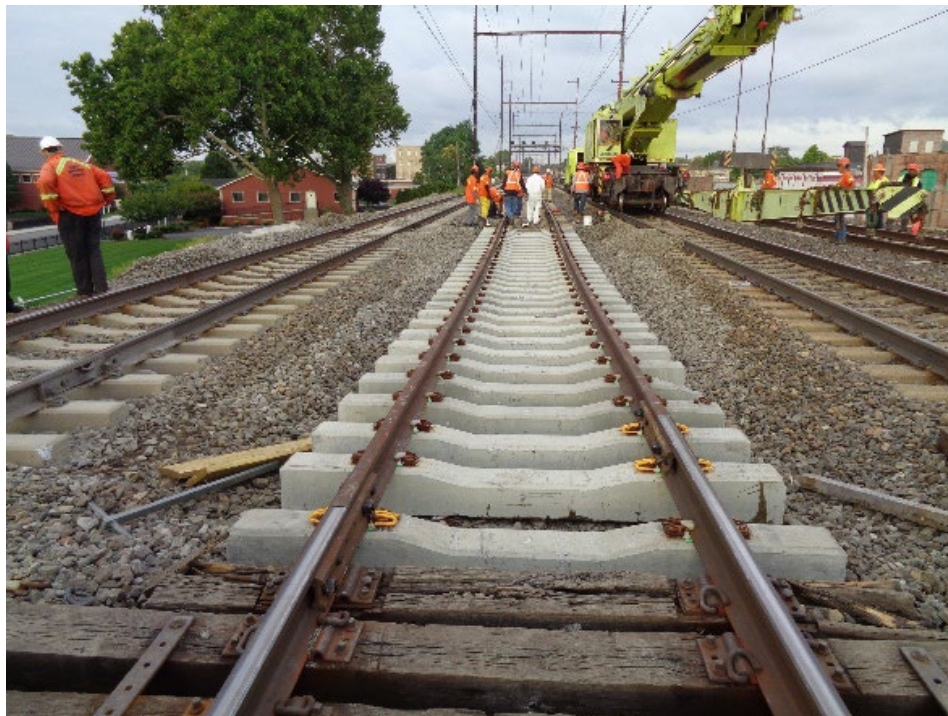
Figure 6.37: Final View of the New Tie Panel After Installation
