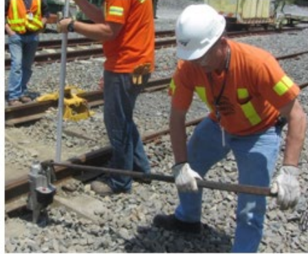
Jacking of Track to Pre-Determined Level
