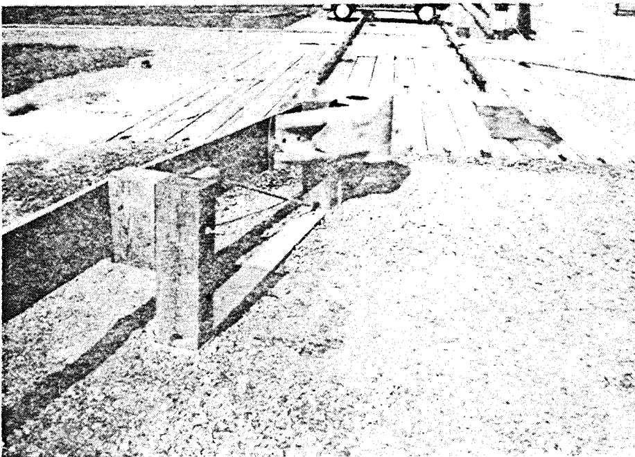
Figure 7. Modified eccentric loader breakaway cable terminal (MELT).
