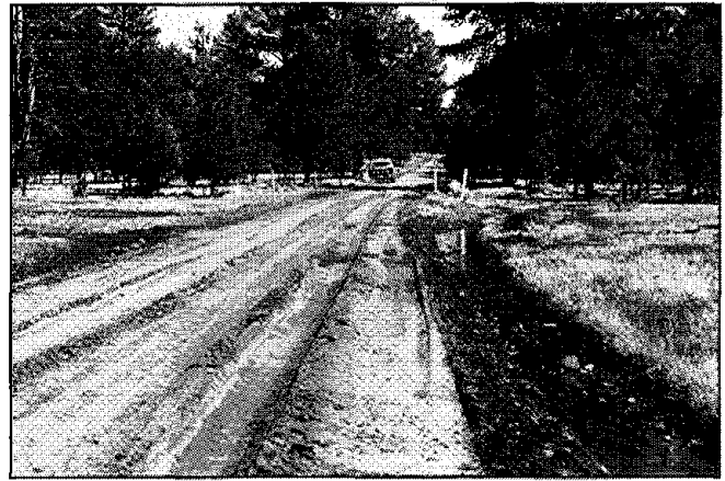
Figure 23. An in-meadow roadside ditch intercepts surface and subsurface flows.
