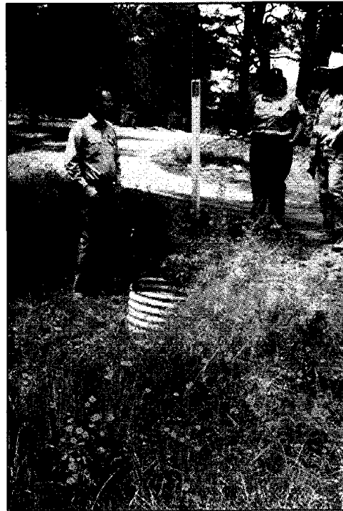
Figure 52. This right-angle elbow has been free from any problems associated with either piping or debris clogging for 7 years since installation, Forest Road 480, Cibola National Forest.
