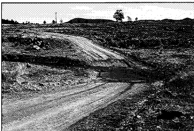
Figure 18. An unimproved ford at "S.A." Creek, near Luna, New Mexico, lowered the nickpoint, initiating headcutting in the upstream meadow.
