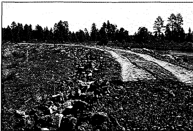
Figure 43. A permeable rock fill embankment under construction. Note placement of rock fill, separation fabric and embankment materials.
