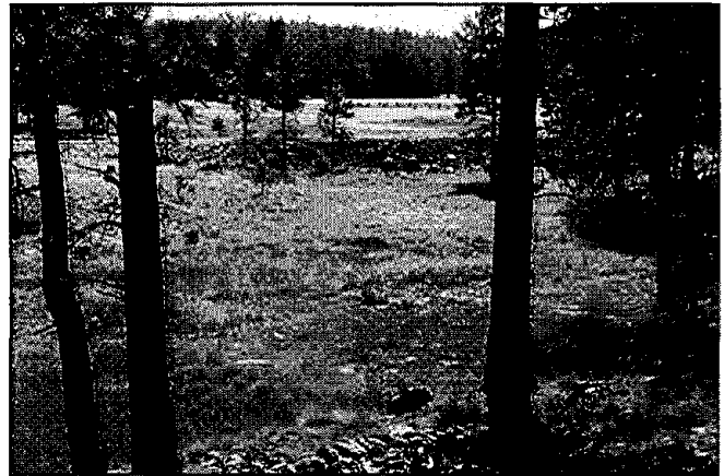
Figure 36. Six years after installation of raised culverts, wet meadow vegetation is sustained by baseflow discharged from a treated wetland, Post Office Flat, Cibola National Forest.
