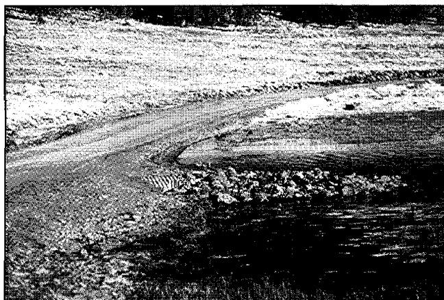
Figure 28. This encased rock berm was constructed by a volunteer youth group at Round Cienega, Apache-Sitgreaves National Forests.
