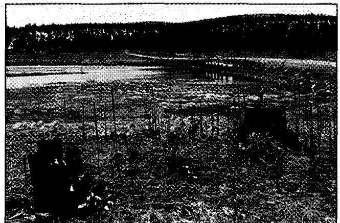
Figure 41. The road embankment serves as a dike at this raised culvert installation.
