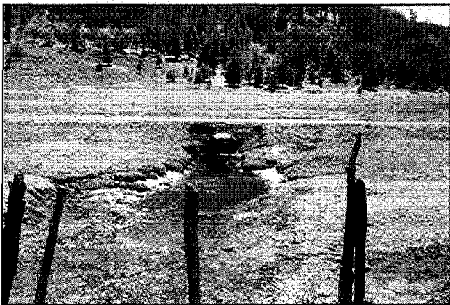
Figure 22. The combination of overgrazing and an overly deep culvert has caused erosion of this meadow.
