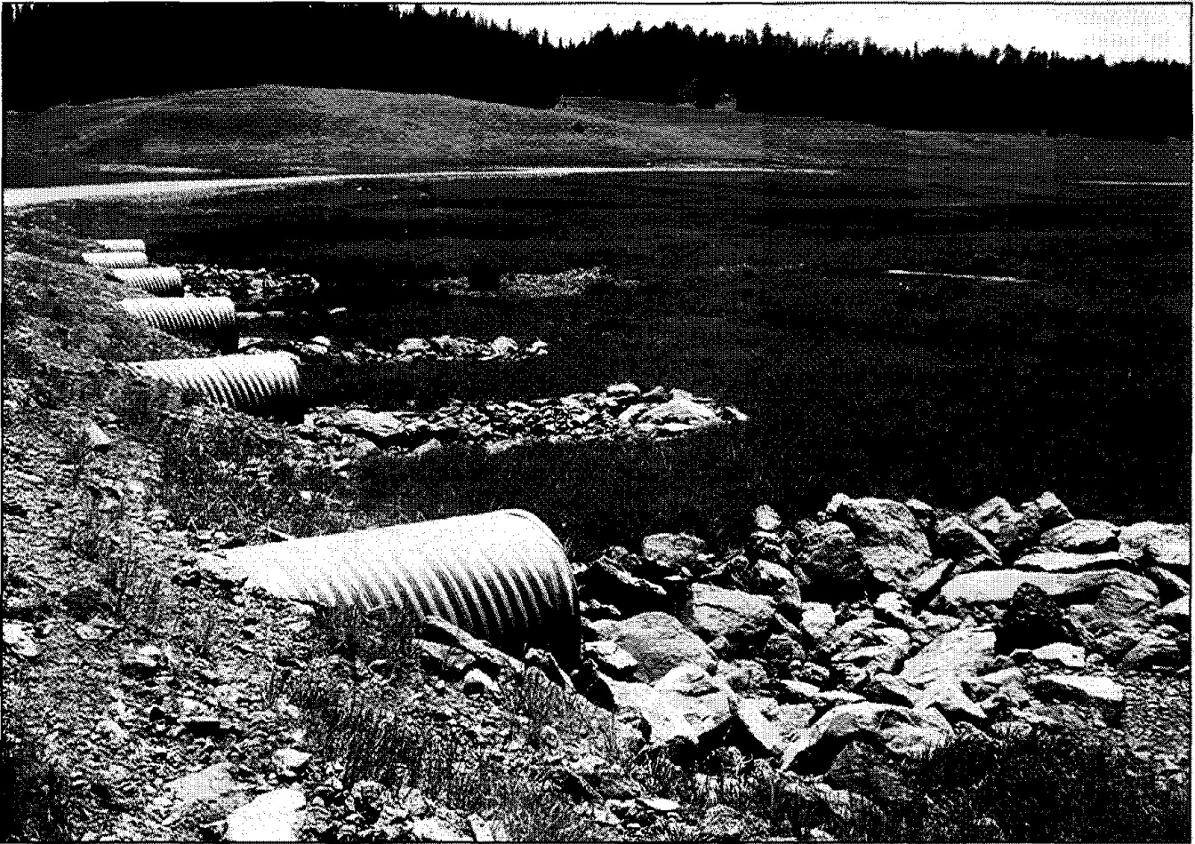
Figure 40. A multiple raised culvert complex 3 years after installation.
