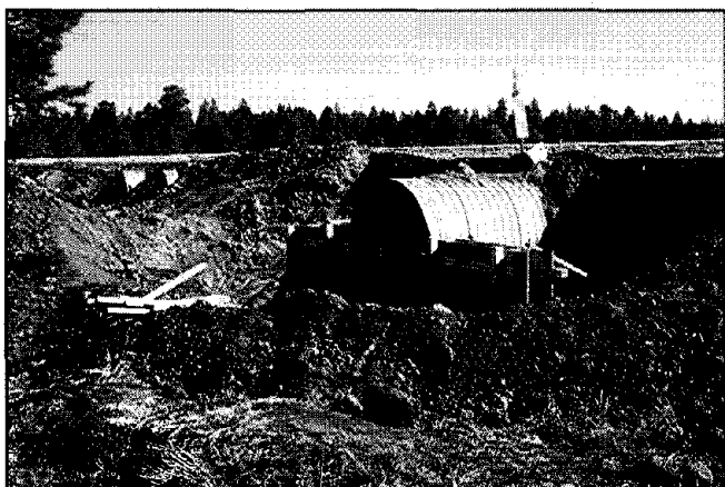
Figure 26. Construction of Forest Road 49, Cibola National Forest, provided an opportunity to install a reconstructed stream channel at Agua Fria Creek.
