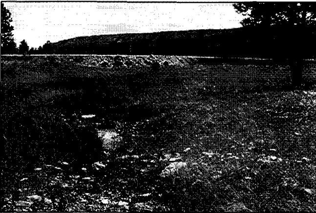
Figure 30. A wet meadow downstream from a raised culvert installed September 1992, Agua Media Creek, Cibola National Forest.
