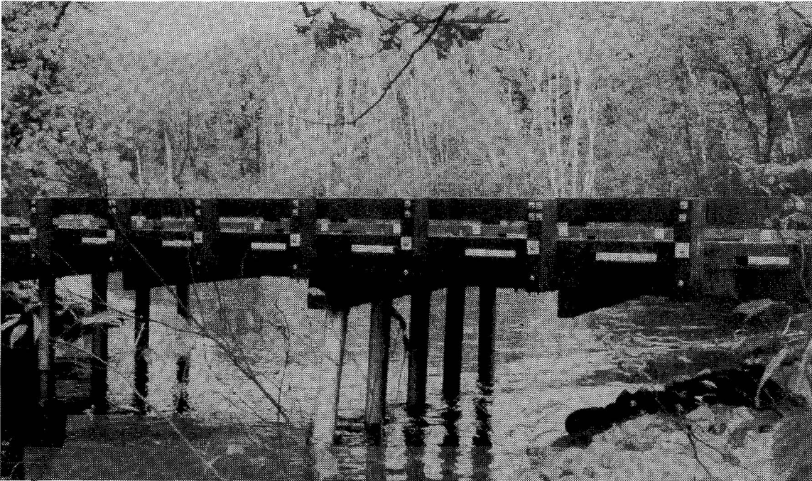
Figure 14. Glue-Laminated Wood Bridge (10).
