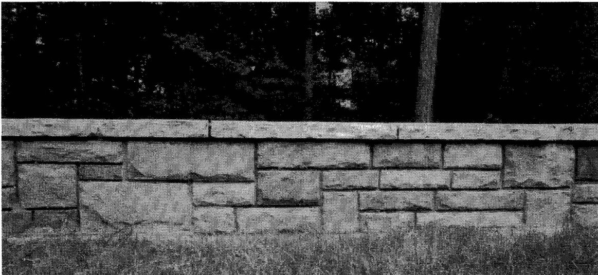
Figure 10. Pre-Cast Simulated Stone Guardwall -- Baltimore-Washington Parkway.
