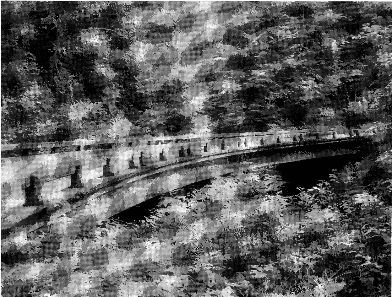
Figure 17. Federal Lands Highways Modified Kansas Corral Bridge Railing -- Olympic National Park.
