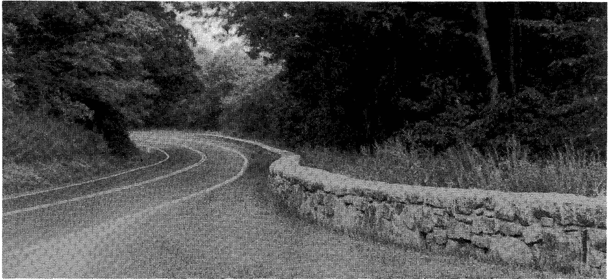
Figure 6. Stone Masonry Guardwall -- Skyline Drive, Virginia.
