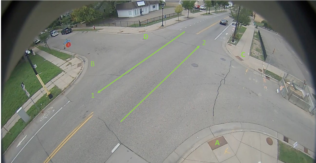
Figure B.16: Data collection site at N Upton Ave and Lowry Ave N, Minneapolis, MN.
