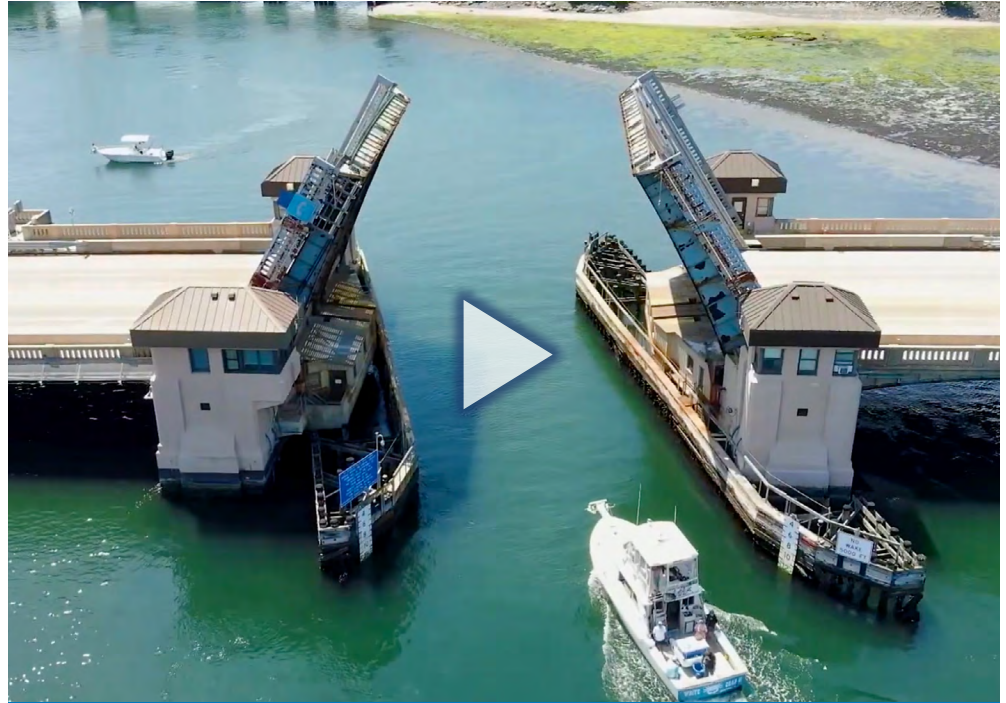
Watch a video to learn how the New Jersey DOT implemented a road diet that improved safety on an aging drawbridge.
