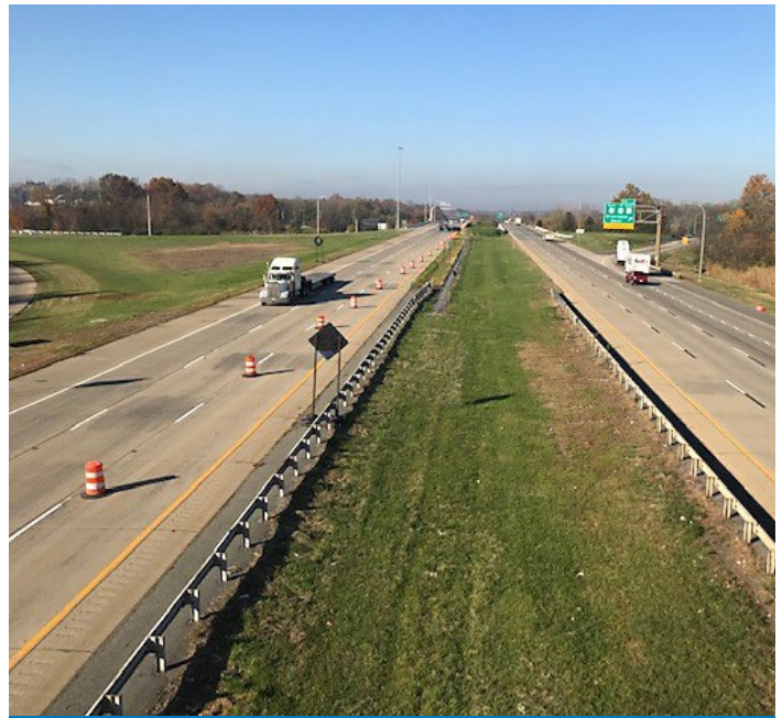
This concrete overlay on I-495 in Delaware was placed more than 30 years ago and still provides a smooth ride today.
