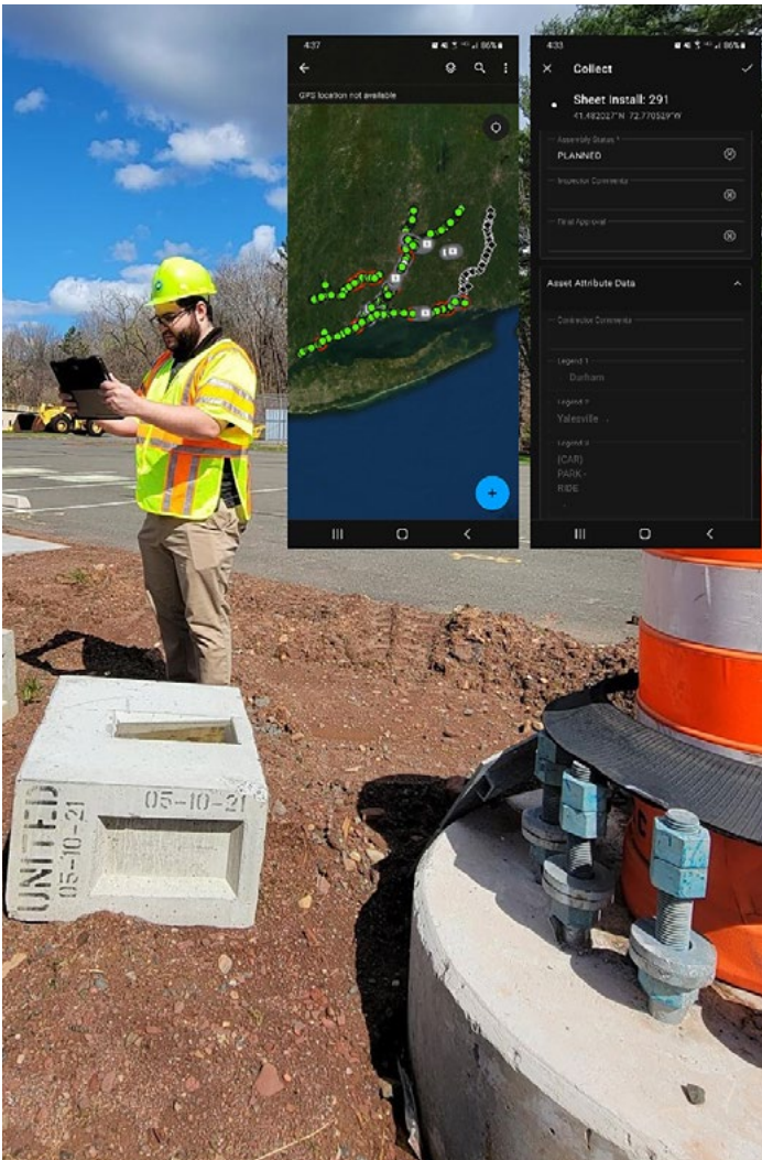
Connecticut DOT uses an app for collecting and updating sign data in the field.
